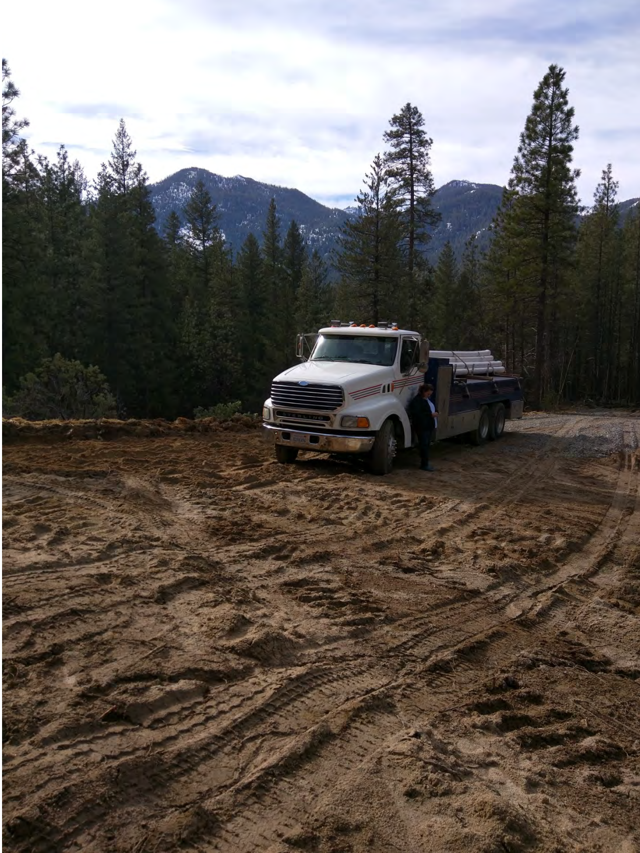
Photo 46: View looking west. New road construction begins and extends downhill on the right side of the photo
