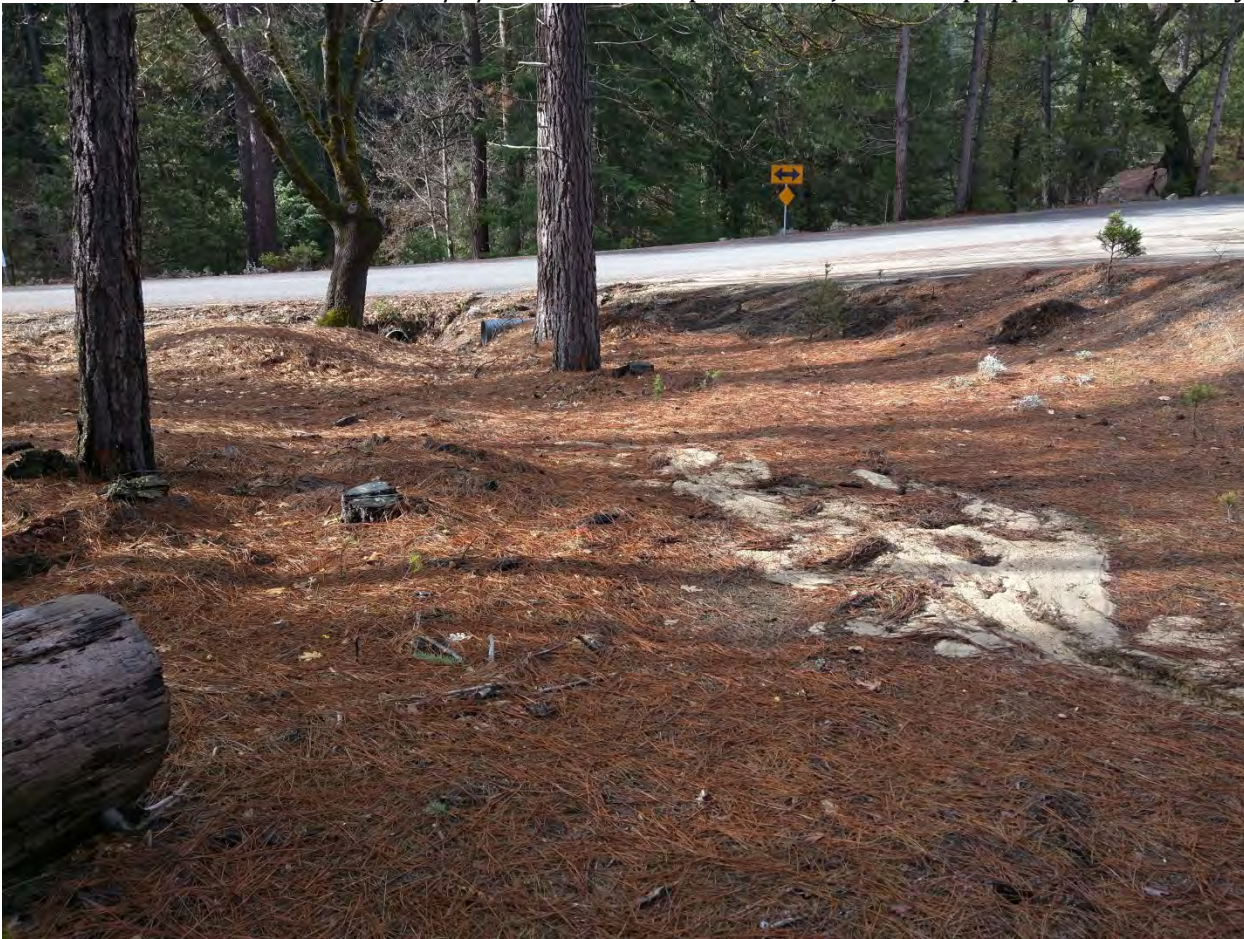
Photo 13: View looking west towards the upstream culvert that transfers flow from the ephemeral watercourse that drains the Western Clearing and discharges into French Creek approximately sixty feet below the downstream end of this culvert
