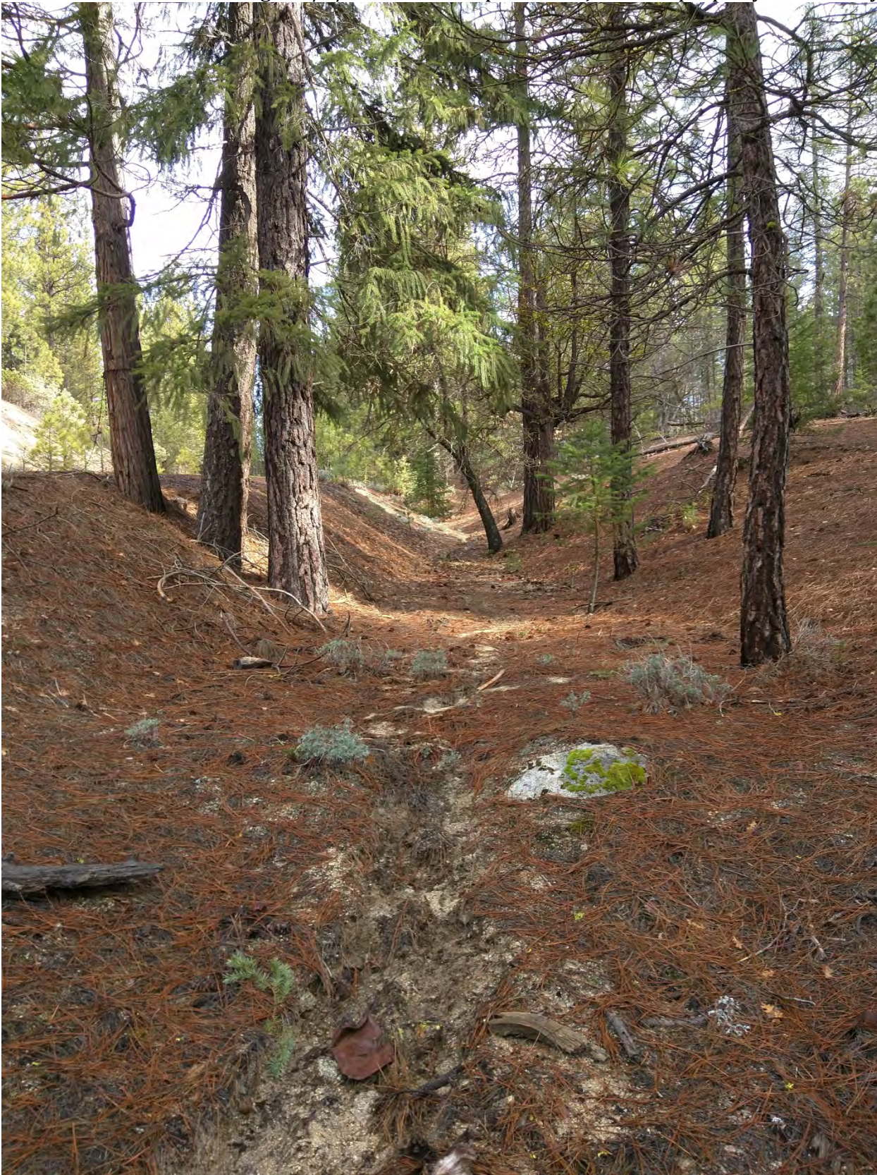
Photo 14: View looking east (upstream) towards the detention basin and the Western Clearing from the culvert crossing of the ephemeral watercourse under French Creek Road
