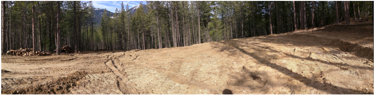
Photo 7: Panorama of the Eastern Clearing area, view to the north
