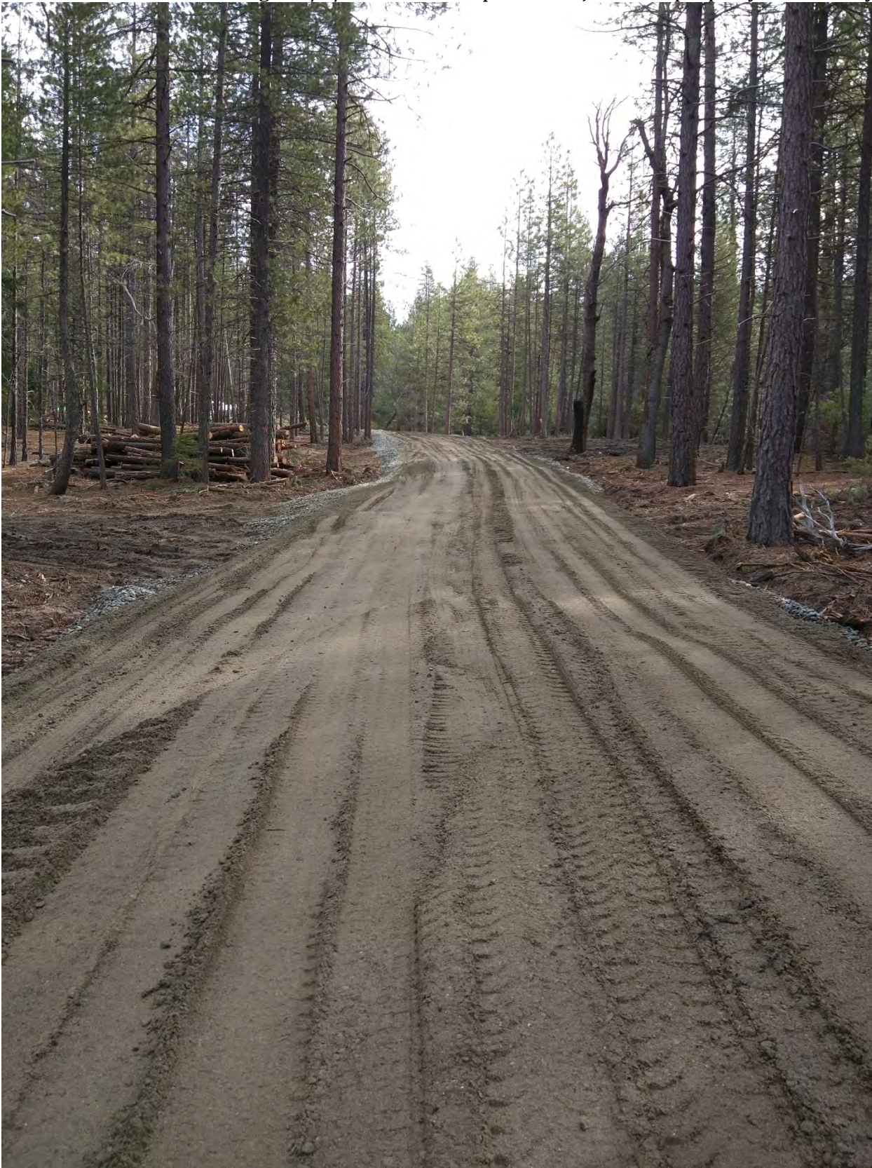
Photo 24: View looking east at the new road construction heading towards the Middle and Eastern Clearings
