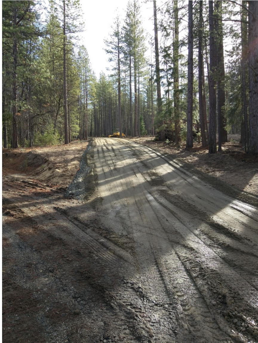
Photo 2: View looking east facing the new road construction at its junction with French Creek Court.
