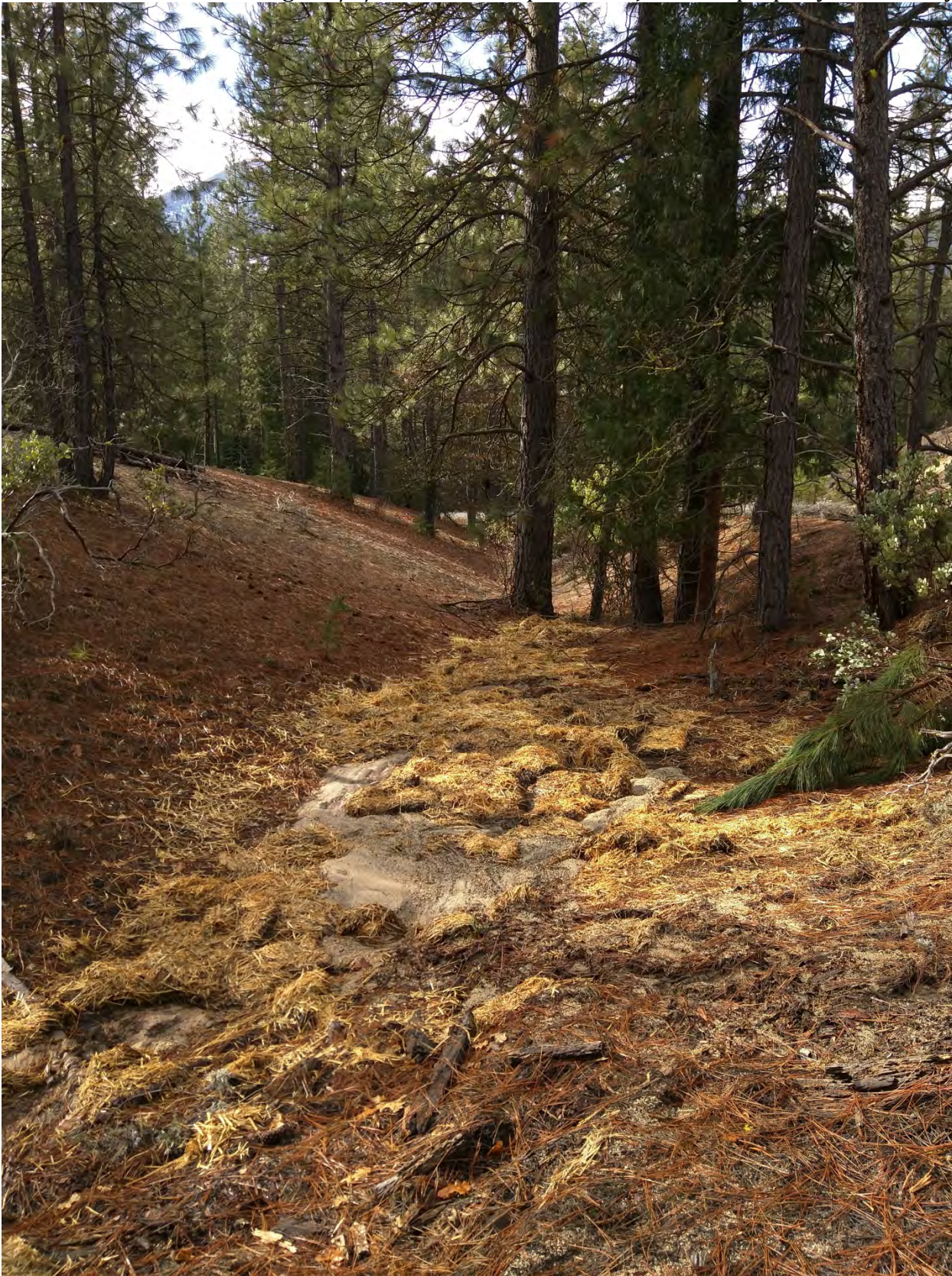
Photo 11: View looking downstream from the same location as Photo 10. Note deposited earthen material in the channel
