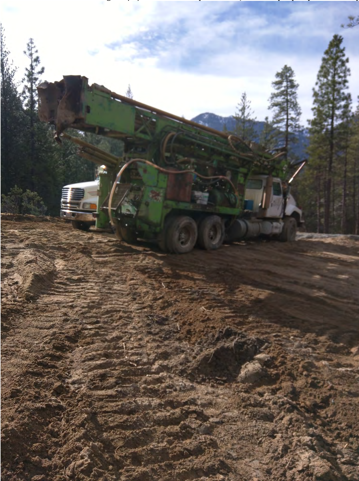
Photo 27: Well driller's equipment parked at the eastern terminus of the new road construction
