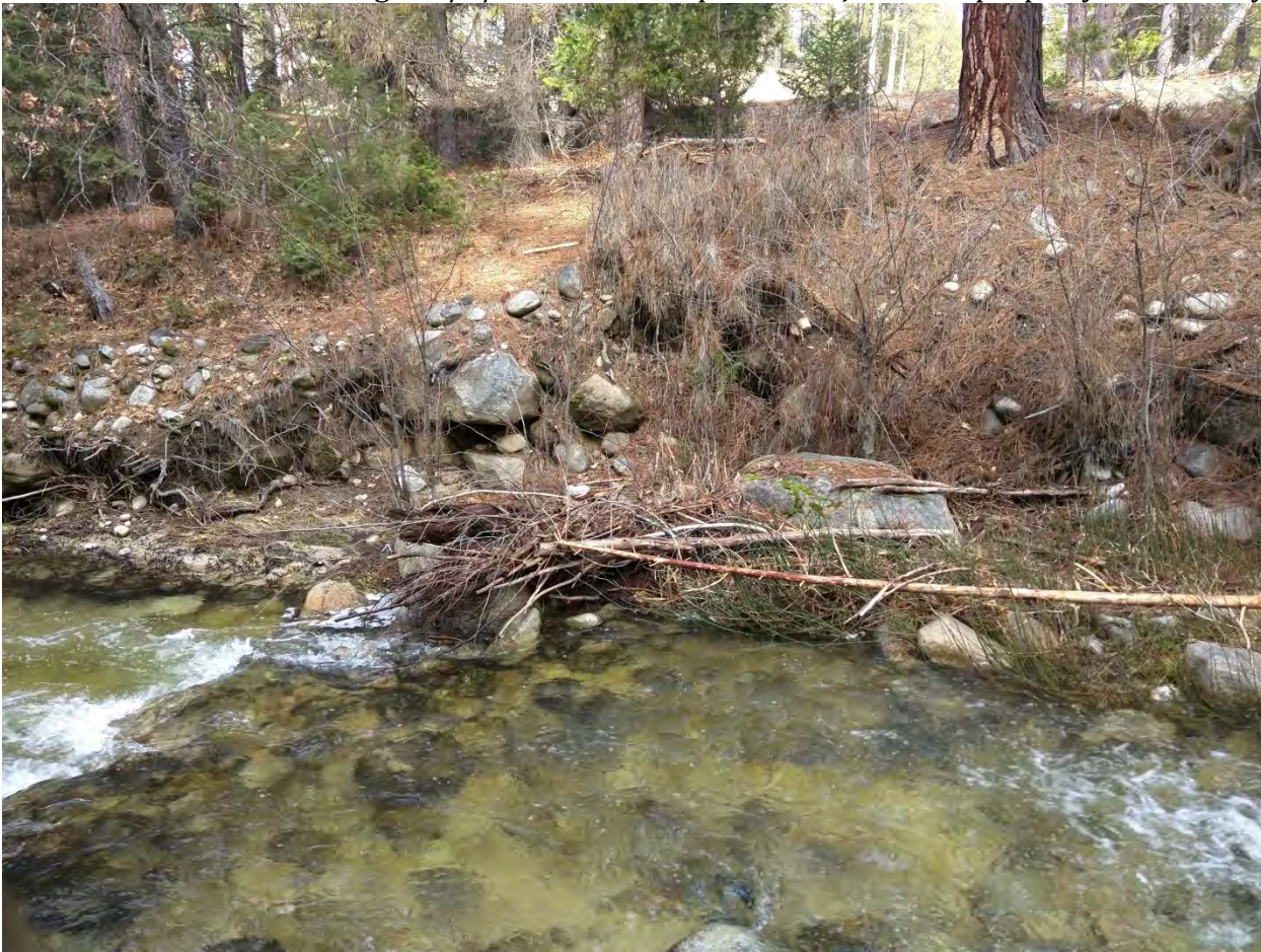
Photo 50: Another view across French Creek towards the culvert of the ephemeral watercourse associated with the complaint
