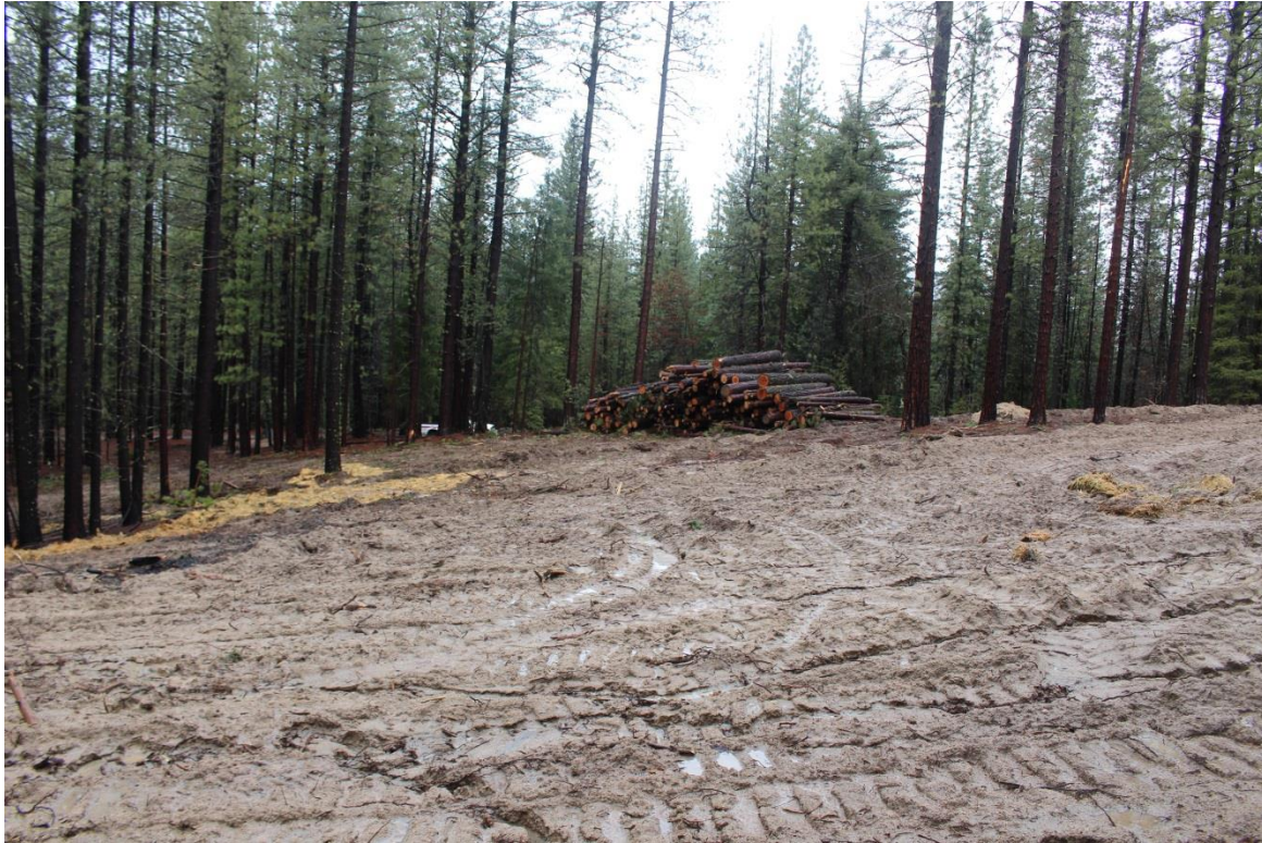
P17 1/29/2016 10:57 AM Looking north at converted area and log deck.
