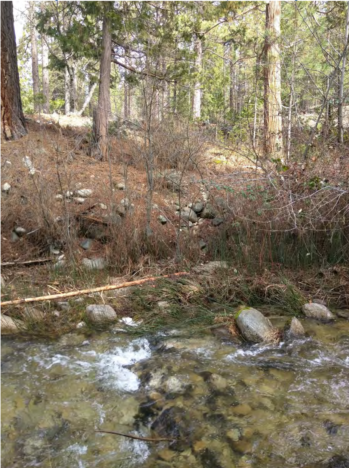
Photo 49: View to the east across French Creek looking at the outboard edge of French Creek Road and the culvert crossing of the Ephemeral Channel identified in earlier photos
