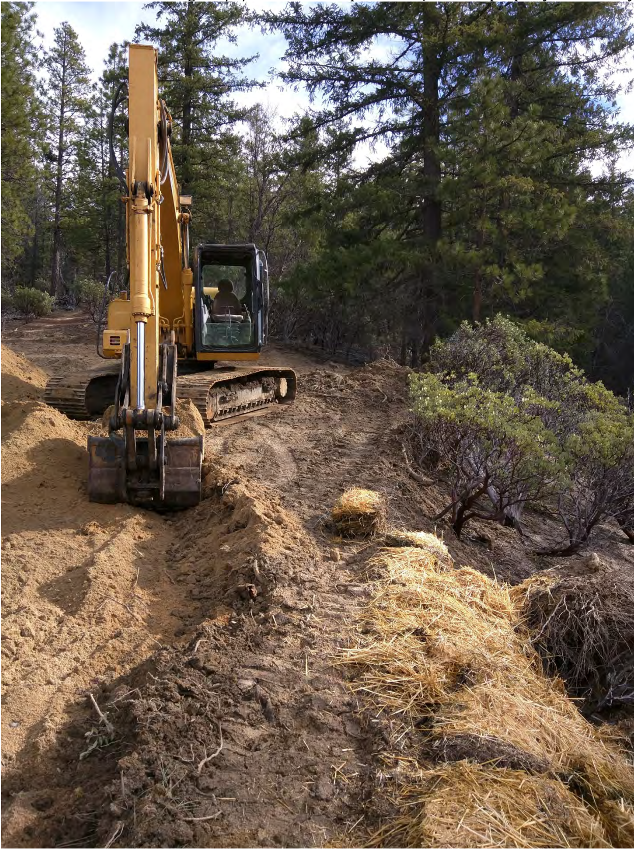
Photo 48: Another view of the excavator
