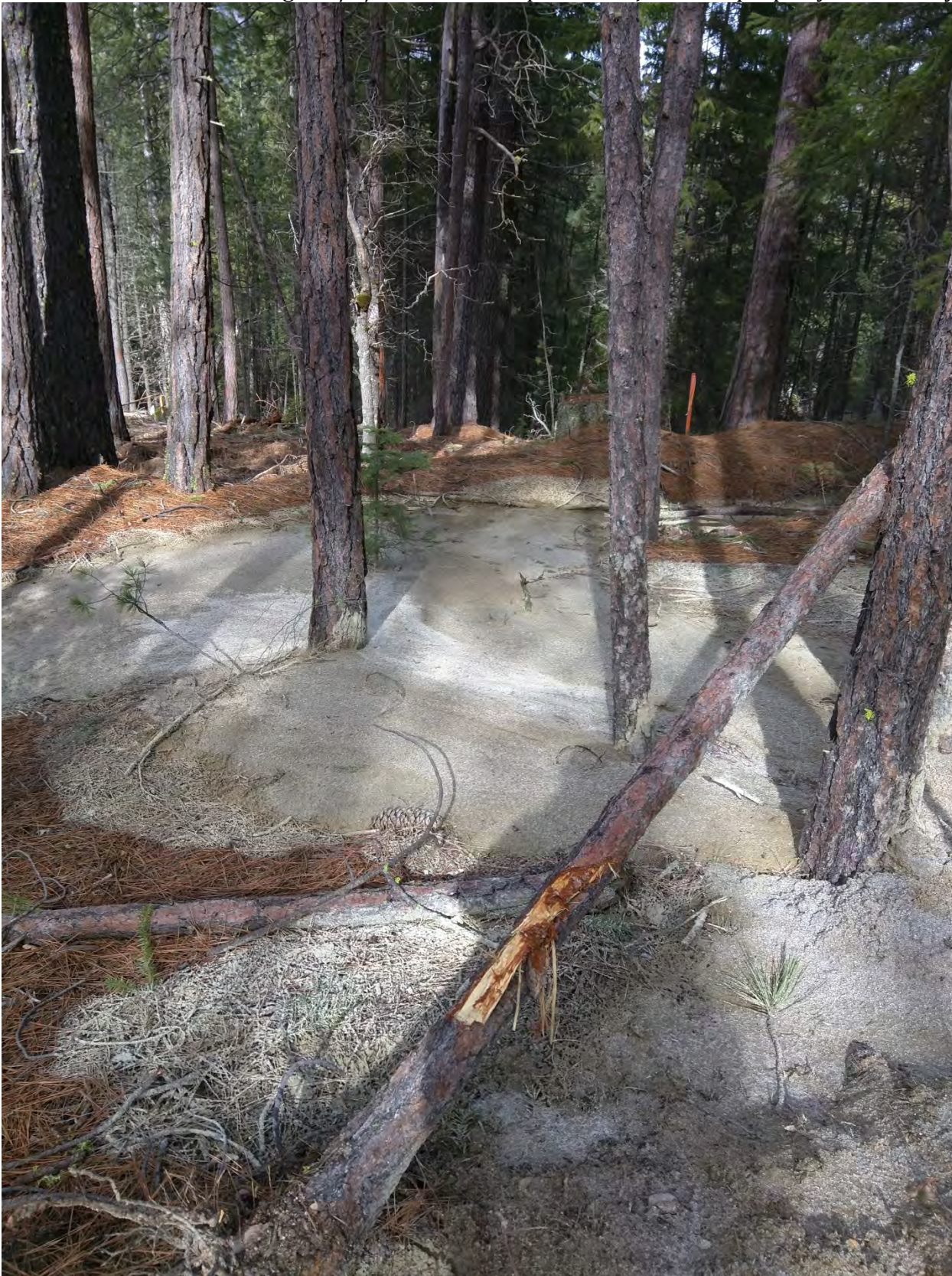
Photo 42: New well installation just east of the main Eastern Clearing. Note evidence of recent movement of earthen material
