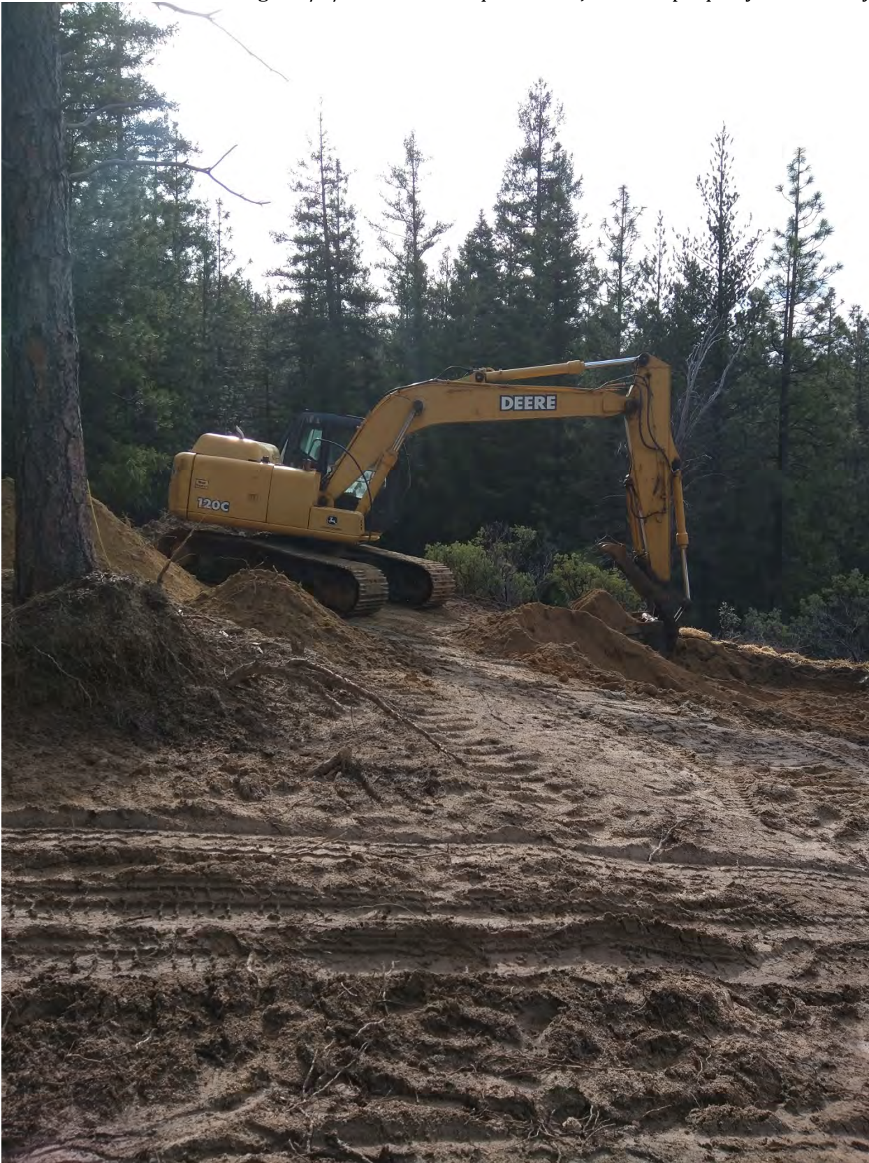
Photo 45: Excavator parked near the well driller's equipment
