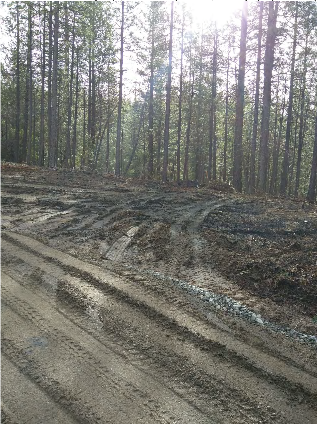
Photo 25: Vehicle turnaround area off of the new road construction.
