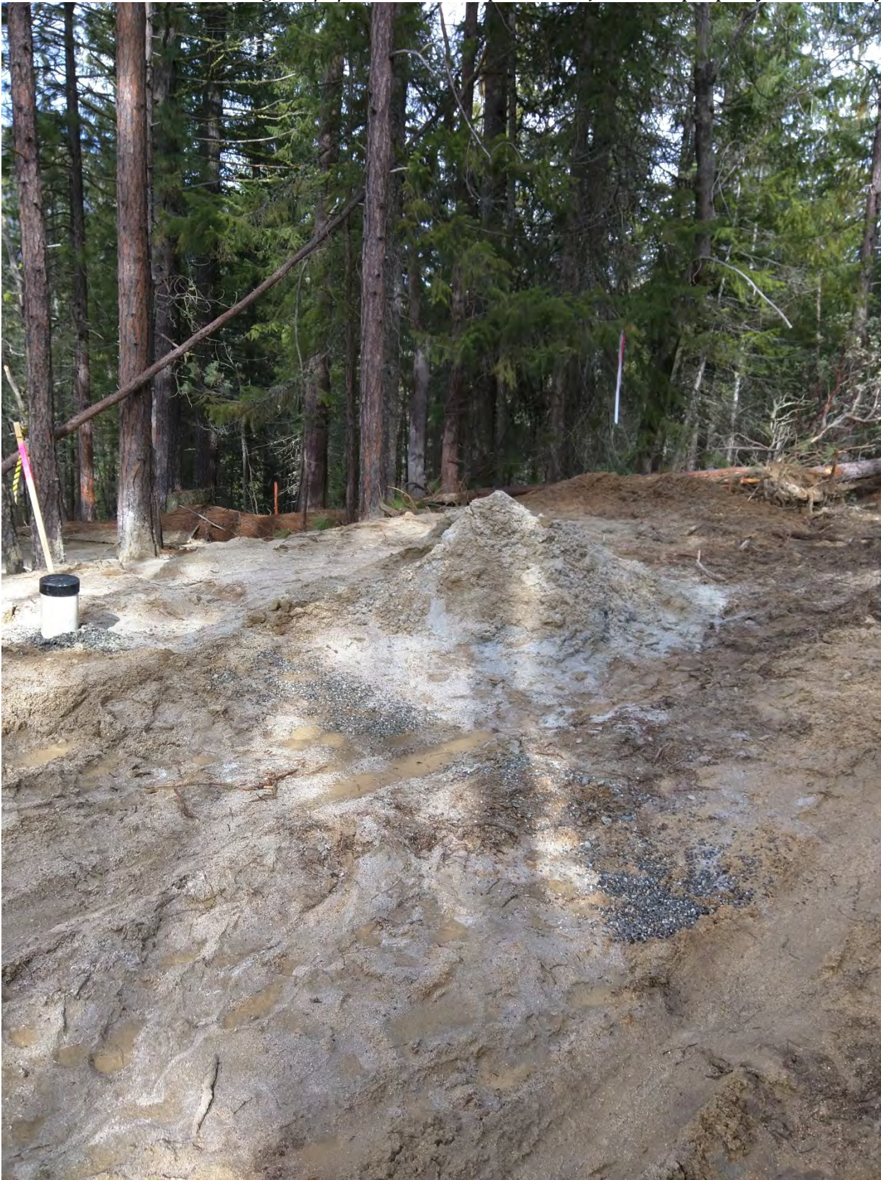
Photo 40: New well installation just east of the main Eastern Clearing
