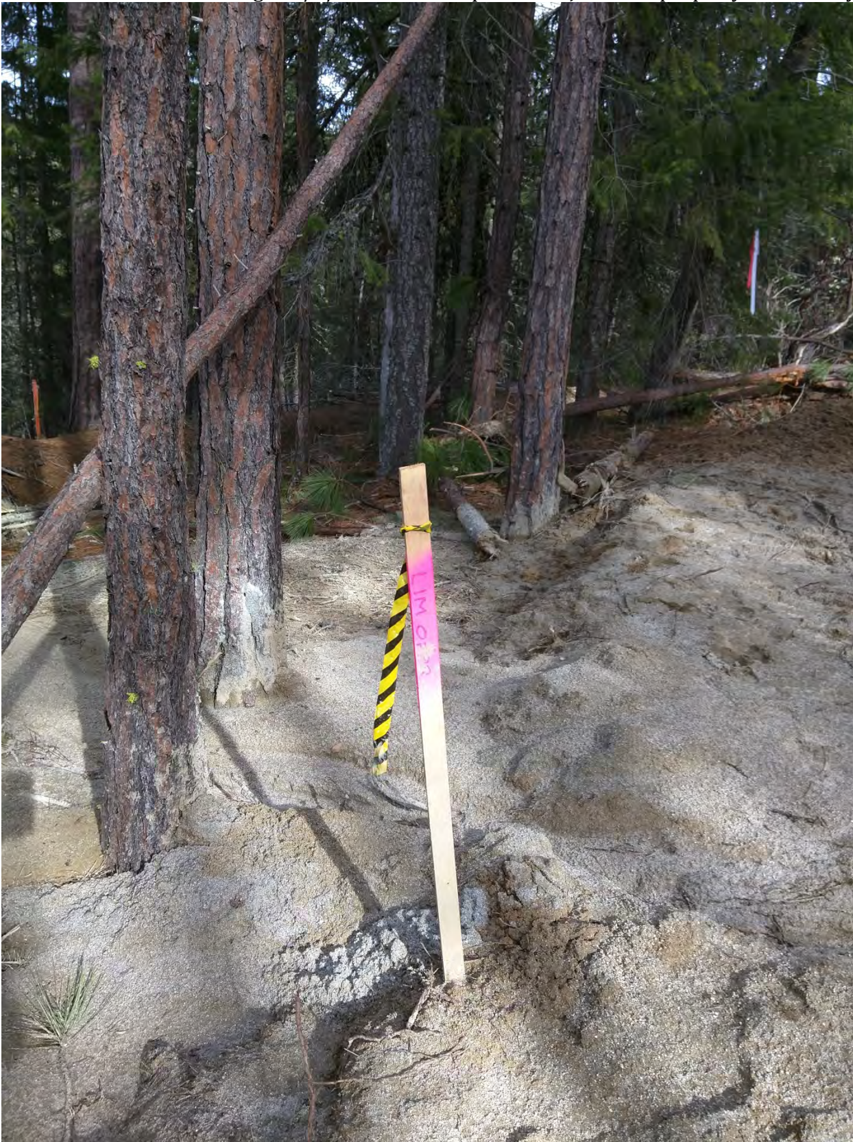
Photo 41: New well installation just east of the main Eastern Clearing
