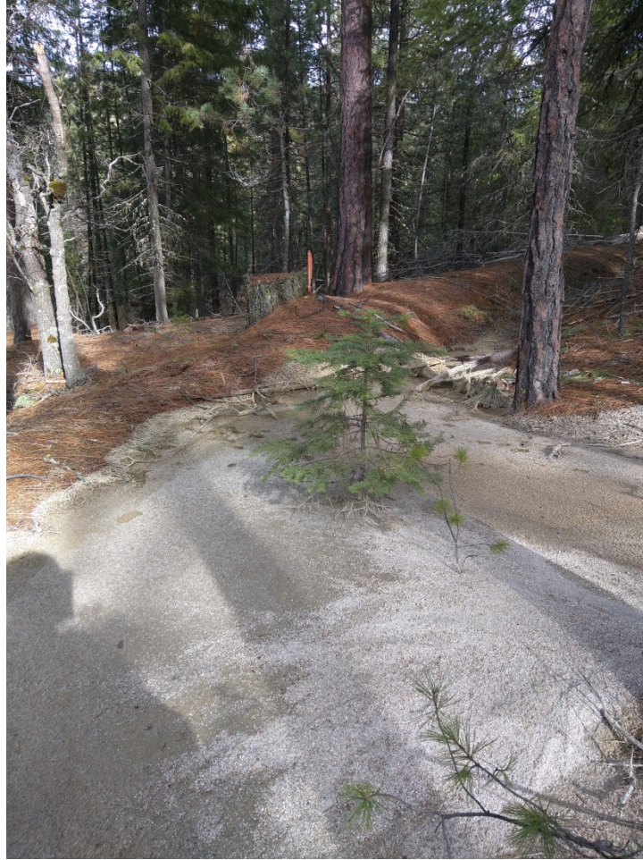
Photo 9: Earthen material adjacent to water well construction
