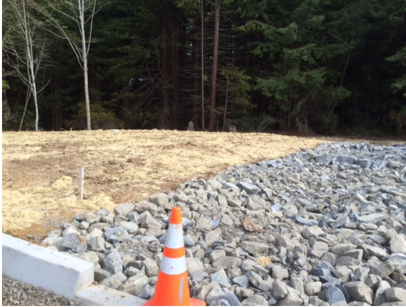
Photograph 1. Armoring of active drainageway
