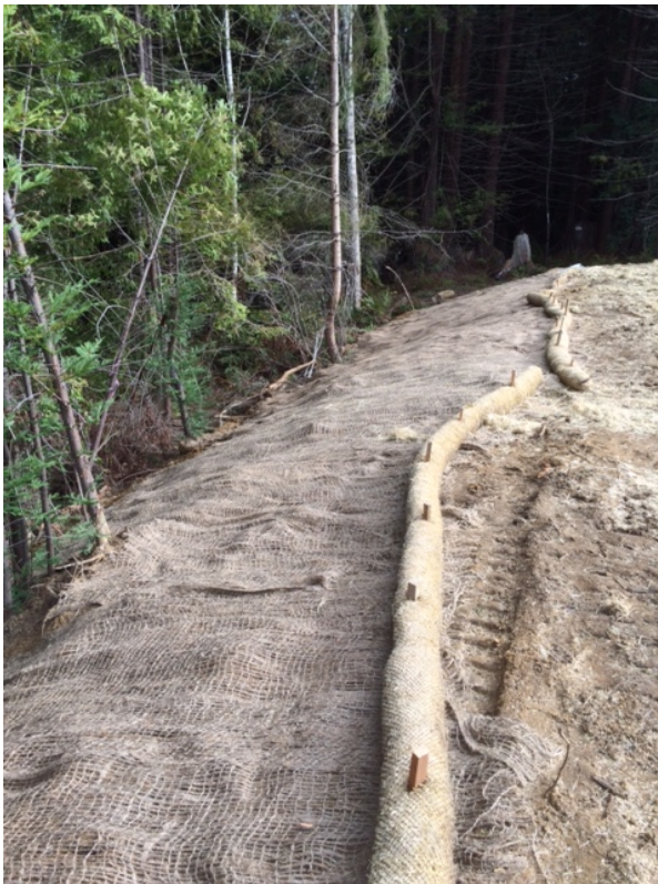
Photograph 2. Re-grading and covering fill-slopes
