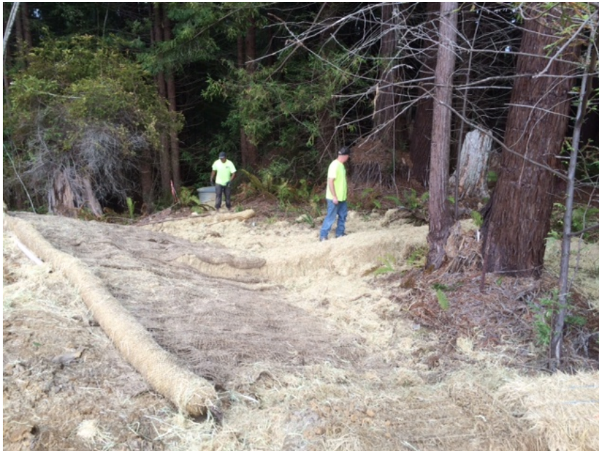
Photograph 4. Repairing downslope areas adjacent to tributary creek
