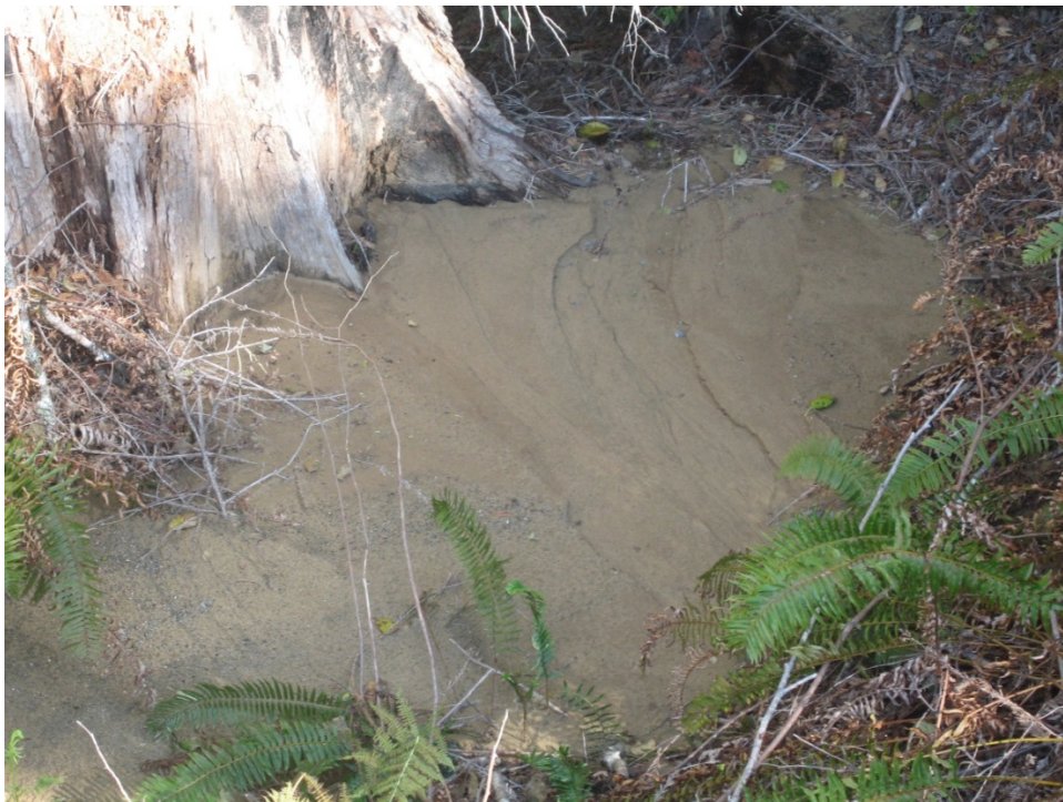
Photograph 4. Mary Court Subdivision –11/02/16: Offsite discharge of sediments adjacent to bank of tributary drainage. Photograph by Paul Keiran, Regional Water Board staff
