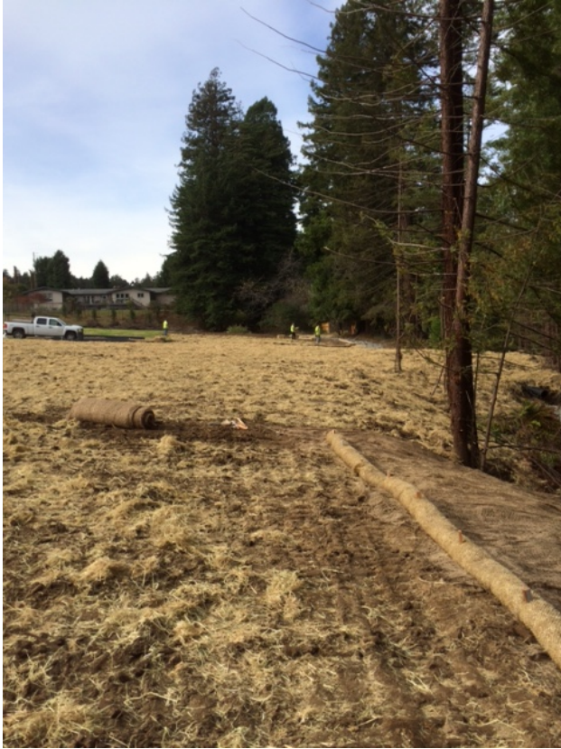
Photograph 3. Straw ground cover and wattle placement
