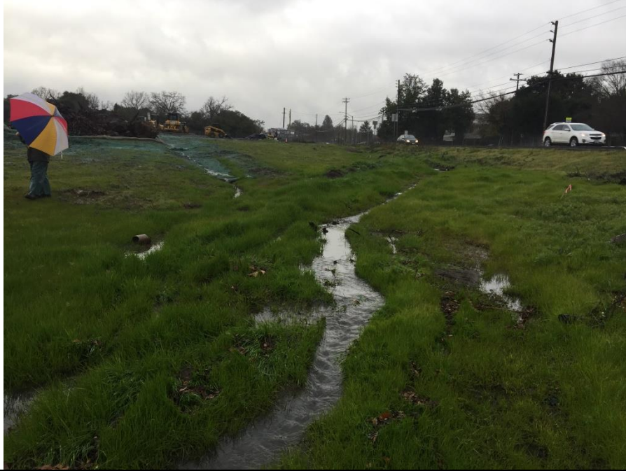
Photo 17: Looking north on the southeast portion of the Project site. Run-on from Fulton Rd. cross-culvert shown coming from the right side of photo to the foreground. A confluence with the drainage from the equipment staging area is in the lower left corner of the photo.
