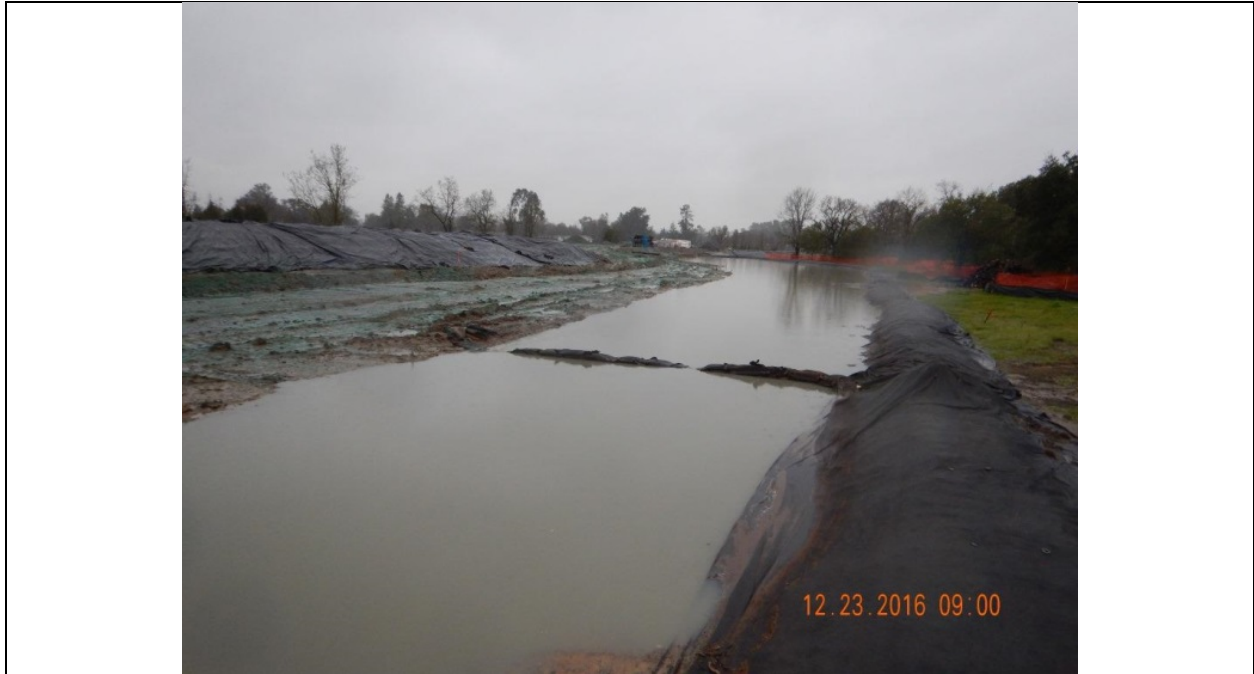
Photo 7: Another earthen berm covered with filter fabric, looking south. Peterson Creek is approximately 60-70 feet to the right.
