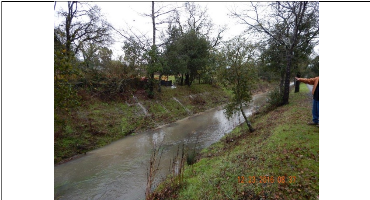
Photo 3: Peterson Creek discharge location 2. This discharge location appears to correspond with discharge sampling location #5 as provided in the 12/23/16 Sampling Field Log sheet. As shown in Photo 4, storm water was either passing beneath the silt fence or infiltrating and discharging at a uniform elevation on the bank of Peterson Creek. Storm water may have infiltrated and forced to emerge from the bank after hitting an impervious soil layer.
