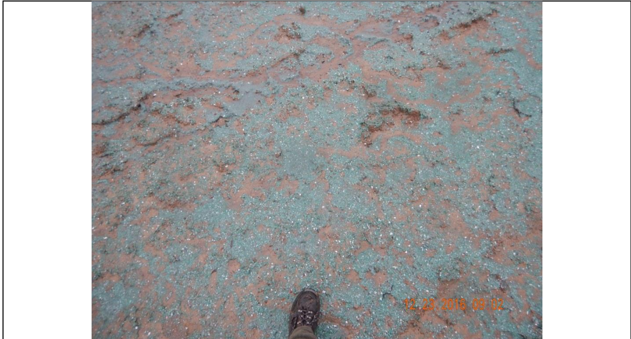
Photo 11: Close-up of area shown in Photo 10. Mr. Fortney said the hydromulch was sprayed at 1,500 pounds per acre.
