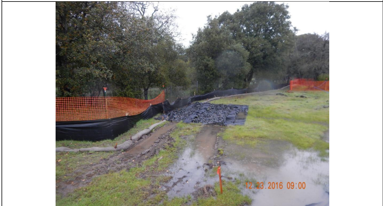
Photo 8: An armored discharge point along the western project boundary, in the northwest corner. There was no discharge to Peterson Creek occurring at the time of our visit.
