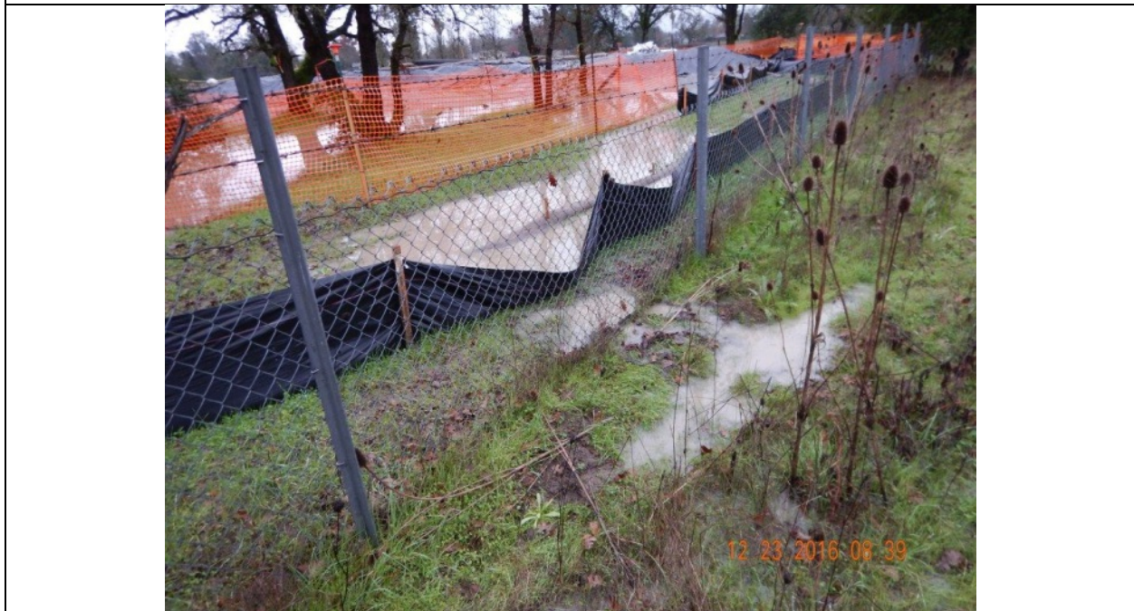
Photo 2: Peterson Creek discharge location 1. It appeared that storm water was passing underneath the silt fence. This discharge location appears to correspond with discharge sampling location #1 as provided in the 12/23/16 Sampling Field Log sheet.
