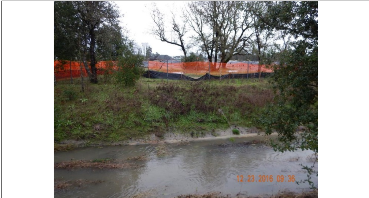
Photo 1: Peterson Creek discharge location 1. Photo was taken at 8:36 a.m. The camera time stamp was corrected after this photo was taken. Water was running down the stream bank and causing turbidity along the left bank channel margin as shown in the photo.
