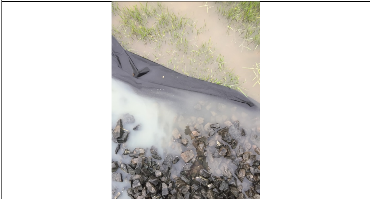
Photo 16. Photo taken within the eastern catchment. The storm water runoff on the bottom half of the photo is from areas treated with hydraulic mulch and has a green hue, unlike the water in the top of the photo, which is from areas largely not treated with hydraulic mulch. Ponded water throughout the Project area, in areas where hydromulch had been applied, had a green hue.
