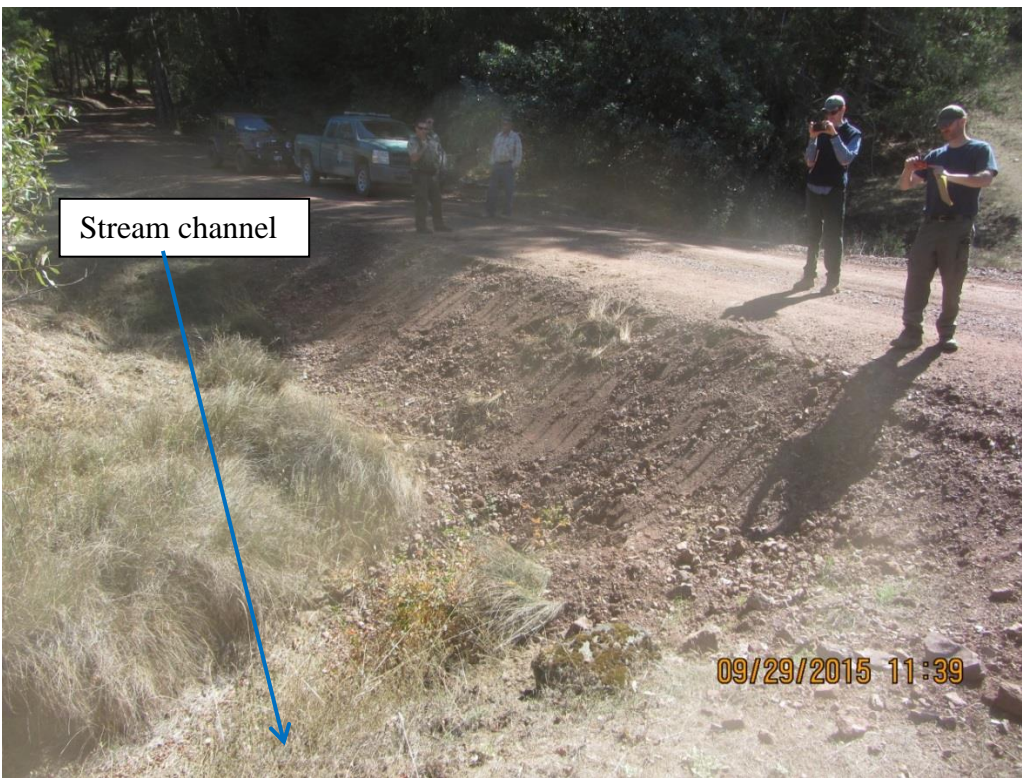
Image 17 shows the upstream east side of the filled stream channel at GPS 5. (IMG 0263)
