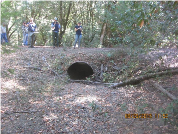
Image 22- upstream of the culvert at crossing 5 (GPS 7) looking downstream at the mouth of the culvert. Note the width of the stream channel as compared with the diameter of the culvert inlet. (IMG 0266)
