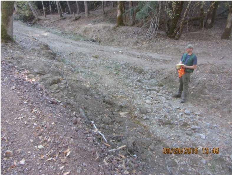
Image 40 shows the secondary road in the stream channel and the road fill in and adjacent to the upstream channel placed during the recent road construction at GPS 14. (IMG 0321).
