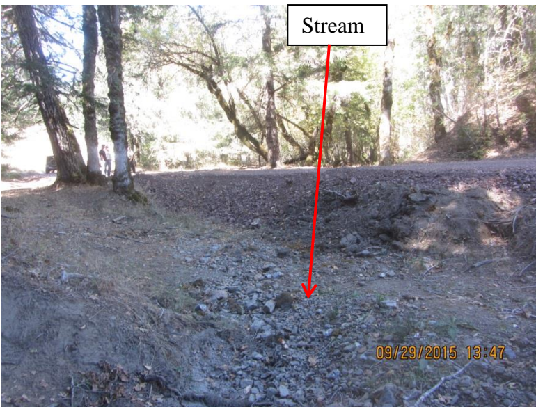
Image 41 shows the road fills in the stream looking upstream at the crossing at GPS 14. (IMG 0323).
