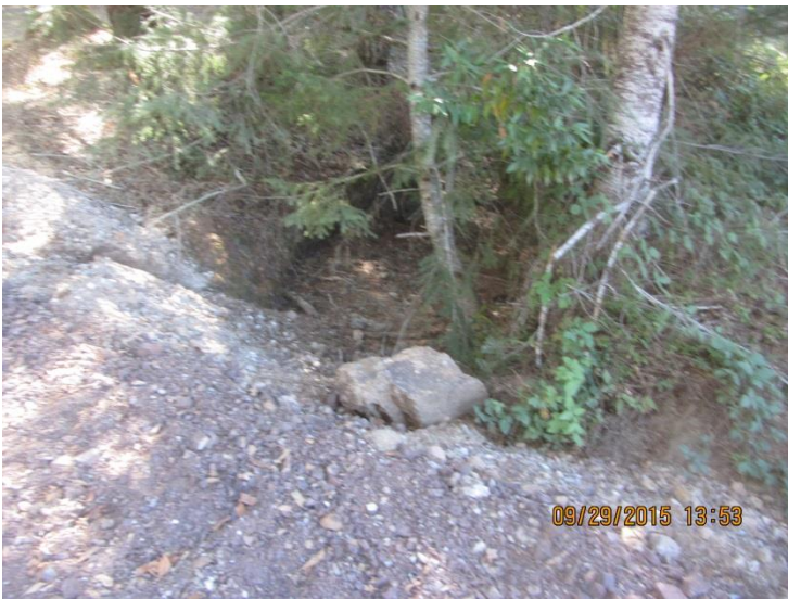
Image 43 shows the upstream channel as it reaches the earthen fills in the road at GPS 15. (IMG 0326)
