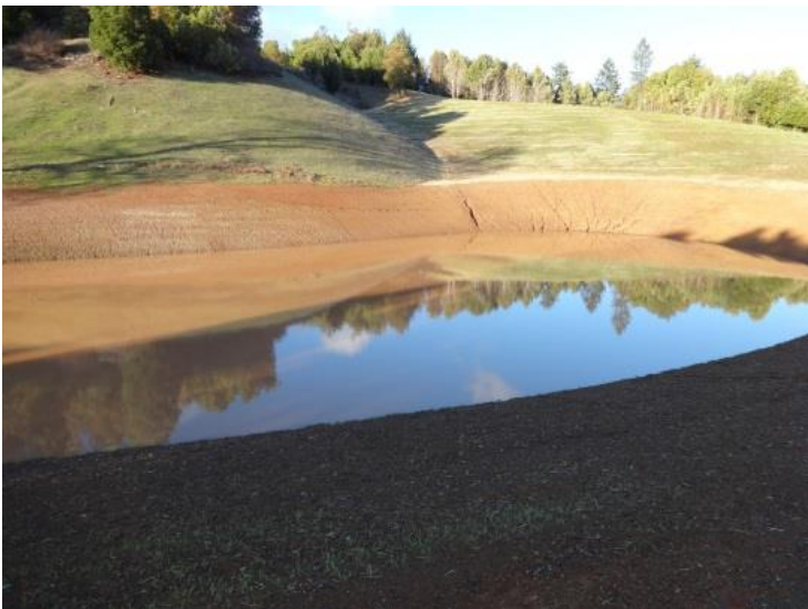
Image 45 shows the new pond now partially filled with water. (Brandon Rose, photo146).
