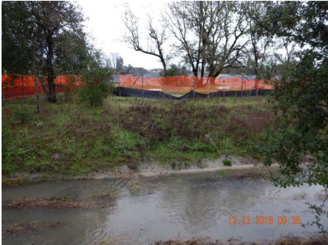
Photo 29. Peterson Creek discharge location 1. Photo was taken at 8:36 a.m. The camera time stamp was corrected after this photo was taken. Water was running down the stream bank and causing turbidity along the left bank channel margin as shown in the photo.
