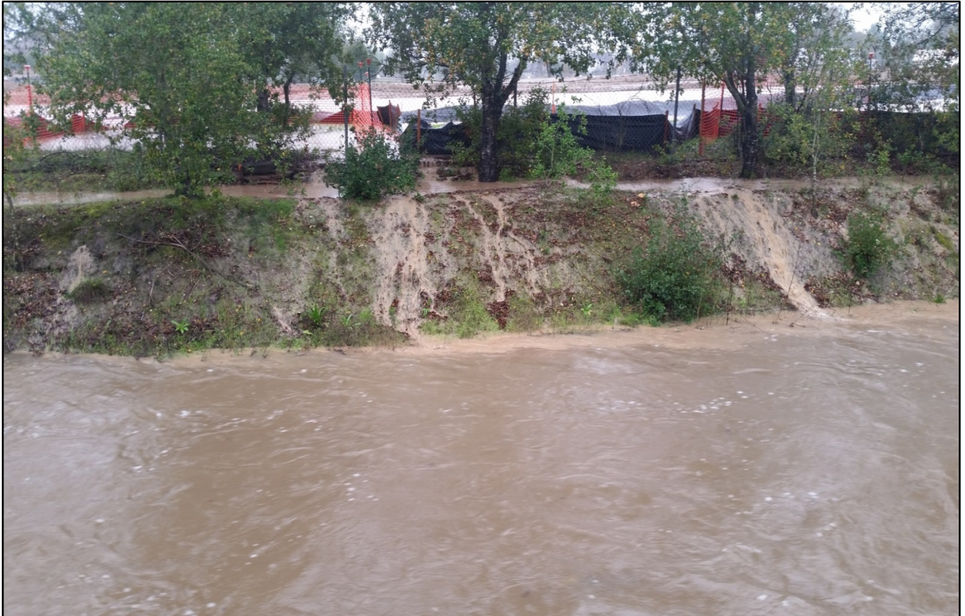
Photo 14. Sediment-laden storm water runoff discharged from the Site along the western boundary and into Peterson Creek. The containment area was overwhelmed by the volume of water, causing it to flow over the berm and over the silt fences and into the creek. Photo was taken facing southeast at 13:25.
