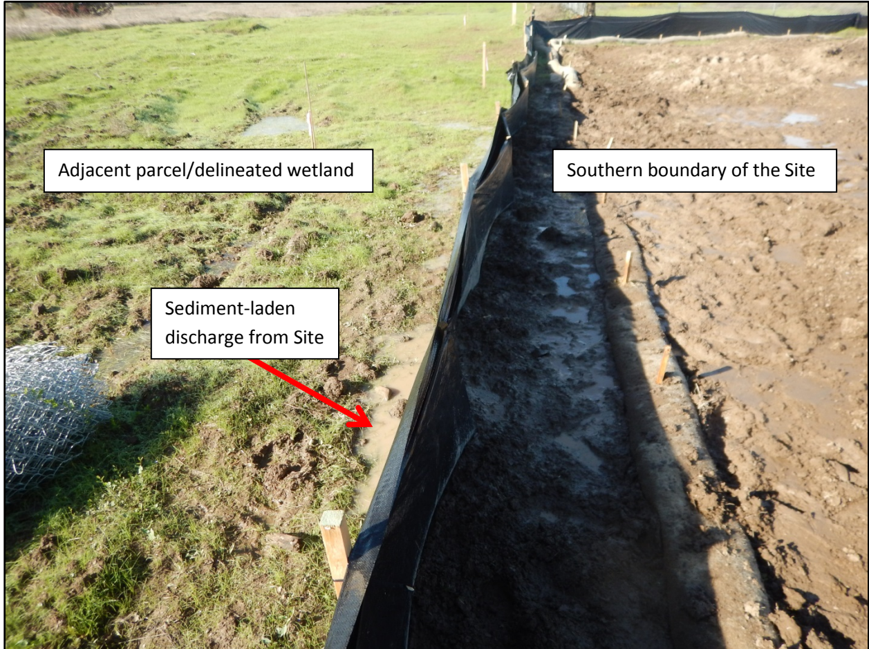
Photo 2. This photo depicts one of the discharges locations from the Site that Staff observed during the inspection. Staff observed a lack of erosion controls on the twenty-plus acres of disturbed soil onsite, plus inadequate sediment controls that were overwhelmed during the rain event that occurred in late October, 2016. Photo was taken facing roughly west at 10:48 on November 3, 2016.
