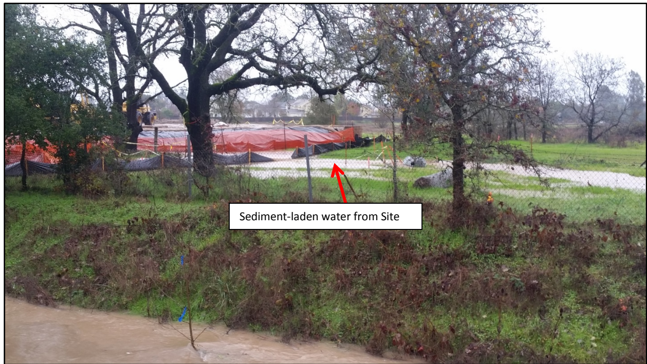
Photo 17. Sediment-laden storm water runoff overwhelmed a silt fence near the southwest corner of Site where the November 20, 2016, discharge was documented. This water flows to a swale on the adjacent property and into a drop inlet into Peterson Creek. Photo was taken facing southeast at 13:30.
