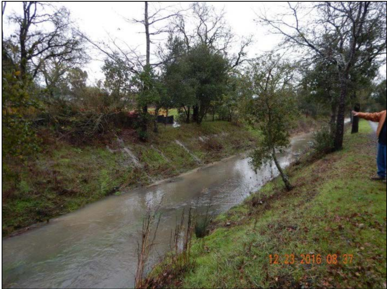
Photo 31. Peterson Creek discharge location 2. This discharge location appears to correspond with discharge sampling location #5 as provided in the 12/23/16 Sampling Field Log sheet. As shown in Photo 4, storm water was either passing beneath the silt fence or infiltrating and discharging at a uniform elevation on the bank of Peterson Creek. Storm water may have infiltrated and forced to emerge from the bank after hitting an impervious soil layer.
