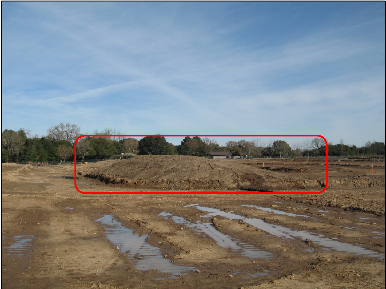
Photo 24. Stockpiled sediment lacked cover and a berm for perimeter control (red rectangle). As a result, the stockpile exhibited rilling. Photo was taken facing roughly north at 11:57.
