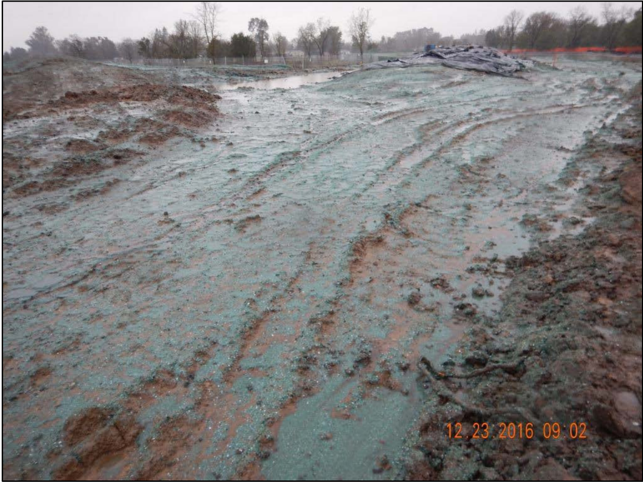
Photo 35. Disturbed area with hydromulch after rainfall.
