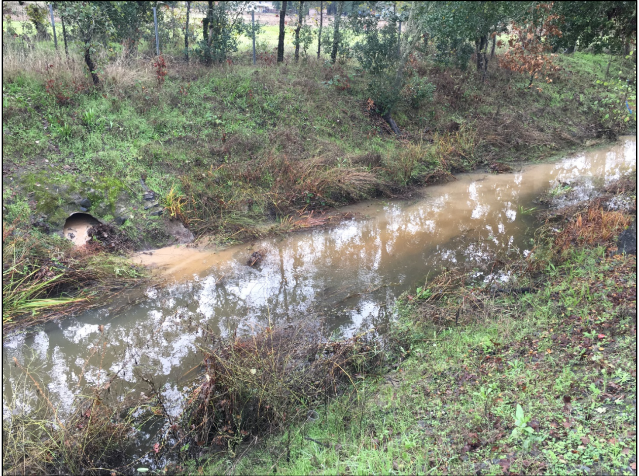
Photo 11. Sediment-laden water discharged from the site to Peterson Creek. Photo was taken facing southeast on November 20, 2016, at 09:13.
