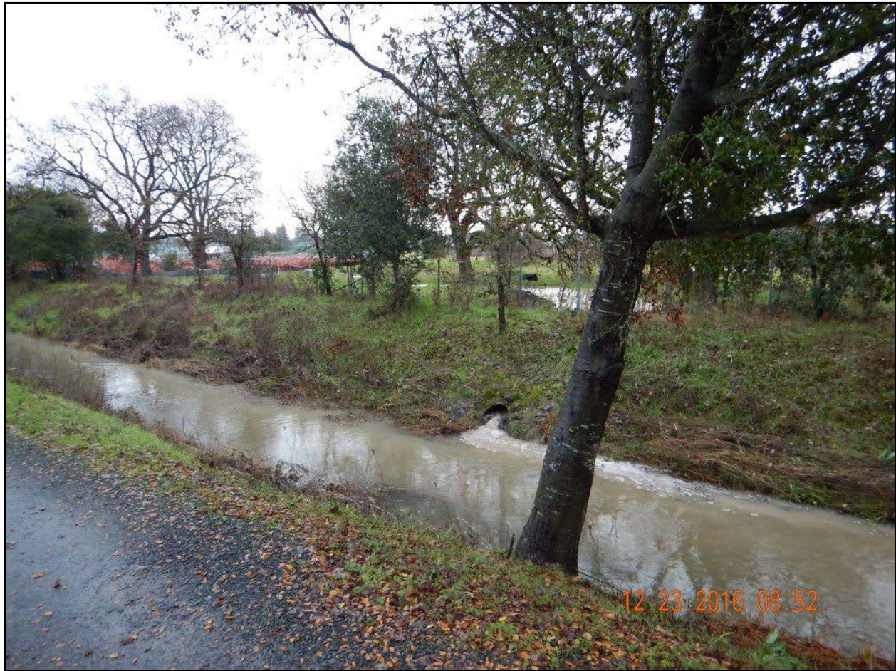
Photo 33. Peterson Creek discharge location 3. It was unclear where or whether this discharge originated from the Project site. This outfall does not appear to be listed as a discharge location on the 12/23/16 Sampling Field Log sheet, though sampling location #4 may be in the background at the silt fence, where runoff leaves the southwest Project boundary.
