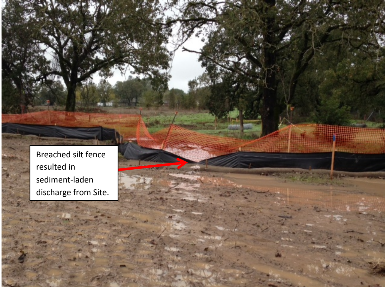
Photo 1. Sediment-laden water discharged from the southwestern corner of the Site. Clayton Jones of the City of Santa Rosa observed five discharges of sediment-laden water from the Site during his October 31, 2016, inspection. Photo was taken by Clayton Jones on October 31, 2016, facing southwest.
