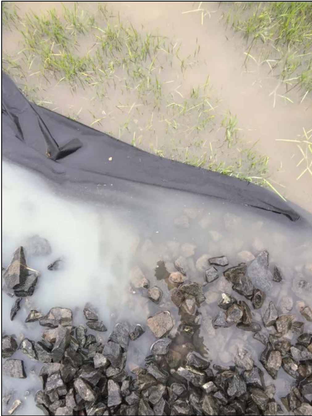
Photo 37. Photo taken within the eastern catchment. The storm water runoff on the bottom half of the photo is from areas treated with hydraulic mulch and has a green hue, unlike the water in the top of the photo, which is from areas largely not treated with hydraulic mulch. Ponded water throughout the Project area, in areas where hydromulch had been applied, had a green hue.
