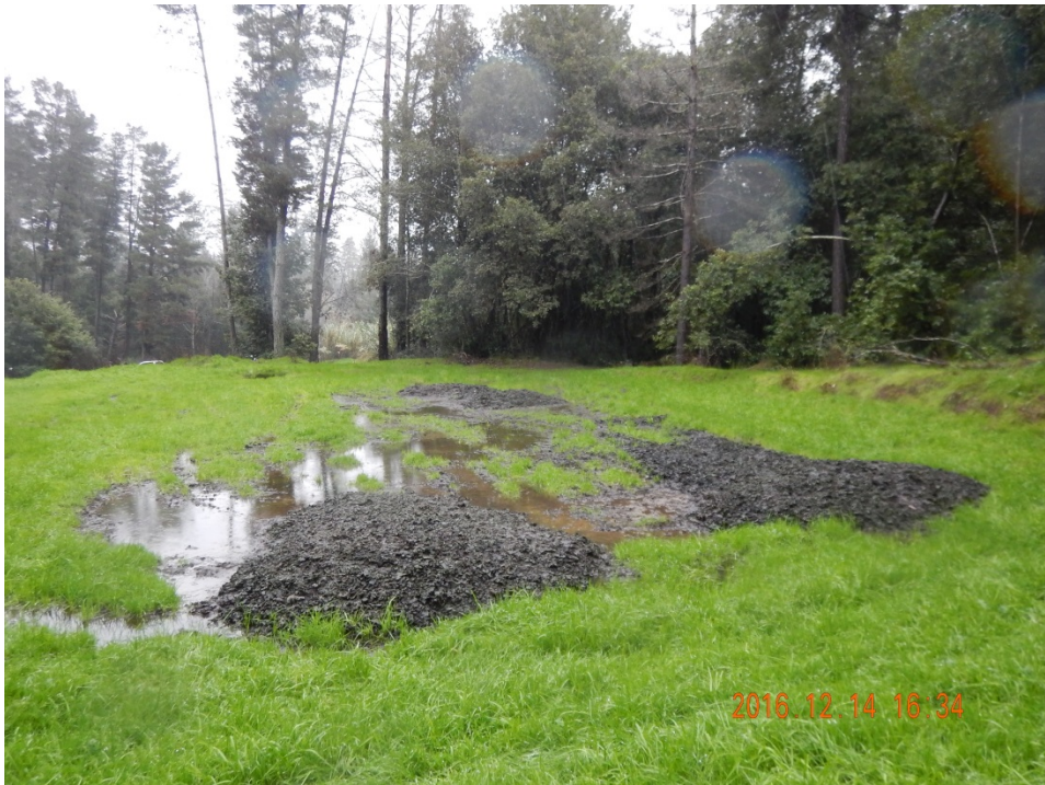
Photograph 2. Redway CSD – 12/14/16: Evidence of ponding water below sludge mounds on forested property northwest of the treatment plant. Photograph by Cathleen Goodwin, Regional Water Board staff
