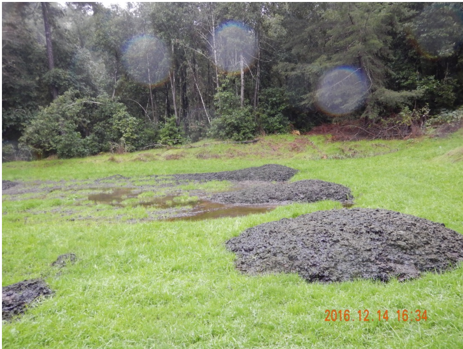
Photograph 3. Redway CSD – 12/14/16: Evidence of ponding water below sludge mounds on forested property northwest of the treatment plant. Photograph by Cathleen Goodwin, Regional Water Board staff
