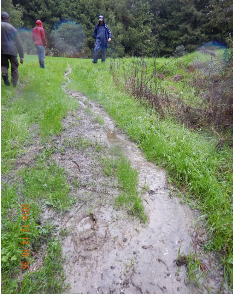
Photograph 6. Redway CSD – 12/14/16: Evidence of sediment laden runoff occurring from sludge disposal area on the forested property northwest of the treatment plant. Photograph by Cathleen Goodwin, Regional Water Board staff
