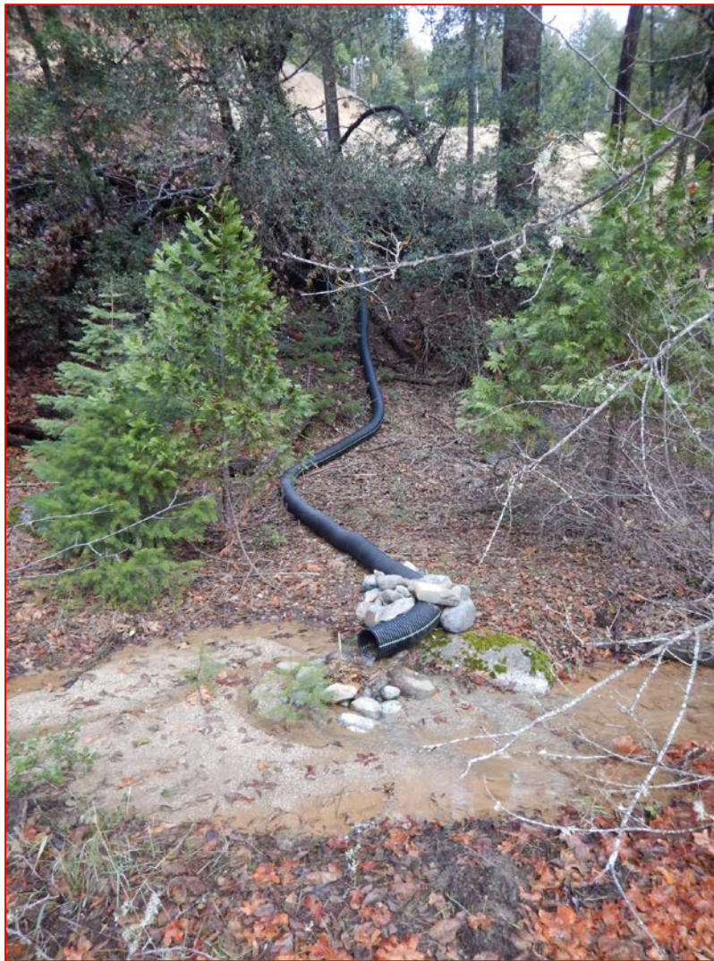
Figure 2: Six-inch plastic culvert discharging to the edge of the floodplain of Stuart Fork
