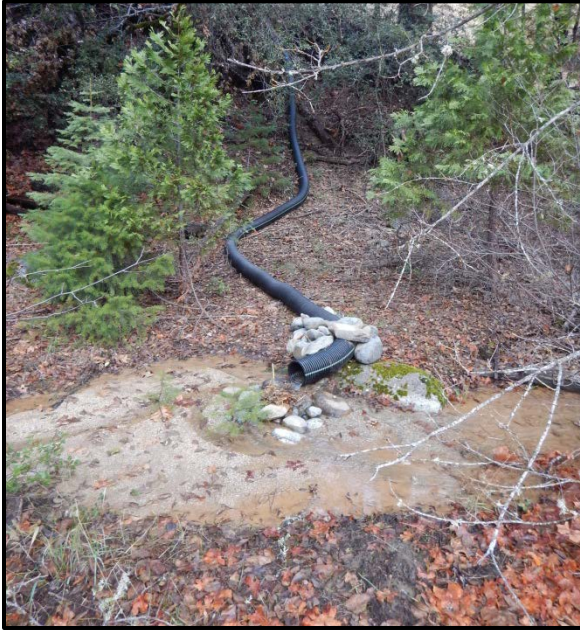
Photo 6: Plastic flexible pipe discharging onto Class I floodplain of Stuart Fork (Forest Fortescue, November 29, 2016)
