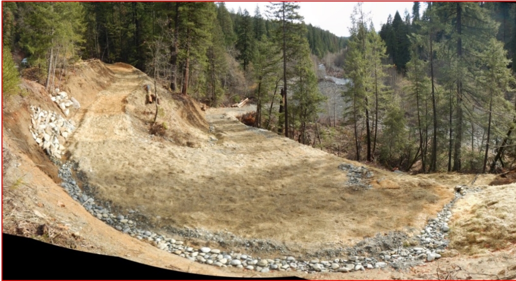
Figure 6: Panorama of the new seasonal road switchback and ditch, taken from top of the DG cut slope on the shoulder of Trinity Alps Road
