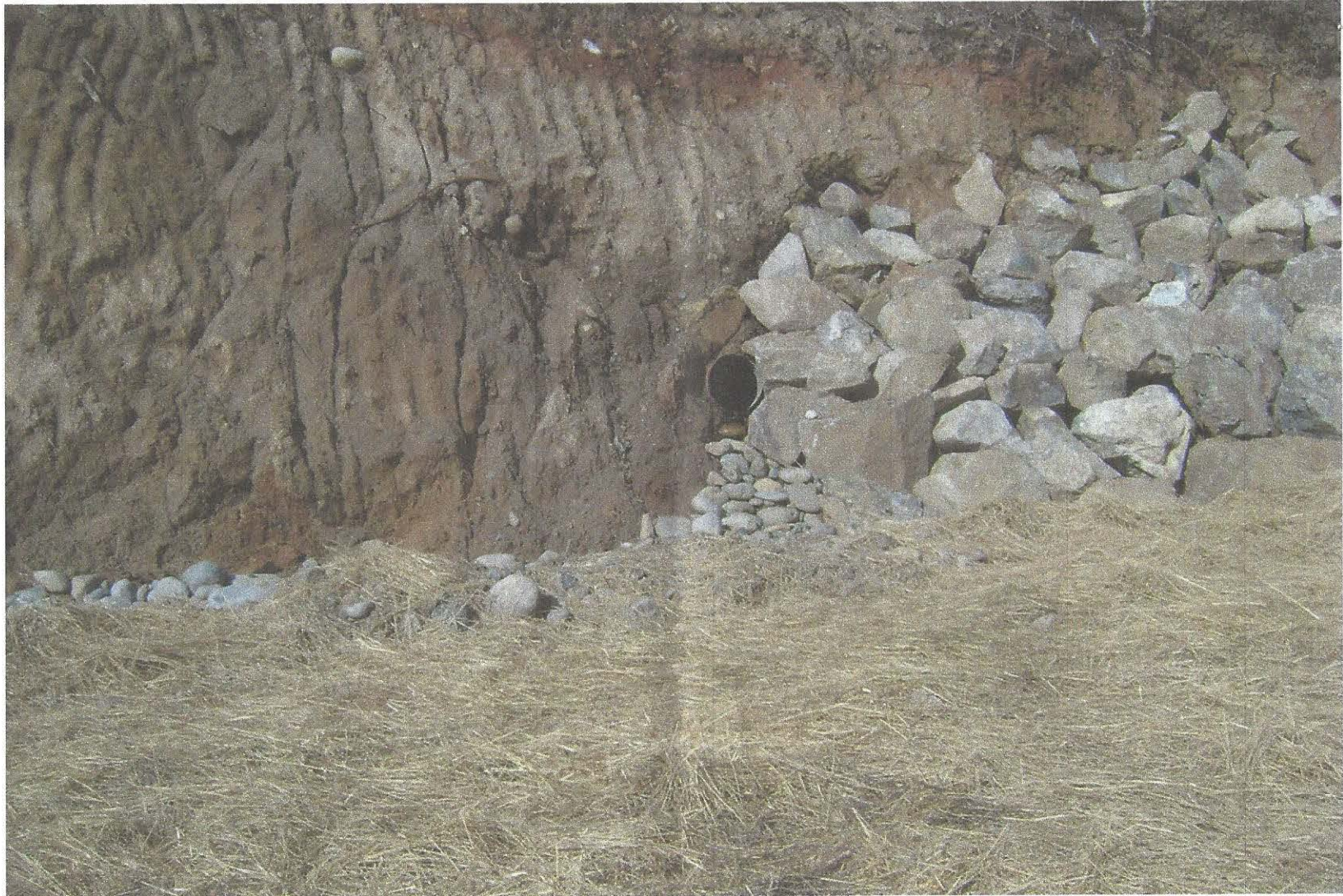
DSC01926- Culvert crossing above P1 and P2.
