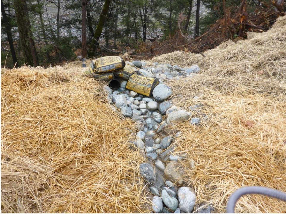
Figure 2: Crossing P2 Inlet
