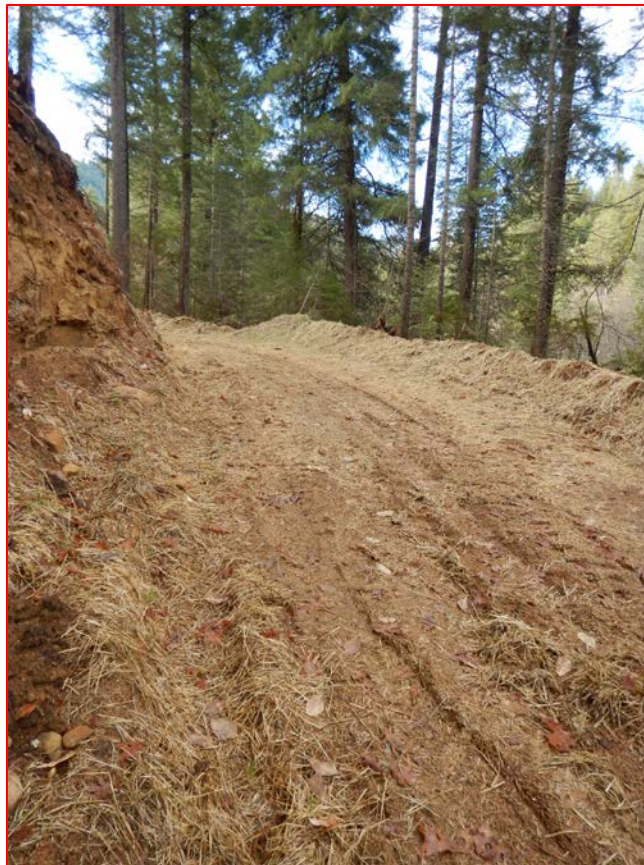
Figure 9: Portion of the new temporary road construction between T1 and L5
