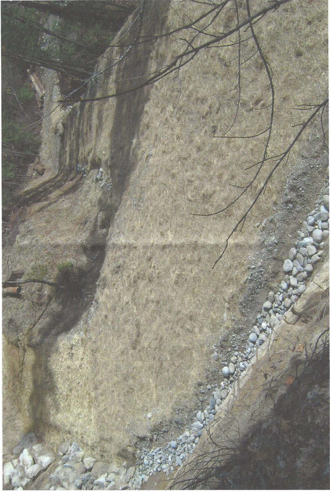
DSC01929- Overview of site.
