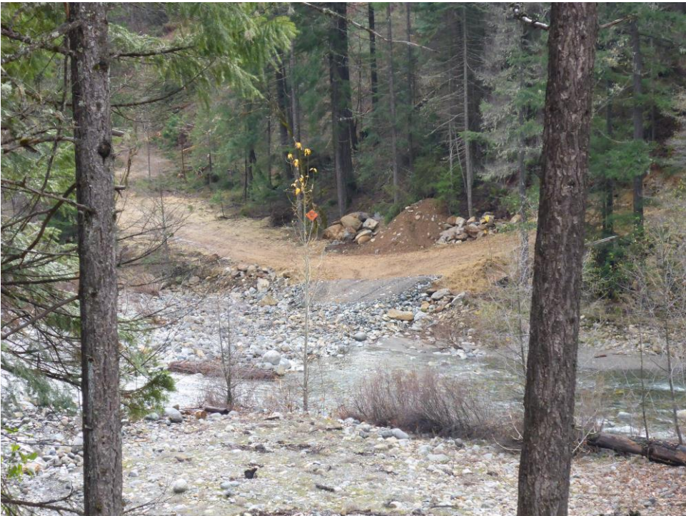
Figure 5: Loose fill placed at T1
