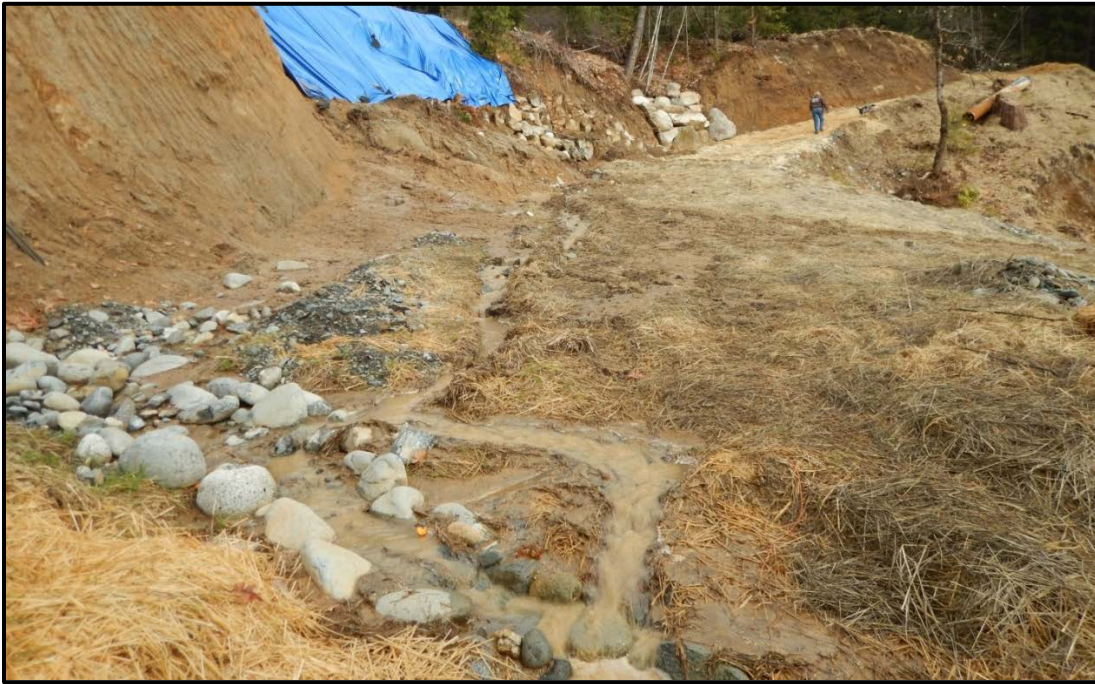
Photo 3: Hand dug drainage channel across the switchback (Graham Brown, December 20, 2016)
