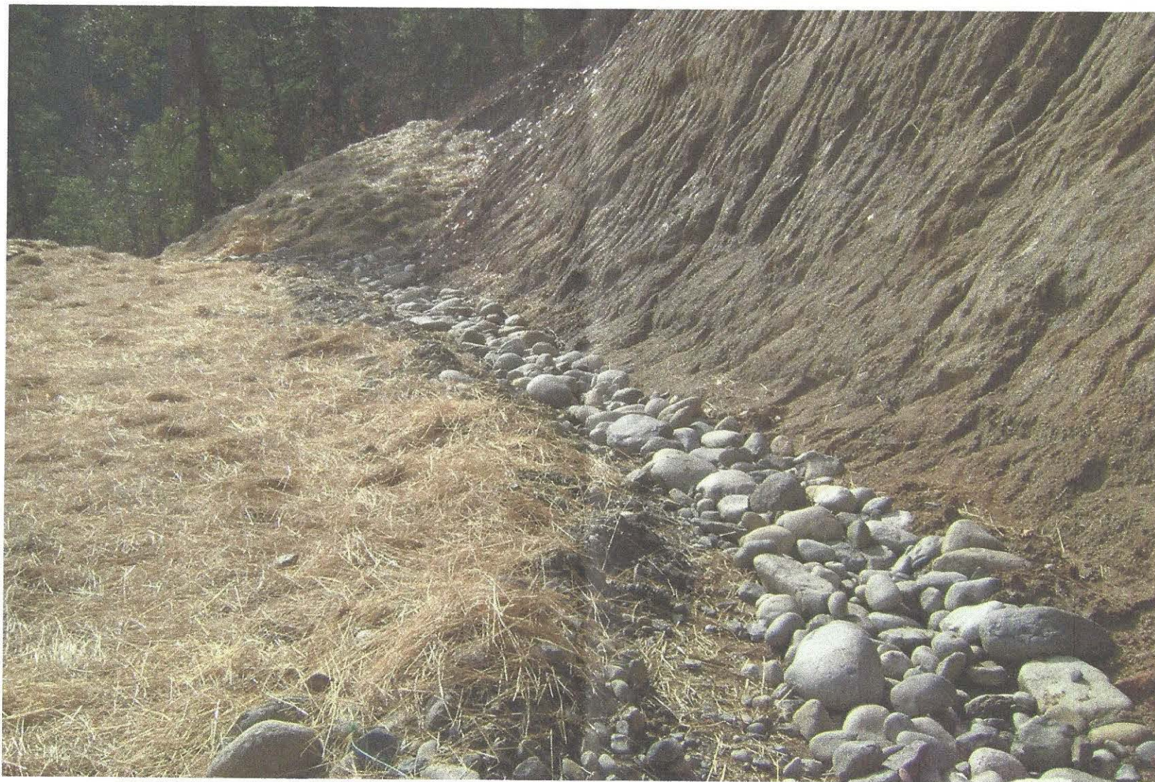
DSC01928- Inside ditch used to divert flow around P1 and P2.
