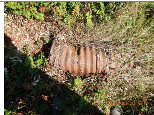
Photo 21: Area C. Old culvert debris in Islas Slough channel at approximate latitude/longitude 41.921795, -124.193744.
