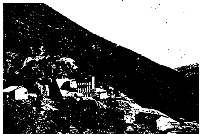
FIGURE 13. Headframe and ore treatment plant at the Lions Den mine, Cachuma district, Santa Barbara County. This mine was a producer during World War II.
