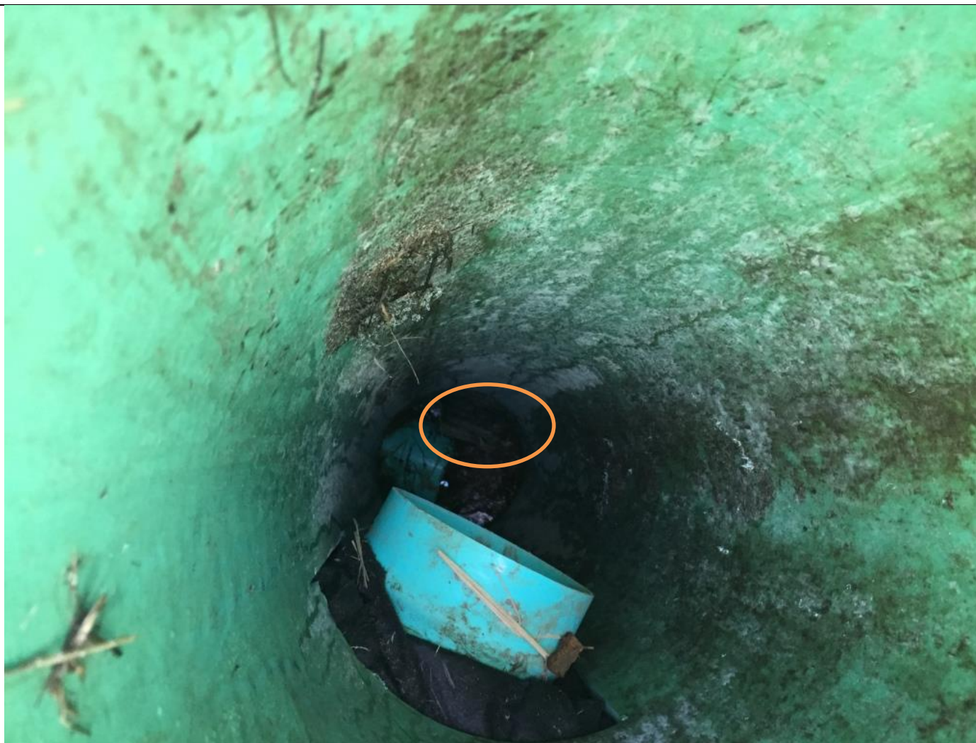
Figure 16: Inside the vertical pipe. There were three pipes protruding into the vertical pipe at differing elevations. At the lowest elevation there was a black, perforated plastic pipe—this pipe is hard to see in the photo and is within the orange circle. Higher in elevation above that pipe were two blue, solid plastic pipes. Figure 17 shows the likely pipe flow paths.
