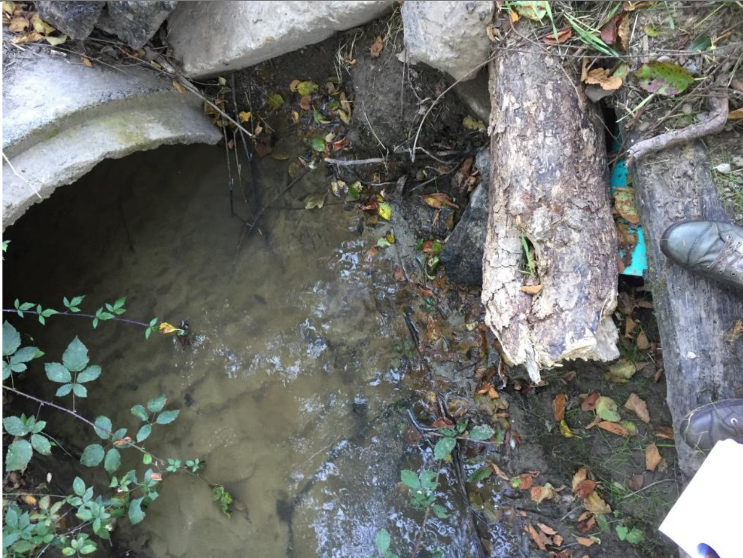
Figure 30: A view of the outfall, ostensibly a continuation of the uppermost pipe in the vertical pipe. It appeared that wood had been deliberately placed over the outfall.
