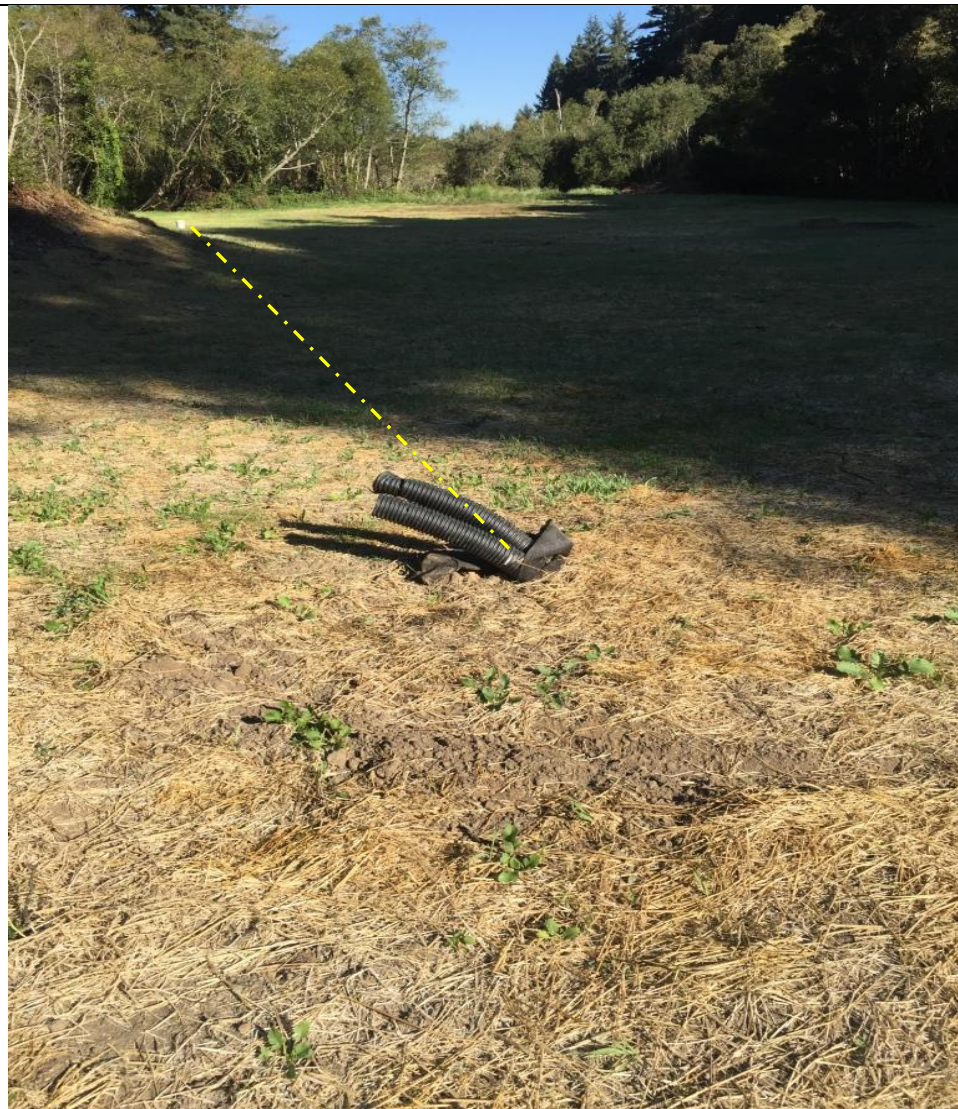
Figure 26: Looking northwest toward the forested wetland and the vertical pipe. There were two black, plastic perforated pipes wrapped in filter fabric sticking out of the ground. It is unknown where each pipe goes, but if one of them goes to the vertical pipe then it may take a path approximated by the dashed yellow line.
