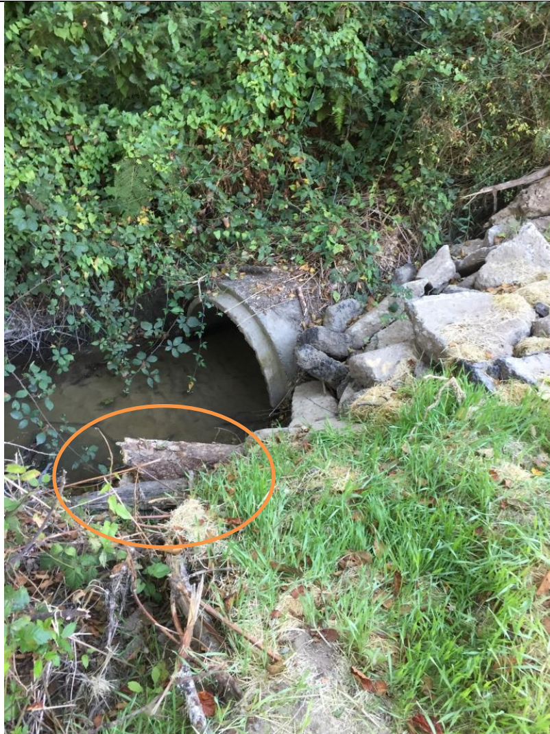
Figure 29: A close-up of Third Slough where it enters a culvert at the eastern parcel boundary. The blue plastic pipe outfall is beneath the wood shown within the orange circle (see Figure 30). The concrete rubble to the right of the culvert appeared recently placed; I suspected there may be another drain outlet beneath the rubble, due to circumstances described in Figure 33 and Figure 34, but could not locate an outlet when peering between the rubble.
