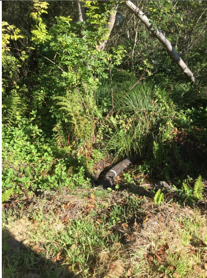
Figure 21: Close up of the possible drain shown in Figure 20. This was coming out of the ground and appeared to be a pipe covered in filter fabric.
