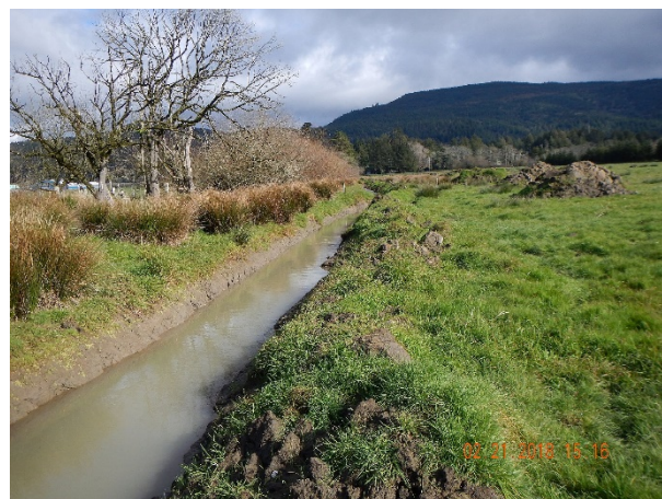
7. Spoil piles placed in wetlands
