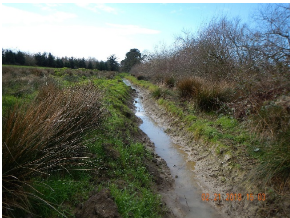
4. Walking west along drainage ditch
