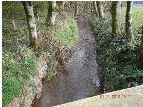
5. Bridge crossing of Morrison Creek for cow grazing access
