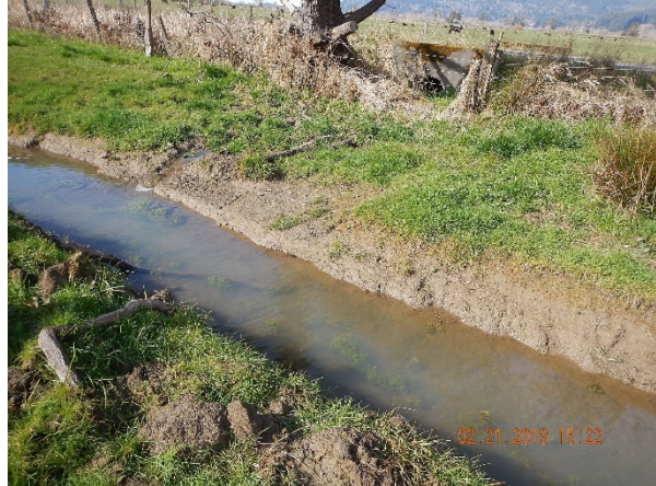
9. Ditch in low spot collecting neighboring fields' runoff
