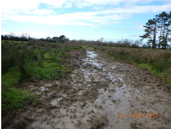
2. Looking west along beginning of trench
