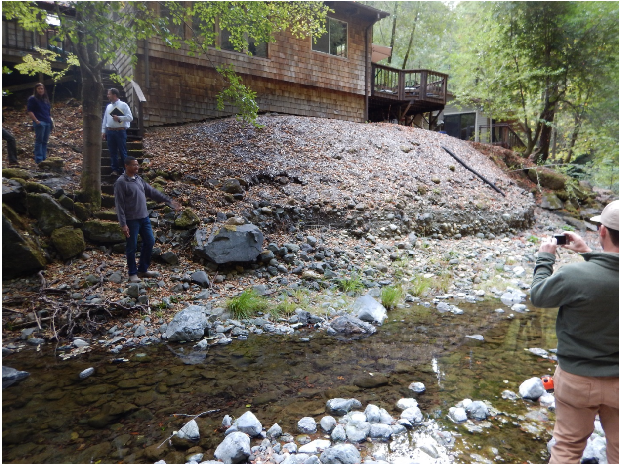
Figure 6: Original condition of northern part of site. Photo taken by Kaete King 9/24/2015
