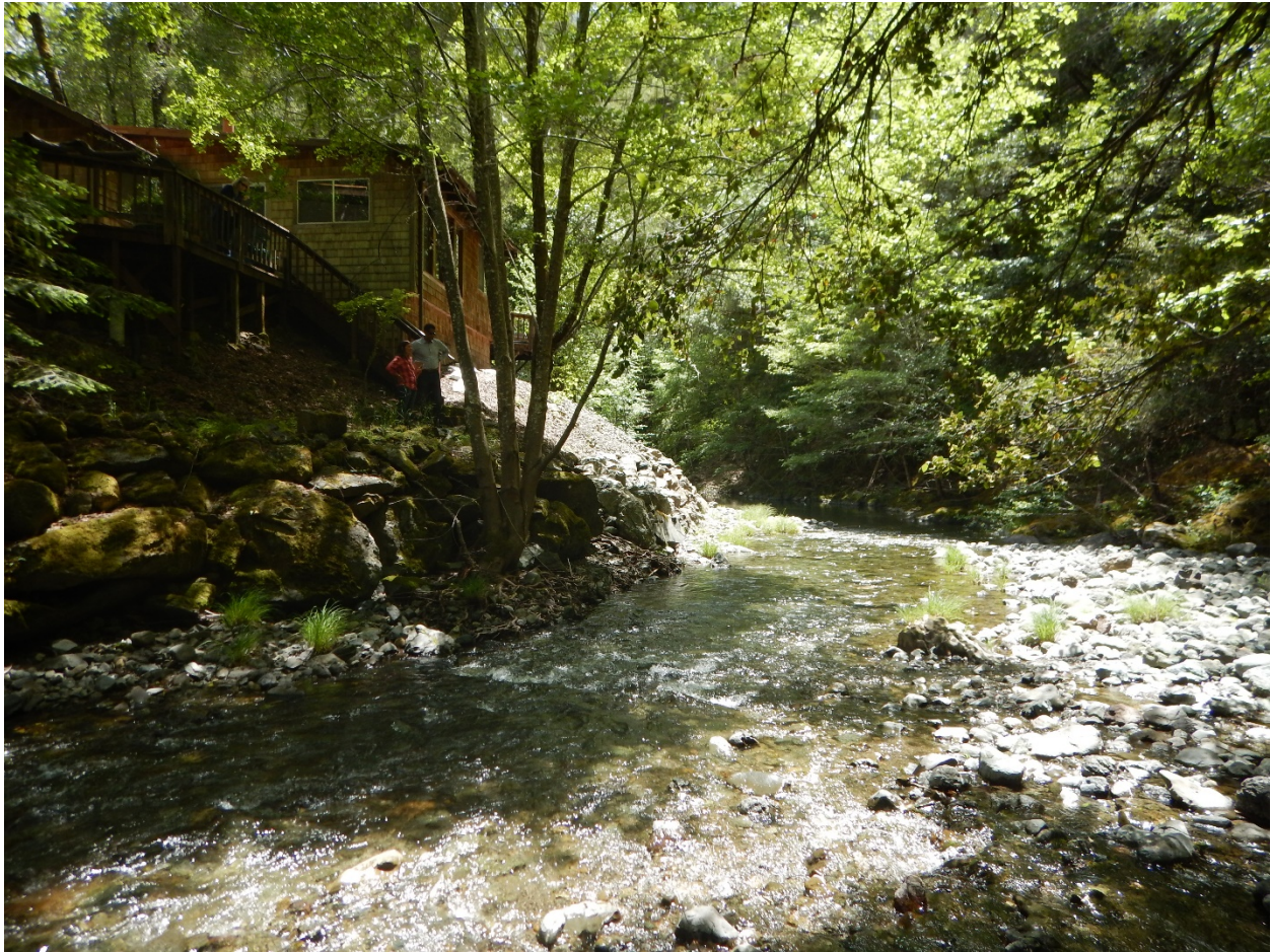
Figure 5: Site overview post-construction. Rip rap visible at toe of slope. Additional fill material behind/upslope from rip rap. Photo taken by Kaete King 5/10/2018.
