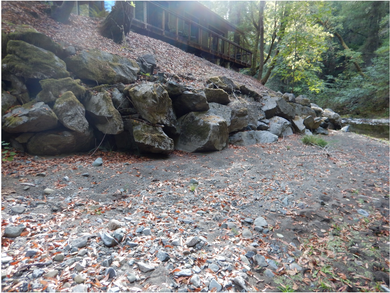
Figure 10: Existing rip rap below southern structure. Just 14 linear feet of RSP was proposed in this area, with additional planting-only at the top of the slope. Photo taken by Kaete King 9/24/2015.
