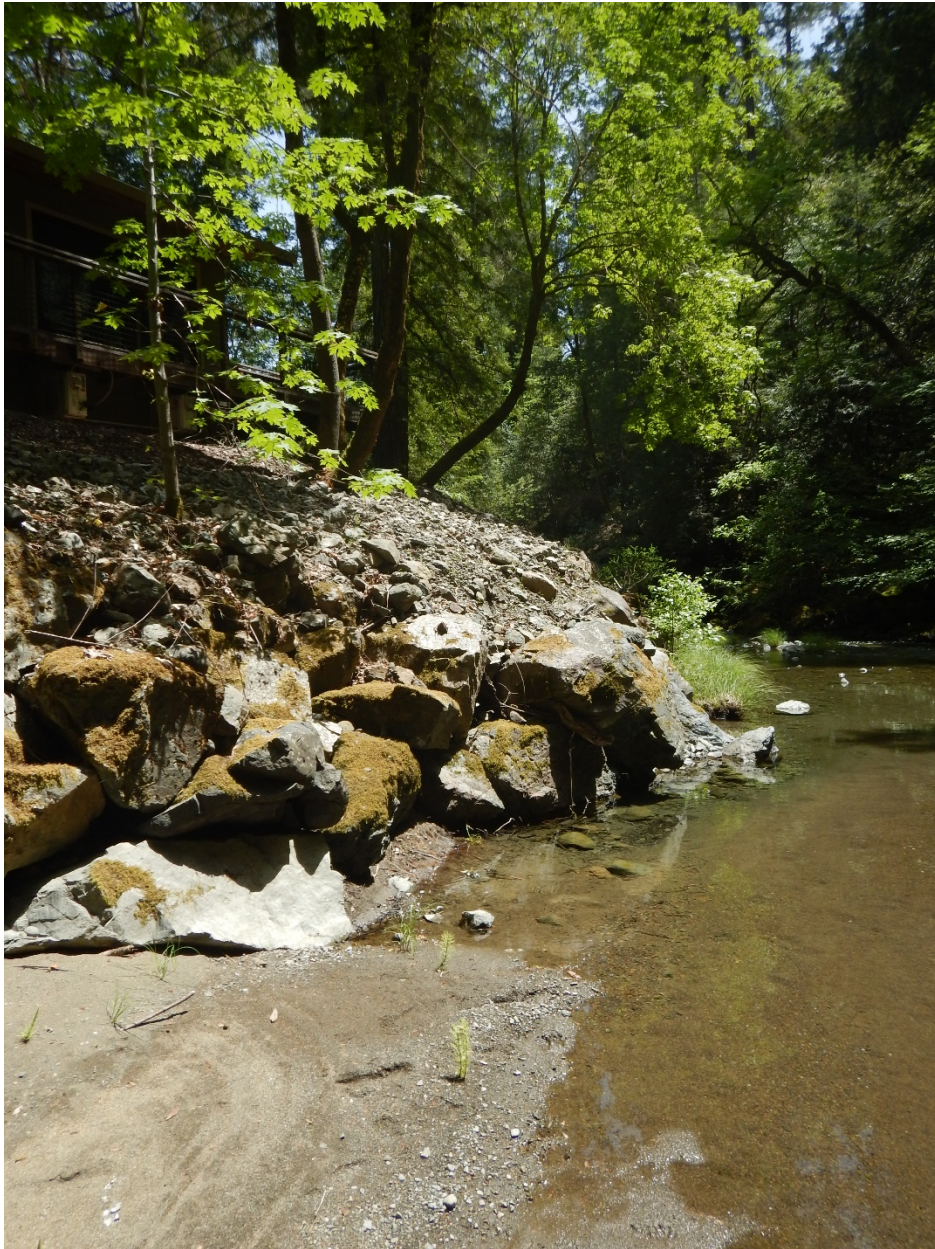
Figure 15: Photo angle reversed from Figure 14. This photo is looking downstream. View of access route that was developed for construction. Small-diameter fill material has been left on slope above existing rip rap. Photo taken by Kaete King 5/10/2018.
