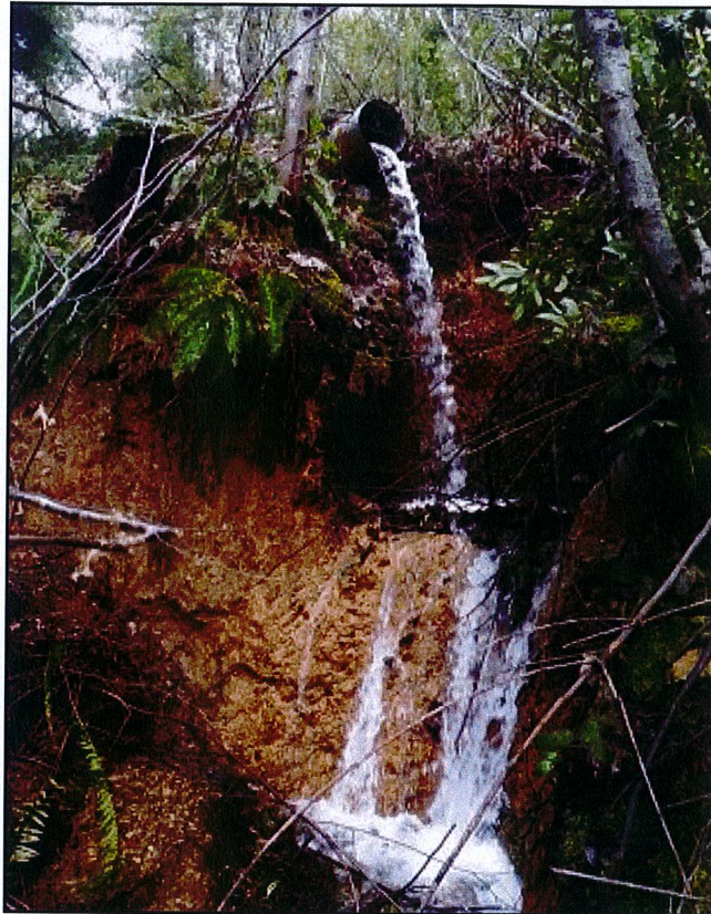
Photo #1. Existing Irving Creek Outfall. Taken by Fiori Geosciences.
