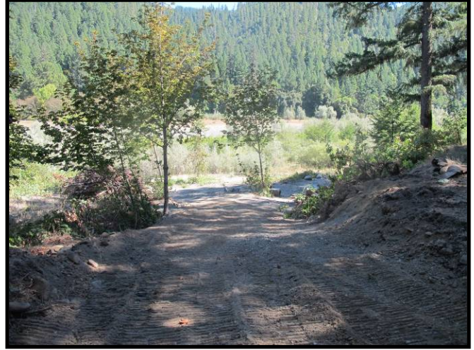
A 200 foot access road was constructed between an existing roadway and the project site, across the Klamath River floodplain. This access road was seeded and mulched after project construction was completed. Images above left and right show the access road from the top, before and after construction. Below, the perspective show's a more complete view of the access road from the top and across the river floodplain.
