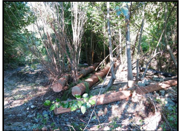
Five 30' logs with rootwads attached were locked into existing vegetation at the head of the off-channel pool, designed to redirect sediment around the project area in high flow events. The upper left and right photos show a close up, before and after, of the log placement, while the photo below shows the structure in relation to Stanshaw Creek and the off-channel habitat during winter flows.
