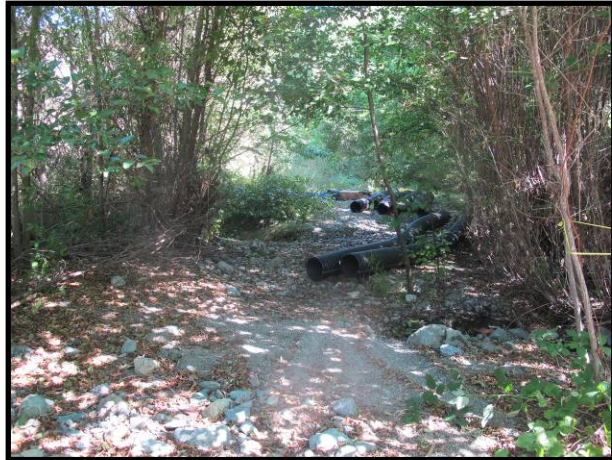
Five 30' logs with rootwads attached were locked into existing vegetation at the head of the off-channel pool, designed to redirect sediment around the project area in high flow events. The upper left and right photos show a close up, before and after, of the log placement, while the photo below shows the structure in relation to Stanshaw Creek and the off-channel habitat during winter flows.
