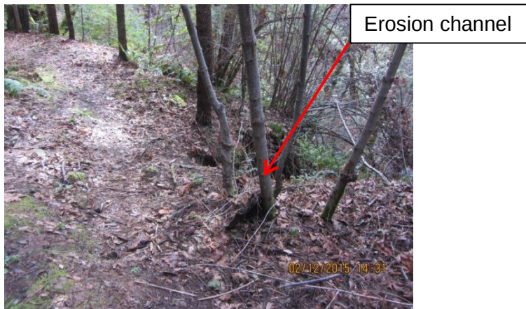
Image 6- shows the erosion channel downslope of Point 3.
