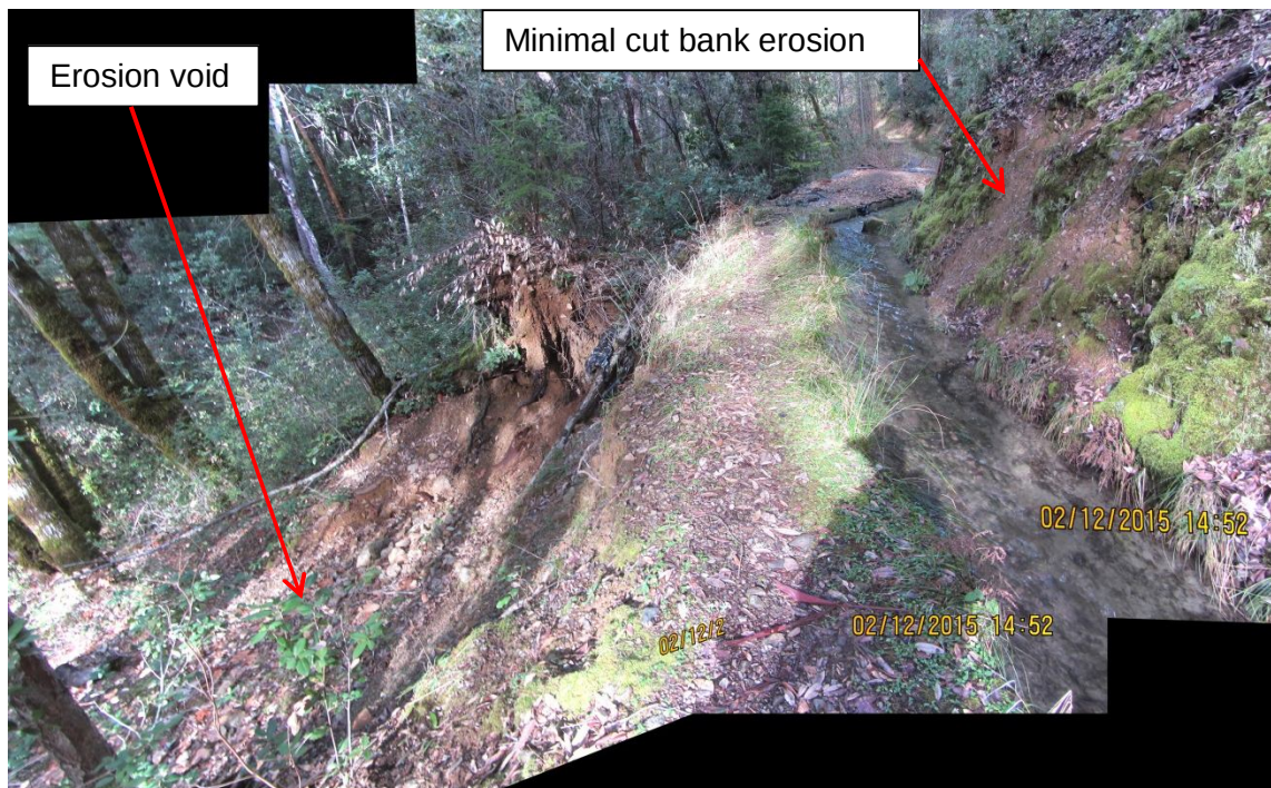
Image 16- Point 10 is an area of concern that includes an erosional channel likely formed by a berm failure and active erosion visible on the cut bank. I observed active cut bank erosion on many of the upper slopes above the diversion ditch and expect that bank slumps have and are contributing significantly to ditch failures. (Photos 8495, 8496, 8497, and 8498 composite image).
