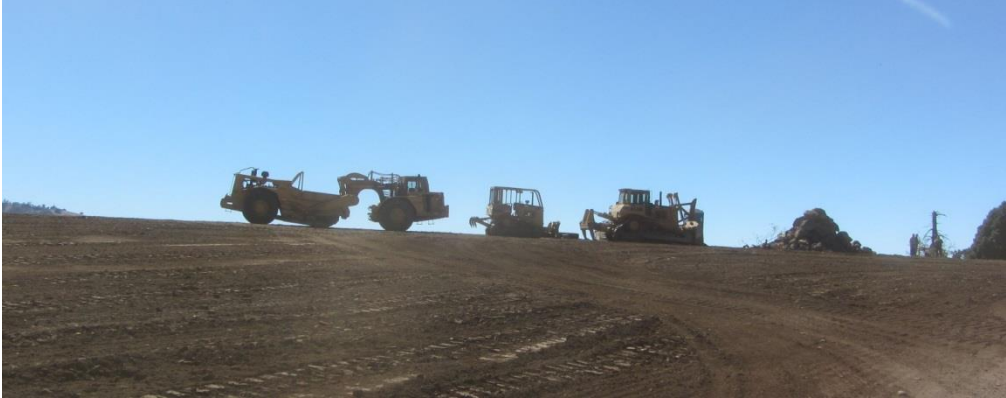
Image 11 shows the equipment observed on site. (IMG 0244 cropped))
