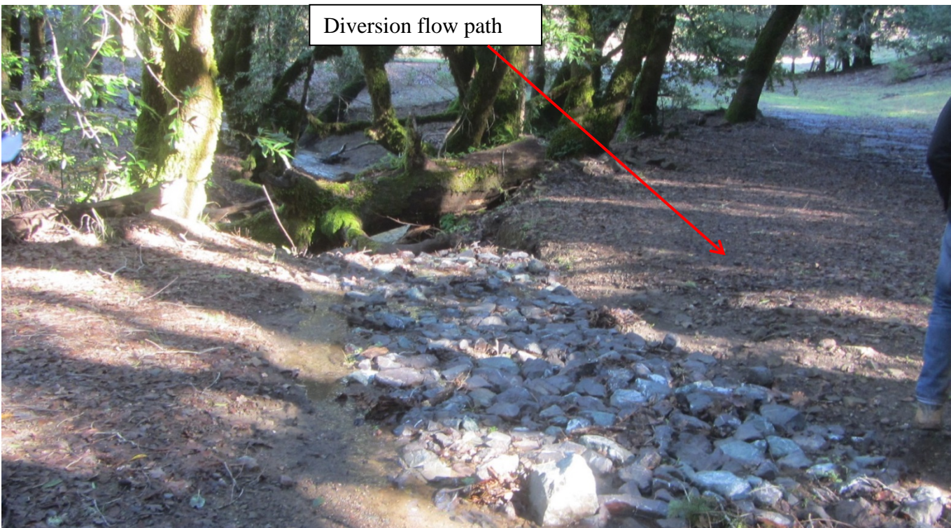
Image 39 shows a closer view of the shallow ford and the diversion of flows out of the channel and down the road surface to the flat area in the far right of the image. (IMG 3065 cropped)
