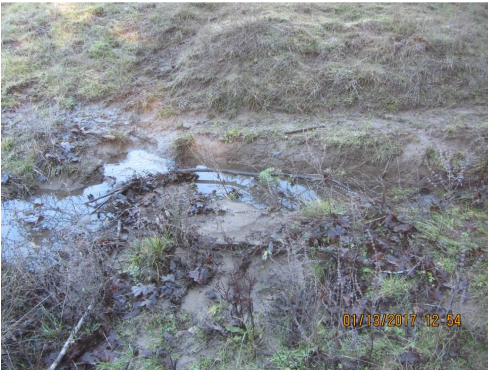
Image 30 shows a close up of the fine sediment deposits mentioned in the caption of image 29 preceding this image. These fine materials are transporting and delivering to the Class III stream intercepted by the inside ditch and to the Large Class II stream at Stream Crossing 7. (IMG 3047)
