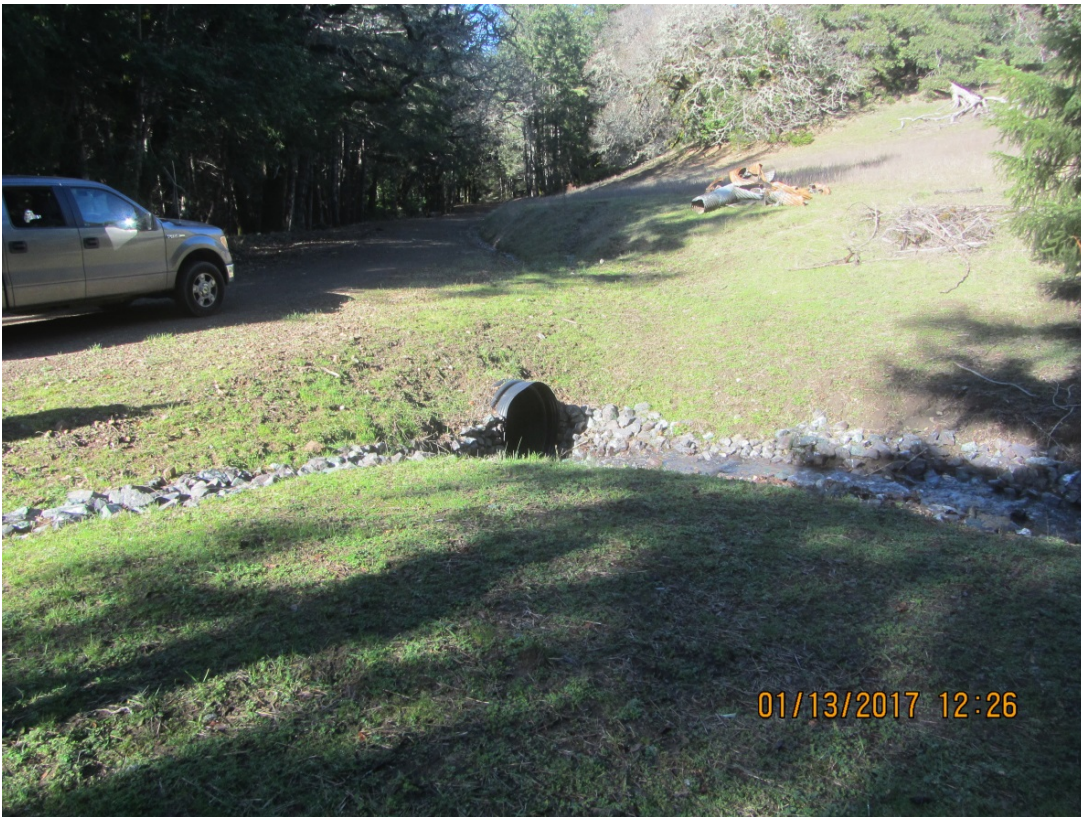
Image 23 shows the inside ditch along the access road delivering to the inlet of Stream Crossing 4. (IMG 3019)
