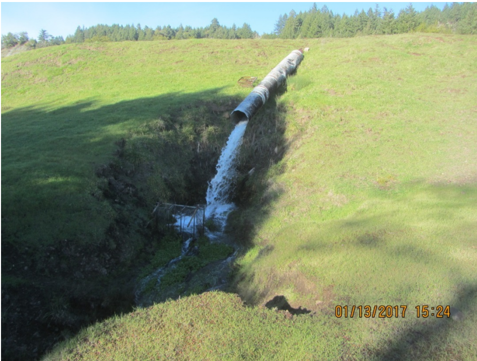
Image 69 shows the spillway to GPS8. (IMG 3178)
