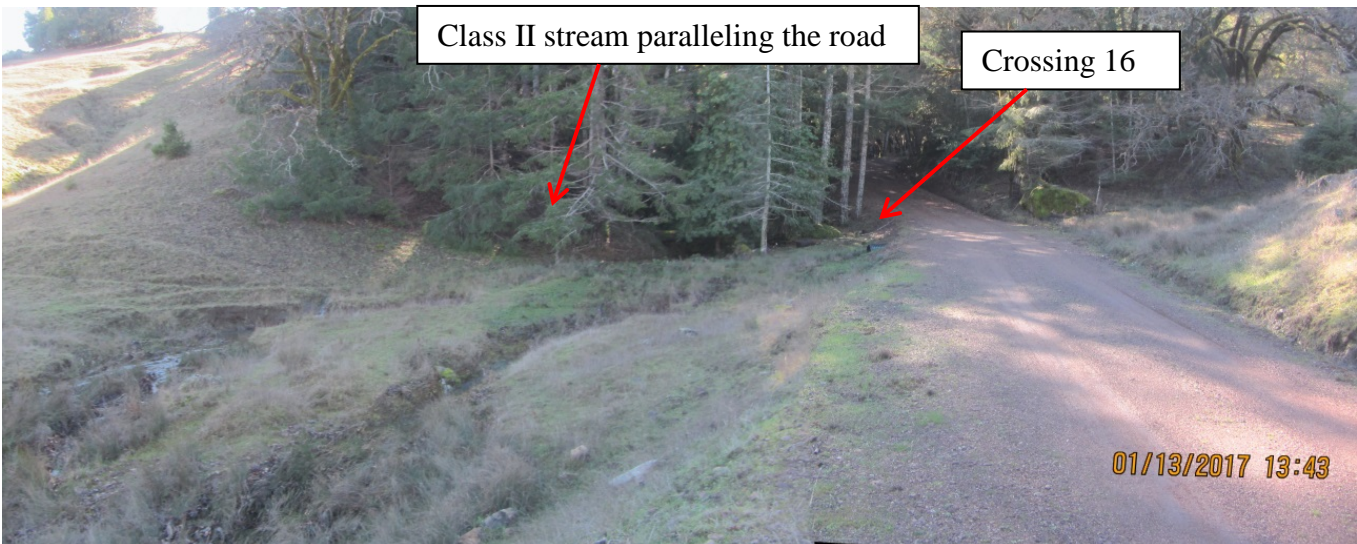
Image 51 shows the Stream Crossing 16 wetlands and the Class II stream that parallels the access road. (IMG 3103-3104 stitch)
