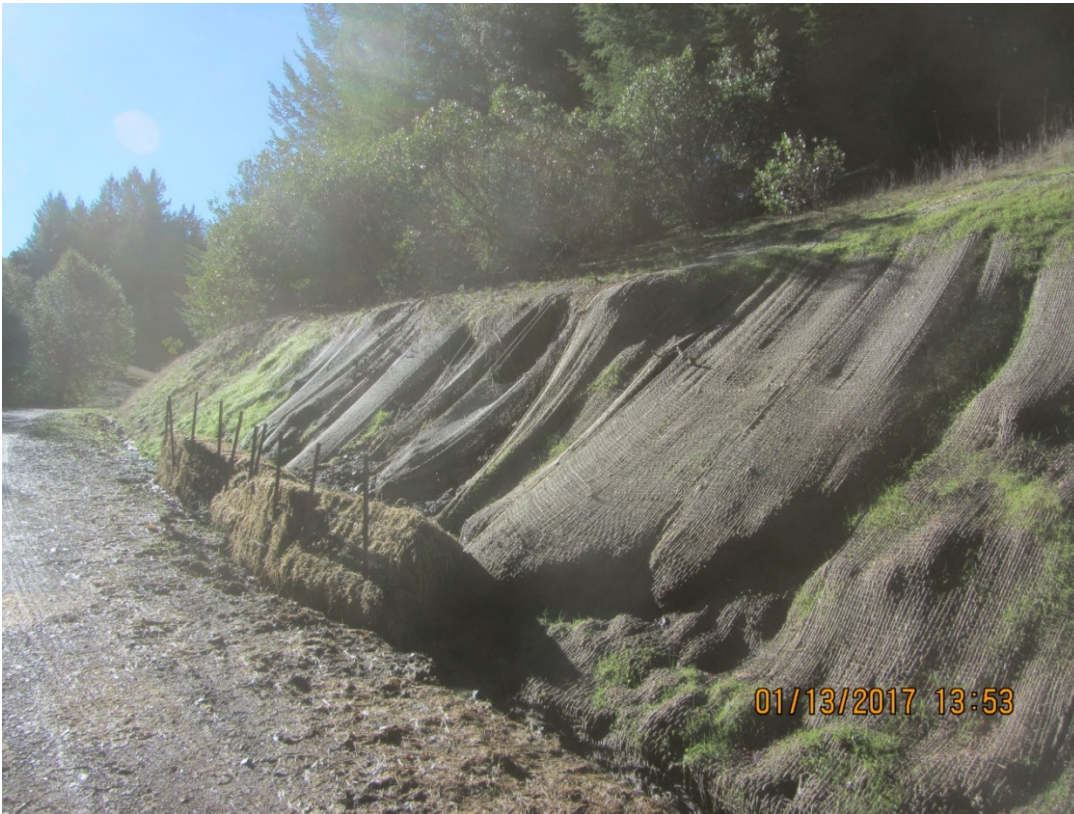
Image 54 shows the top of the second unstable cut bank on the approach to Stream Crossing 17. (IMG 3112)
