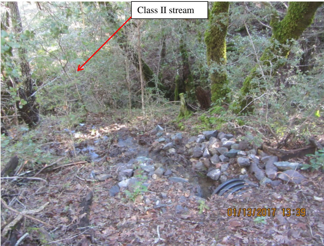
Image 48 shows the outlet of the ditch relief culvert at Crossing 14. (IMG 3089)
