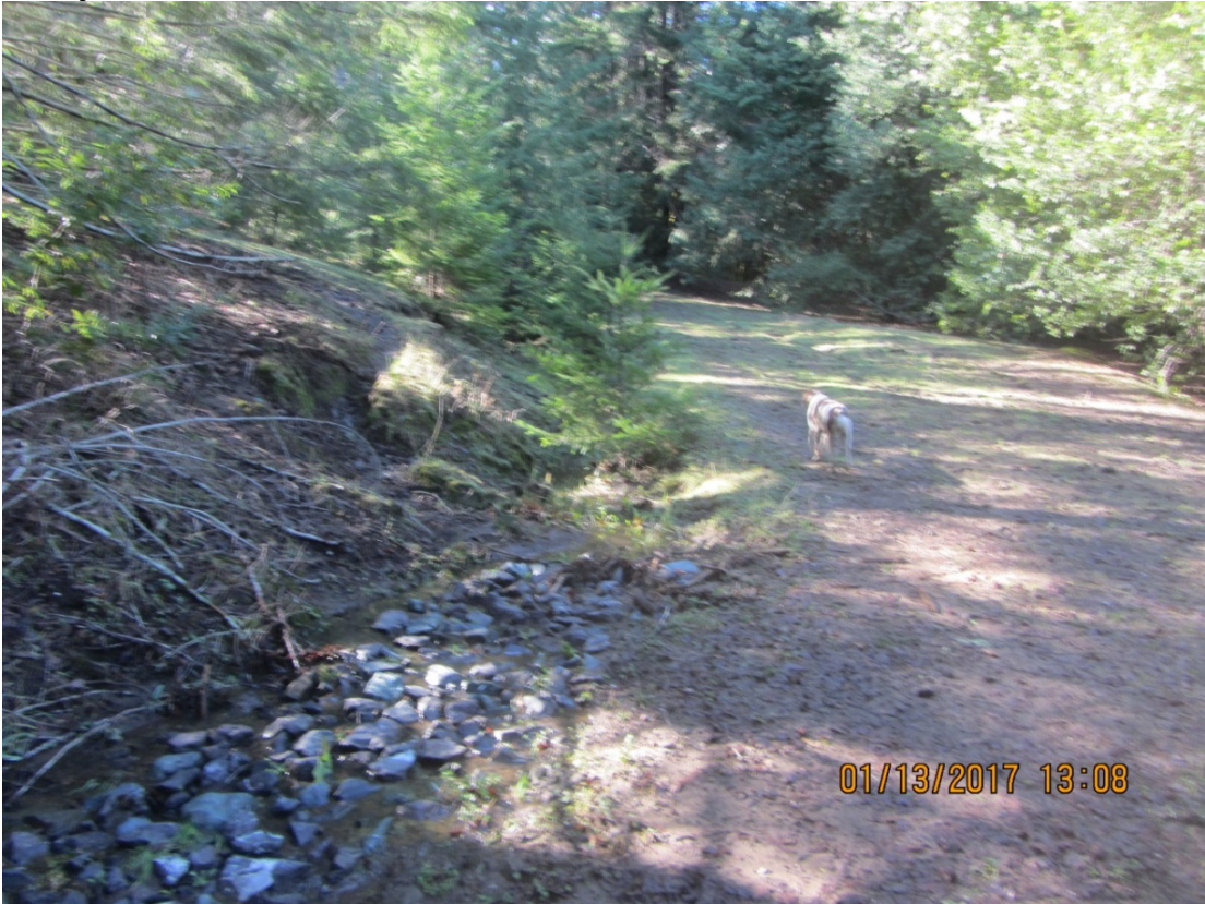
Image 37 shows the Class II stream diverted down the inside ditch of the road west of Crossing 9. (IMG 3064)
