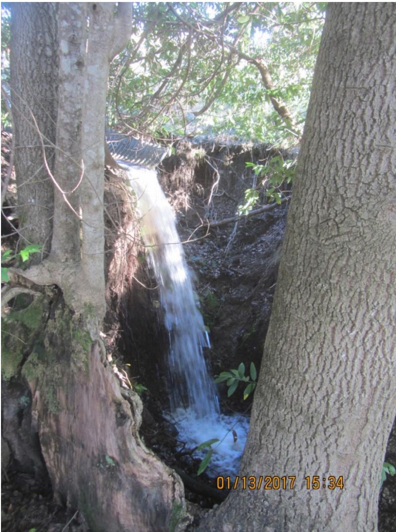
Image 73 shows the outfall of the half-round spillway of the pond located at GPS8. (IMG 3200)
