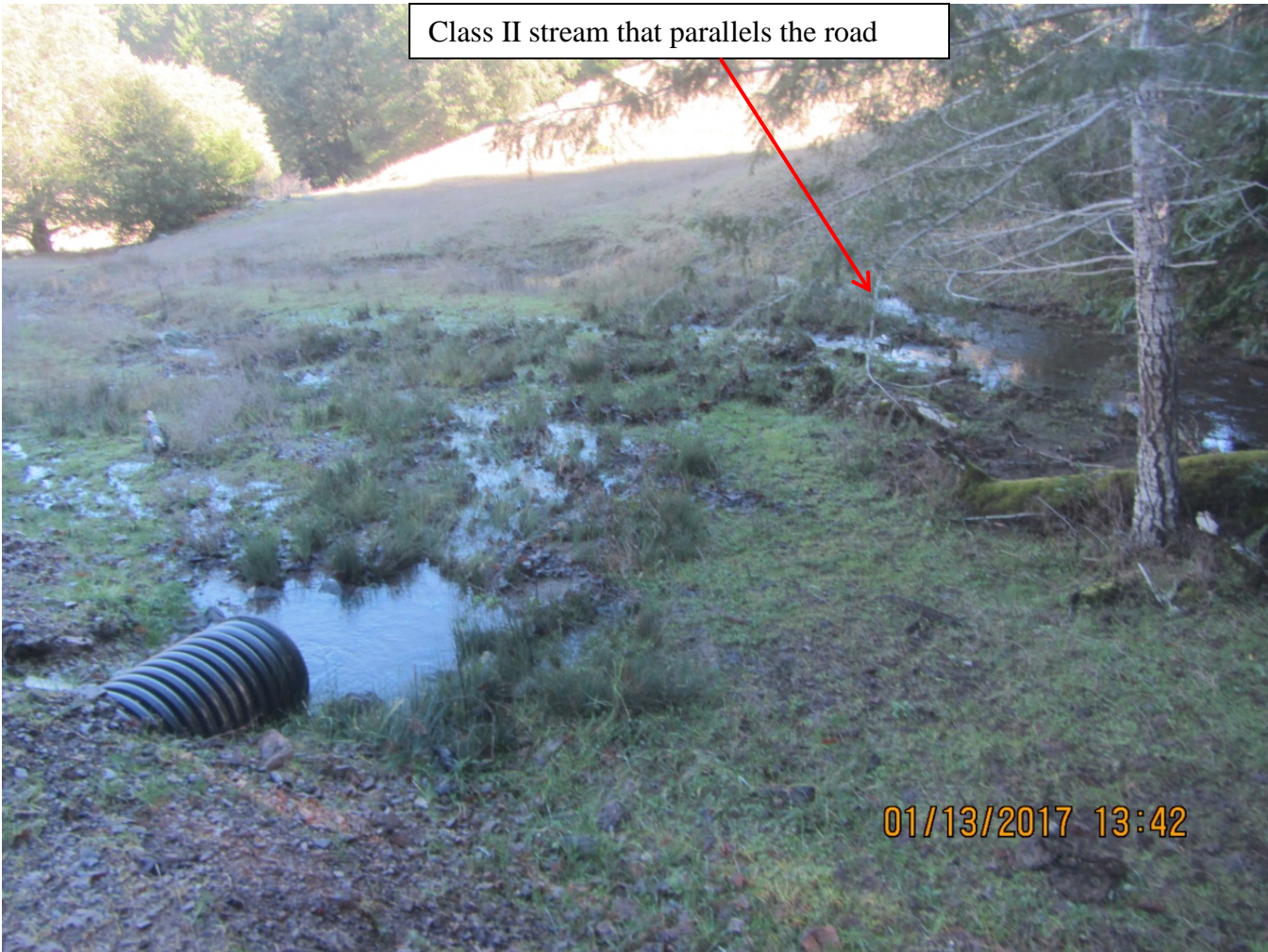
Image 50 shows the outlet of Crossing 16, note the heavily grazed juncus and spread of water through wetland vegetation. (IMG 3097)
