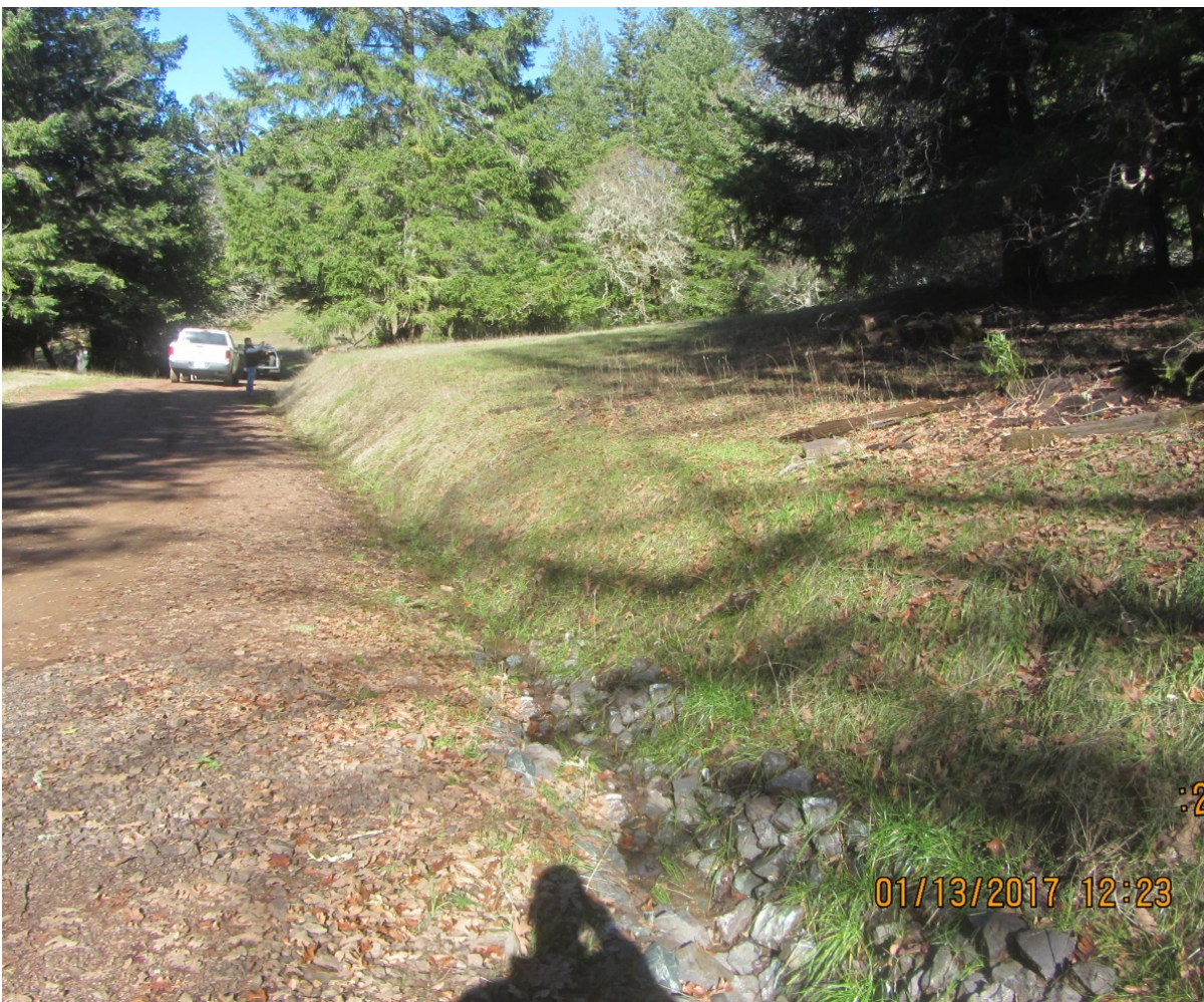
Image 22 shows the inside ditch along the access road near stream crossings 2 and 3. (IMG 3008-3009-3010 stitch)
