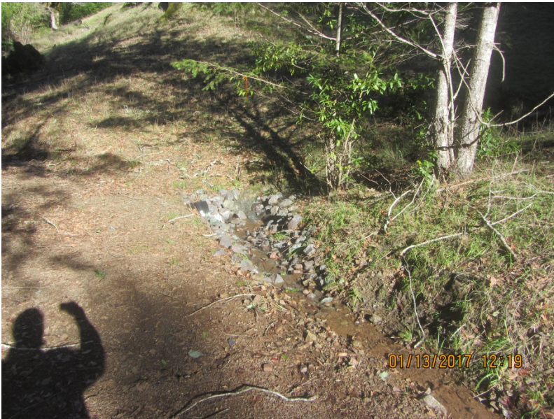
Image 18 shows stream crossing 2 inlet and inside ditch; note the fine sediment in the ditch and erosion of ditch banks delivering to the stream. (IMG 3003)
