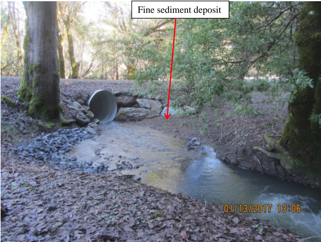
Image 36 shows the inlet of Stream Crossing 8 and the fine sediment deposit from the upstream diversion and overland flow. Also of note is the placement of rock armoring along the left bank of the image. (IMG 3063)
