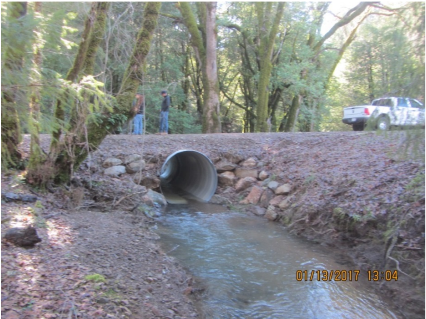
Image 35 shows the outlet of Stream Crossing 8. (IMG 3056)
