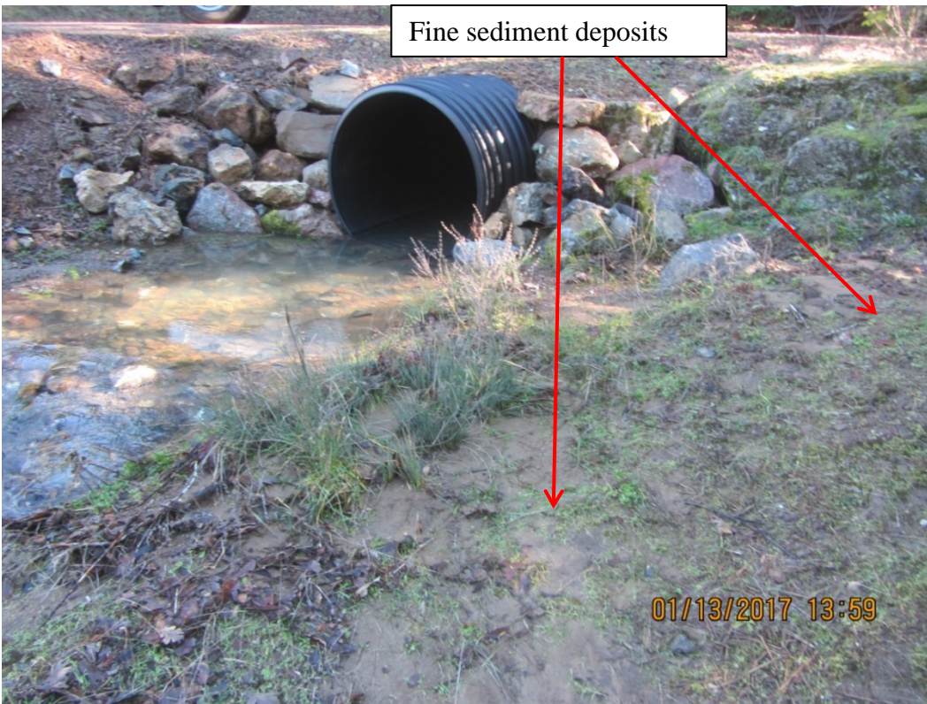
Image 57 shows the Stream Crossing 17 outlet; note the fine sediment deposits from road surface runoff and the active high flow channel. (IMG 3126)
