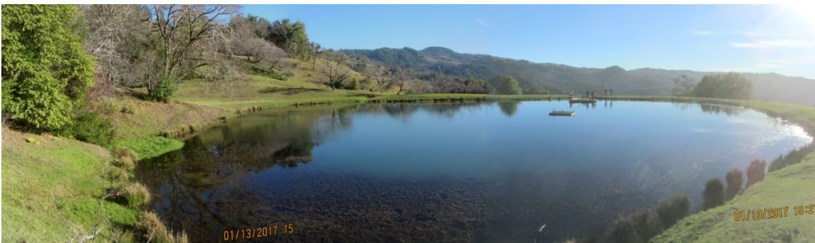
Image 68 existing pond located at GPS8. ((IMG 3170-3172))
