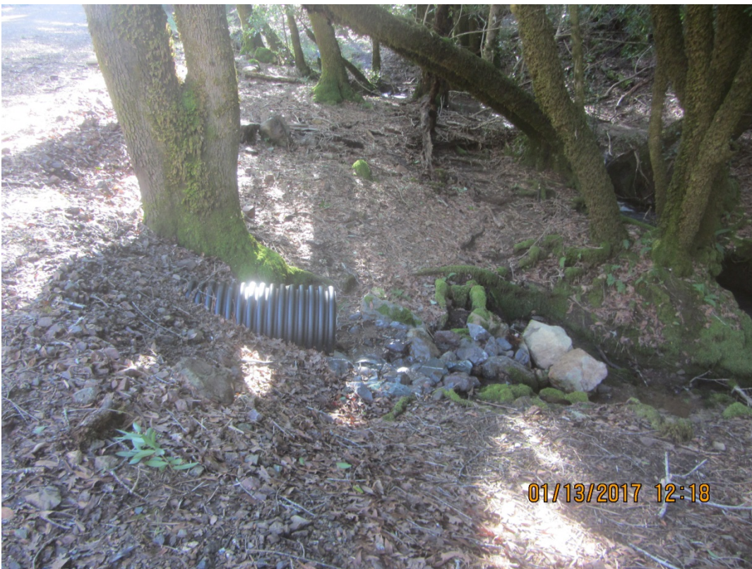
Image 19 shows the stream crossing 2-culvert outlet to the Large Class II stream originating at the vineyard. (IMG 3001)
