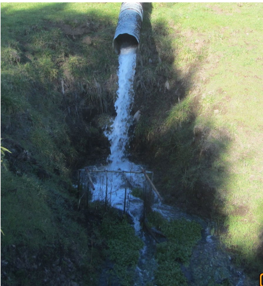
Image 70 shows the Spillway in a closer view note the head cut visible behind the falling water. (IMG 3179 cropped)
