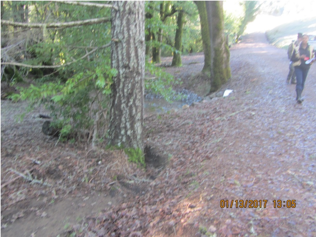
Image 41 shows the erosional channel off the flat as it is leading to the inlet of Stream Crossing 8. (IMG 3058)
