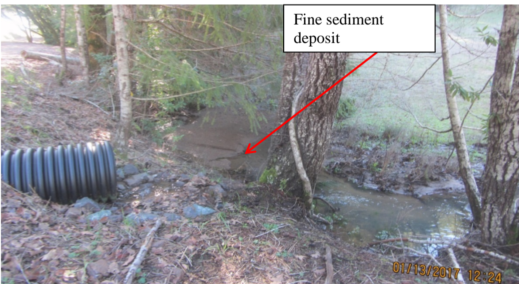
Image 21 shows the outlet of Stream Crossing 3 and an example of instream fine sediment deposited upstream of the culvert outlet. The observation is of background fine sediment loading in the stream flowing from the developed vineyard, and not one associated with the functionality of this culvert. (IMG 3014-3015 stitch)
