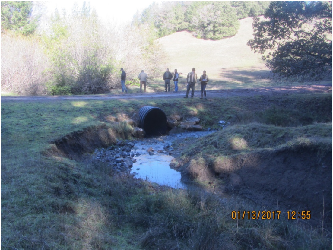
Image 31 shows the inlet of Stream Crossing 7. (IMG 3049)
