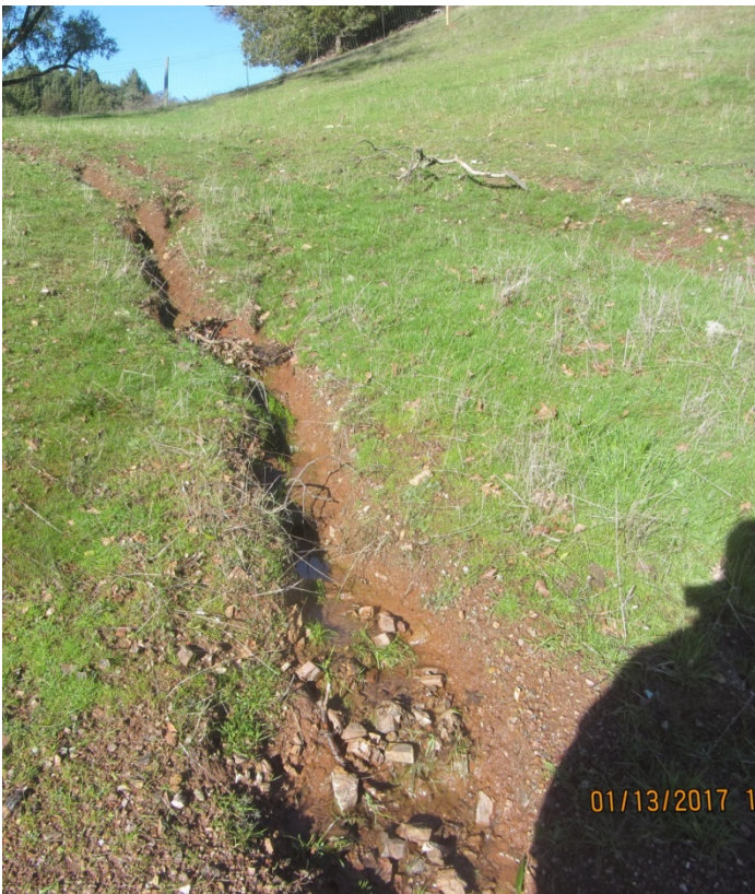
Image 8 shows the spring observed during the inspection flowing into the pond. (IMG 2969-2971)
