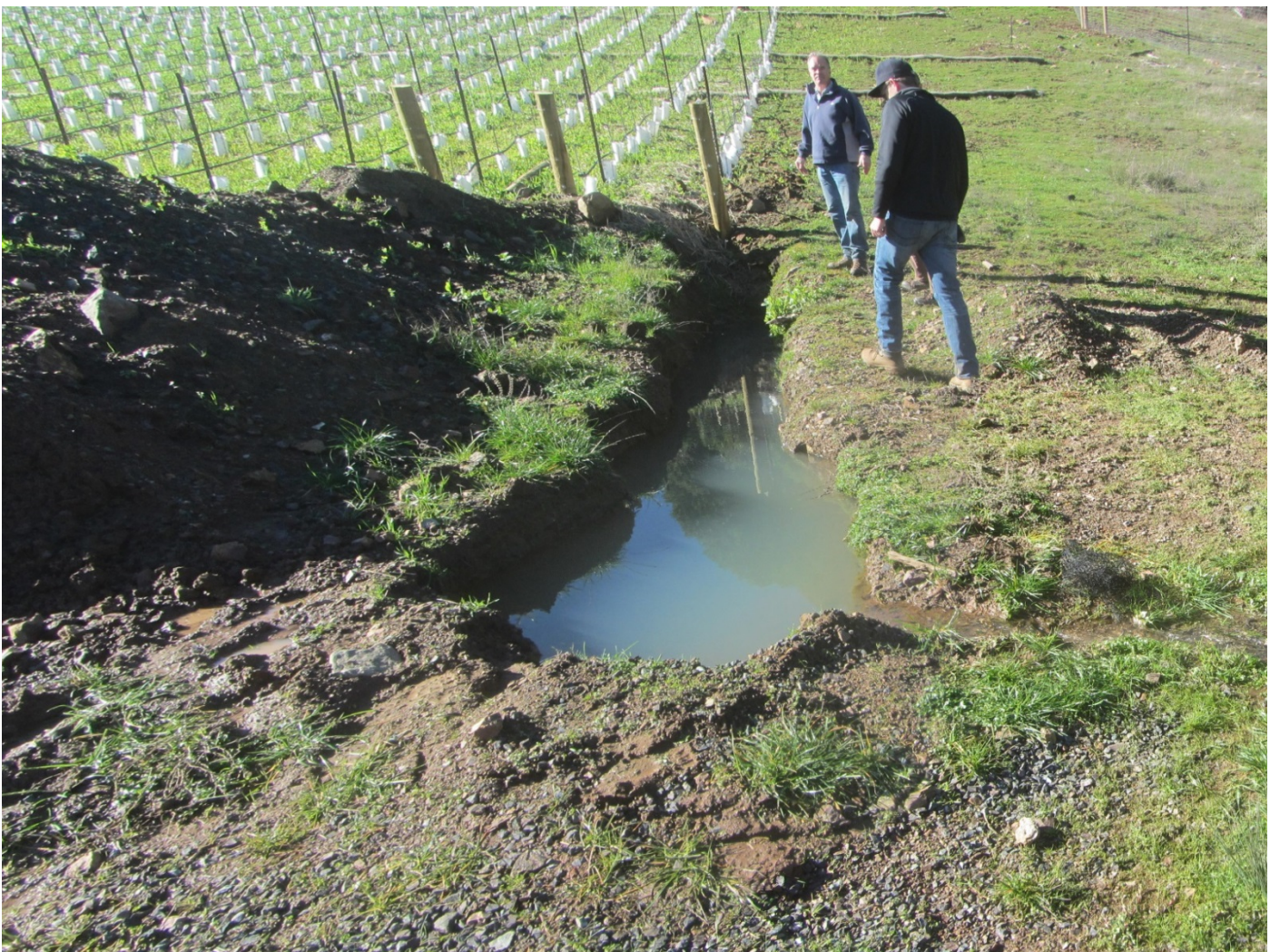
Image 13 shows the downstream slope from the vineyard where a recently dug ditch intercepts what appears to be the buried stream, which was flowing during the inspection. The spoils generated digging the ditch are likely contributing sediment to the stream. (Image 2979-2980 Stitch)
