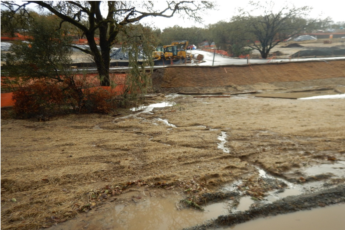
Picture 15 above. Resort Area. Erosion controls need maintenance. No sediment controls.
