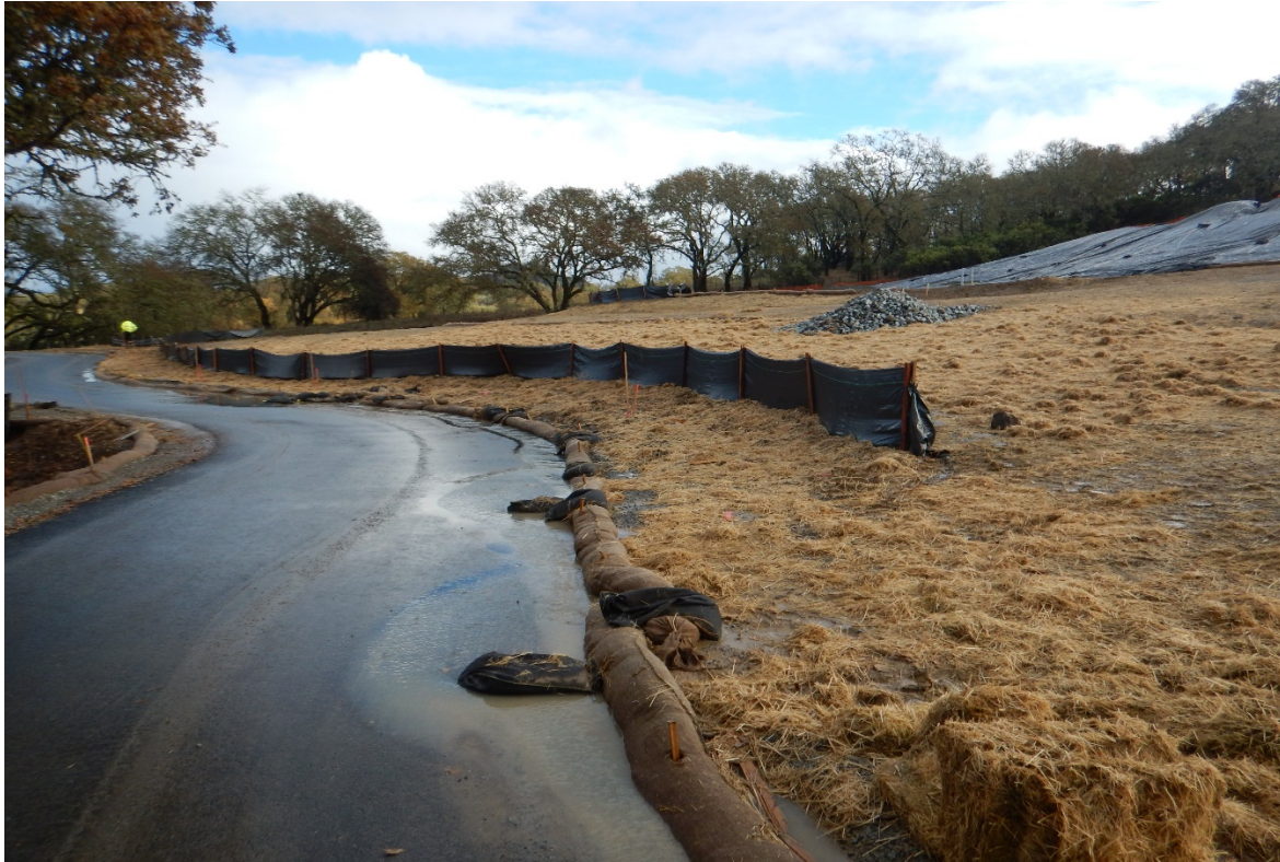
Picture 11 above. Resort Area. Good example of redundant BMPs. Even with this level of protection turbid runoff is still observed.
