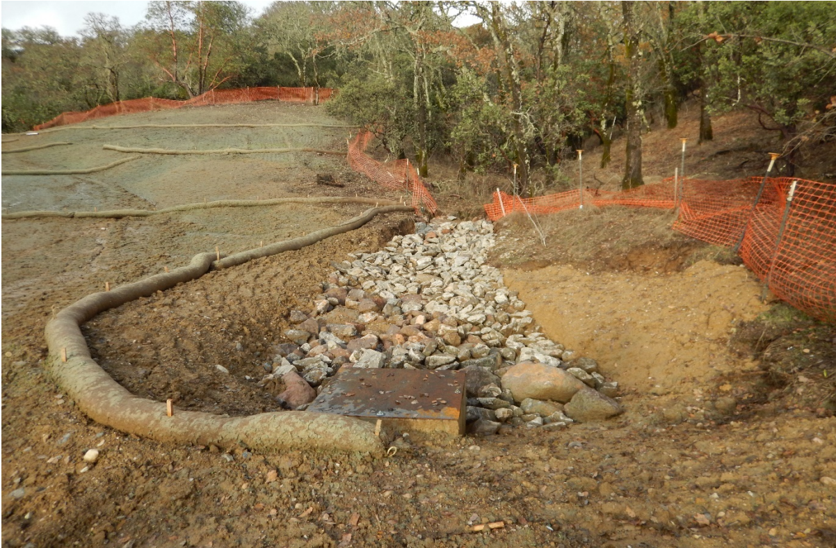
Picture 37 above. Road 8. BMPs present yet there are signs of erosion and sedimentation.
