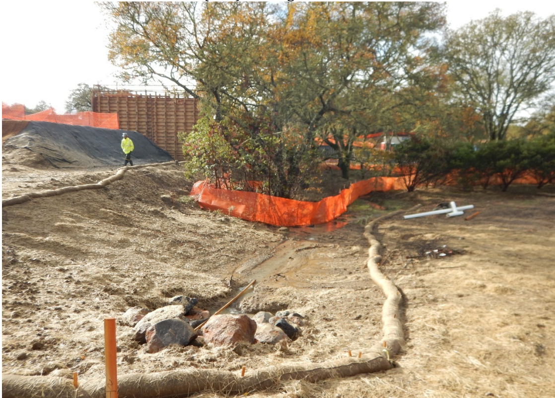
Picture 6 Above. Resort Area. Image show erosion and sediment controls with ESA fencing. BMP maintenance and housekeeping is needed. Some erosion and siltation and noted.
