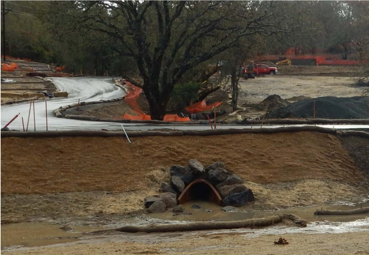
Picture 15 above. Resort Area. Erosion controls need maintenance. No sediment controls.
