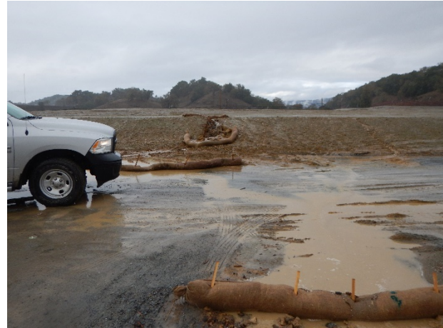
Pictures 3a (left) and 3b (right) above are from the lower Site construction trailer. BMPs are overwhelmed and turbid discharges from this area flow toward the City of Healdsburg detention basin.
