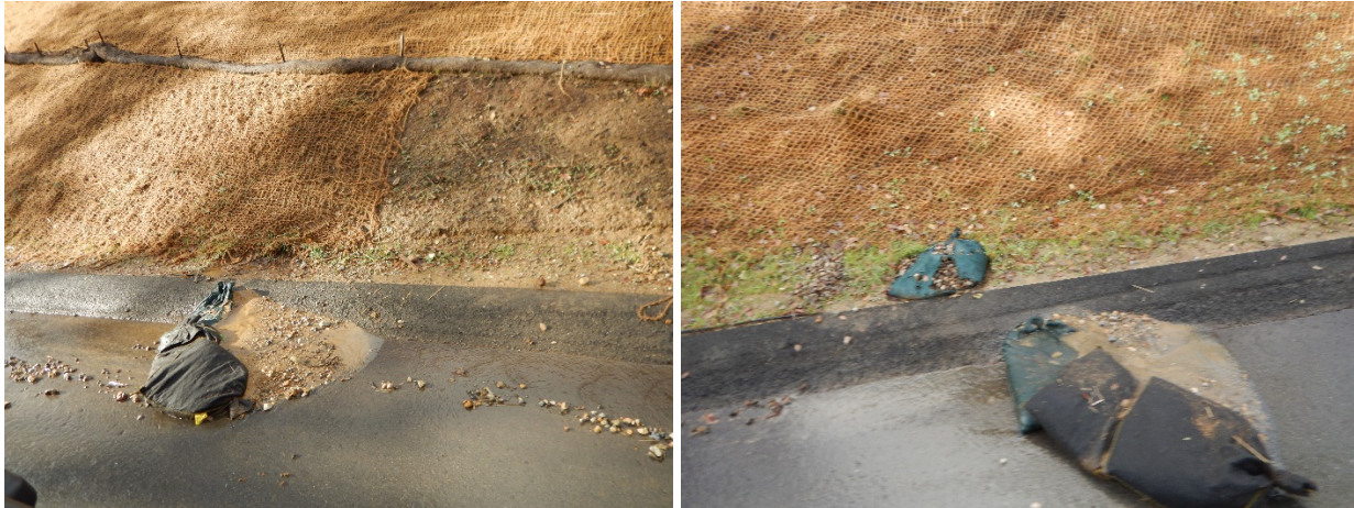
Pictures 33a (left) & 33b (right) above. Shannon Road. BMPs overwhelmed and in need of maintenance.
