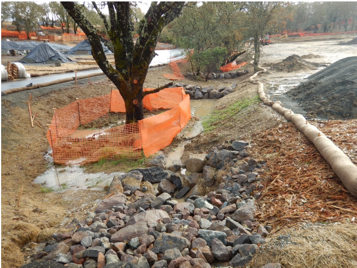
Picture 8 above. Resort Area. Shows waters of the state. While BMPs are present maintenance is needed and some stockpiles are placed near the top of bank and are uncovered. Additionally, bark, slash and woodchips are placed where they may wash into waters of the state.
