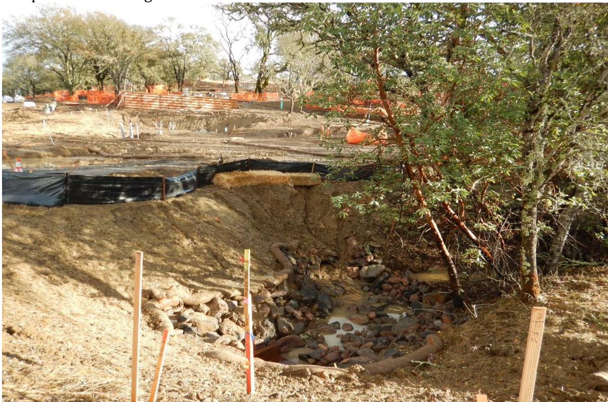
Picture 28 above. Resort Area. Inadequate erosion and sediment controls. BMPs were compromised leading to bank erosion. Culvert full of sediment.
