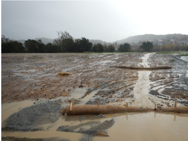
Pictures 3a (left) and 3b (right) above are from the lower Site construction trailer. BMPs are overwhelmed and turbid discharges from this area flow toward the City of Healdsburg detention basin.
