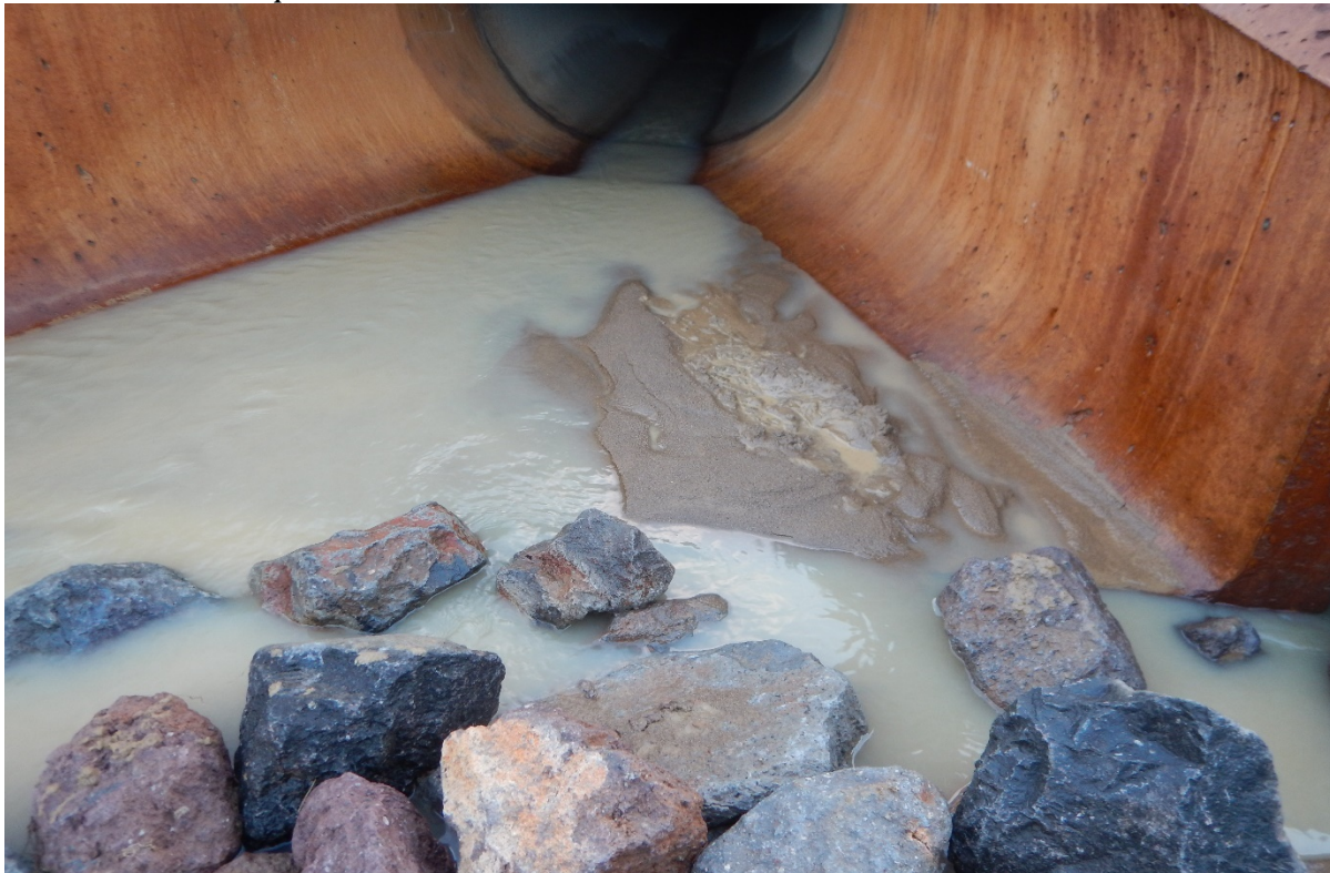
Picture 62 above. Shannon Road. Fine sediment deposition of the same composition (silty sand) as compared to sediment discharging from Road 5 and Road 8.
