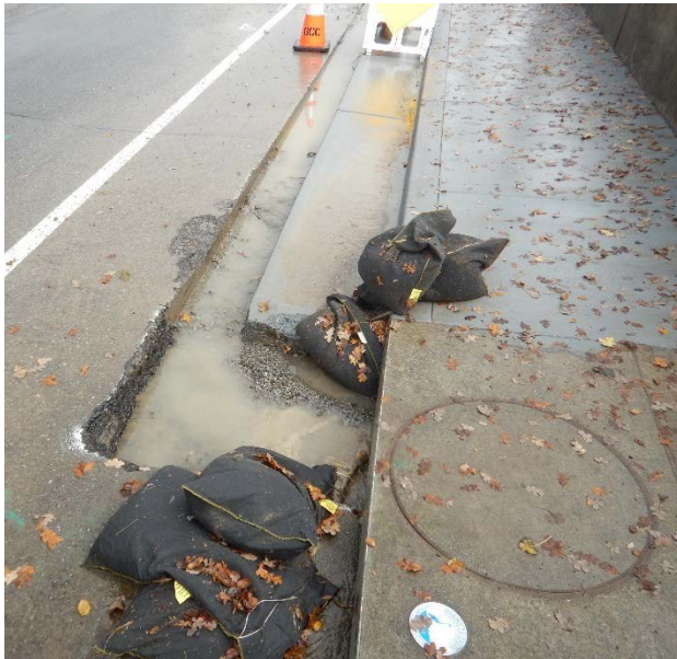
Pictures 2a and 2b above. Pic 2a (left) shows a turbid discharge from construction Site entrance along Healdsburg Avenue. Pic 2b shows Regional Water Board sampling the turbid storm water discharge from the project entrance (367 NTU). Additionally, a background storm water sample was collected from Healdsburg Ave (72.7 NTU).
