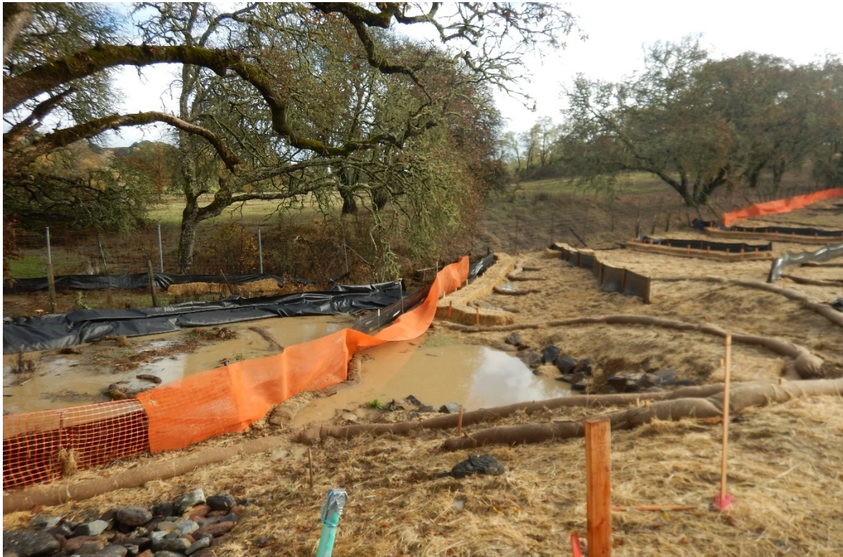
Picture 14 above. Resort Area. Downstream of sediment basin. Looking at downstream discharge location that leaves the Site. BMP maintenance is needed: many areas are overwhelmed by flows.
