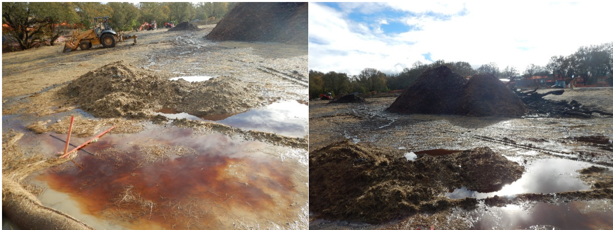
Picture 7a and 7b above. Resort Area. Images show tannins leaching from wood chips and mulch.
