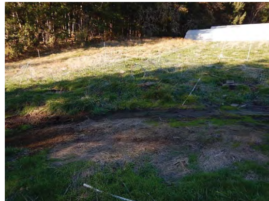
Figure 11. Road at the base of the wetland, leading to the other upper greenhouse area. The road is saturated and rutting, and I observed potting soil spread over the surface.
