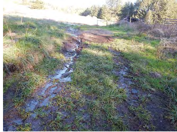
Figure 9 Road at the base of the wetland, leading to the other upper greenhouse area. The road is saturated and rutting, and I observed potting soil spread over the surface.
