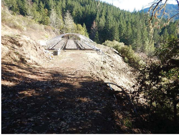
Figure 20. WQ-8 with erosion, transport, and delivery of sediment and cultivation-related potting soil to watercourses from both ends of the 0.11 acre flat. The greenhouse is oriented approximately east-west.
