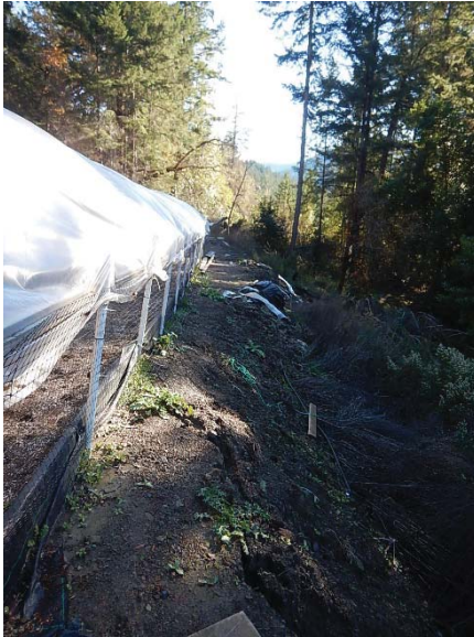
Figure 4. At WQ-1, a flat was developed for cannabis cultivation by grading and side casting spoils; the side cast exhibits cracks and threatens to deliver sediment. Cultivation waste, potting soil, and plastic waste is pushed over the side cast fill slope toward a Class II watercourse creating a condition of threatened delivery of waste to surface water.
