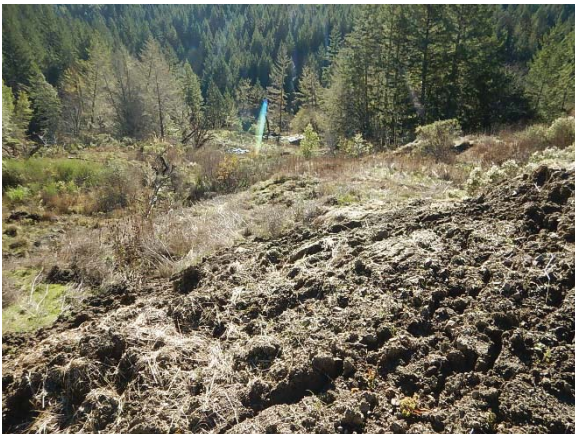
Figure 27. At WQ-7, the flat is constructed with the edge of the fill pushed within 20 feet of a class II watercourse associated with the slide.
