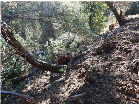
Figure 16. WQ-3. Freshly side-cast fill placed on already sweeping trees at WQ-3.
