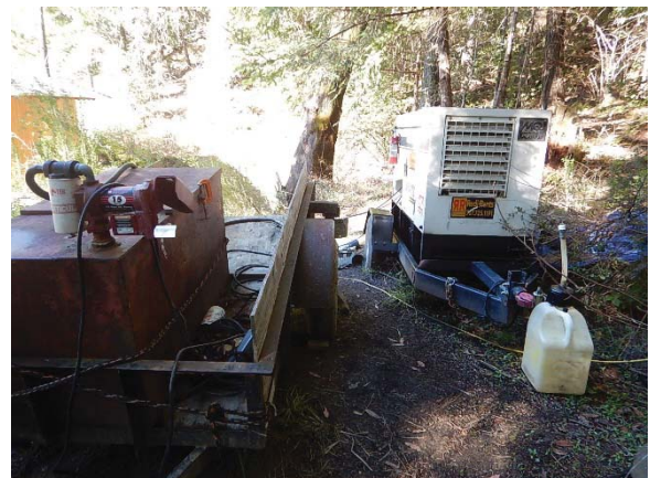
Figure 8. Generator and fuel tank located on property near the structure.
