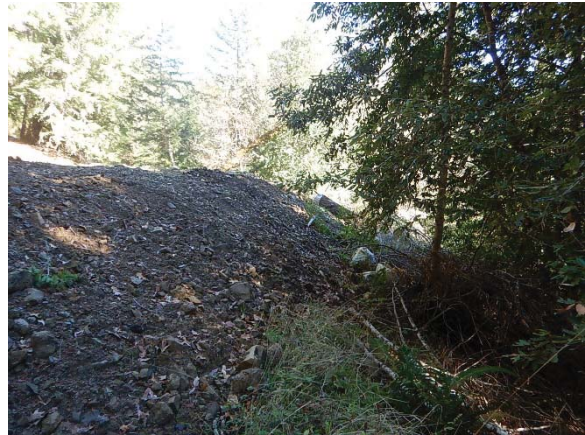
Figure 18. Loose, side-cast fill at WQ-3
