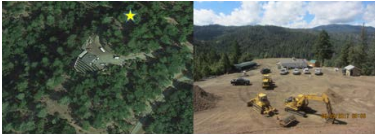
Figure 6: The left photo is aerial imagery of the Property prior to significant development (Google Earth Pro, 2017). The yellow star indicates the approximate location where I was standing when I took the photo on the right, looking southward toward the house located on APN 025-350-53-00 (IMG_4129 S. Feiler).
