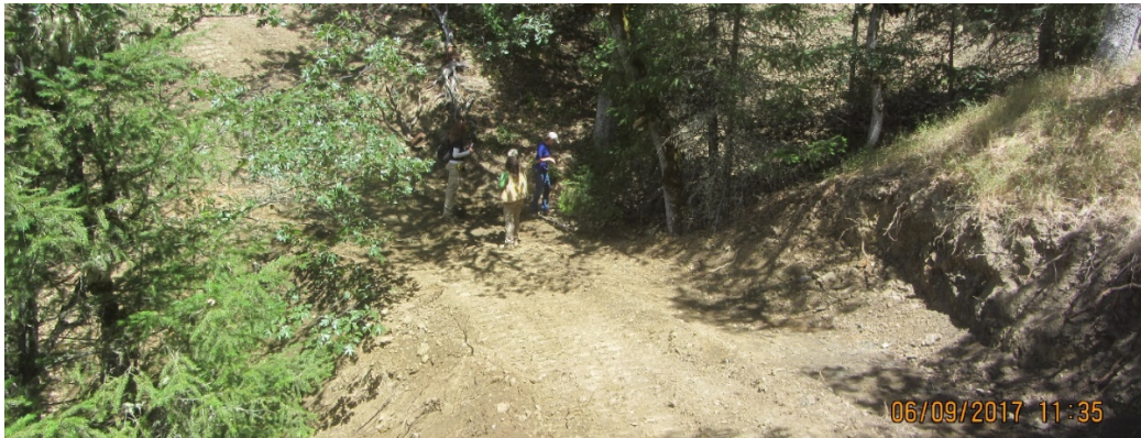
Figure 19: Overview of road at the base of the filled canyon, crossing a Class III watercourse channel (IMG_4233_4234 S. Feiler) (Edited by Luders, J.).
