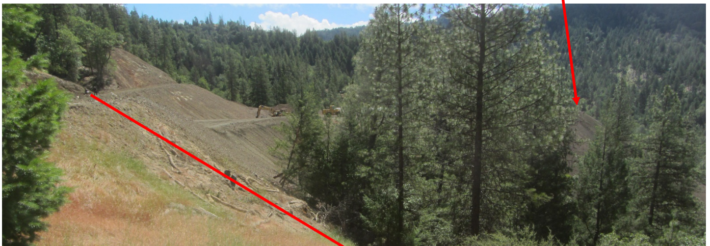
Figure 16: The red line shows the approximate alignment of the stream that was excavated and buried during construction. Earthen spoils in front of the home are partially visible through the trees (IMG_4164_4165 S. Feiler) (Cropped and edited by Luders, J.).
