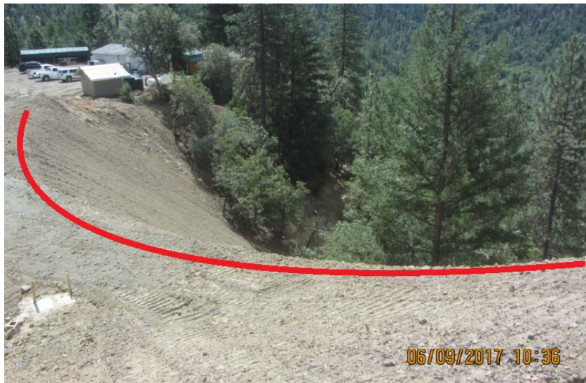
Figure 17: The red line outlines the approximate contour of the filled canyon. The upper edge of this over steepened slope terminates with an abrupt shelf. Staff measured slopes on the fill face at 75%-80% (IMG_4181 S. Feiler) (Cropped and edited by Luders, J.).
