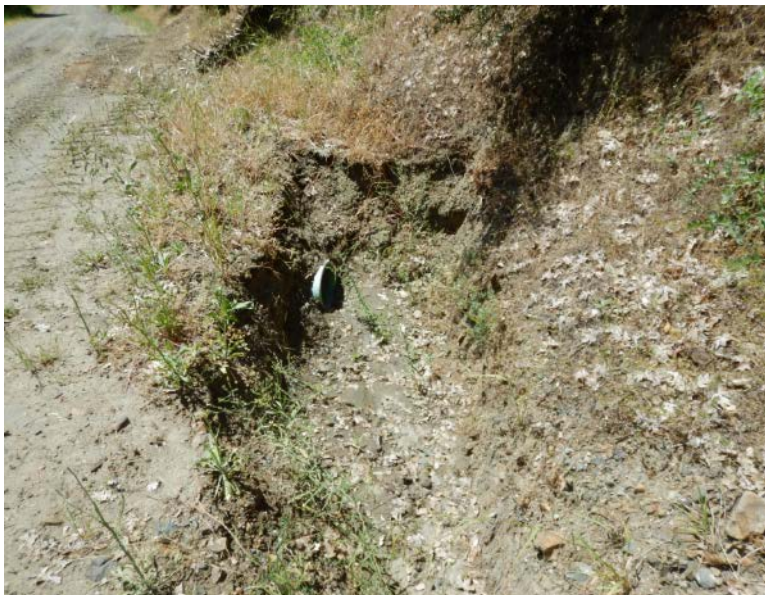
Figure 25: Inlet of the ditch relief culvert at WP-171 (IMG_4211 S. Feiler).
