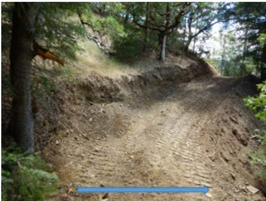
Figure 20: Blue line shows the approximate alignment of the watercourse channel filled in and crossed by the roadway. Viewed from WP-175 (DSCN1296 Luders, J.) (Edited by Luders, J.).
