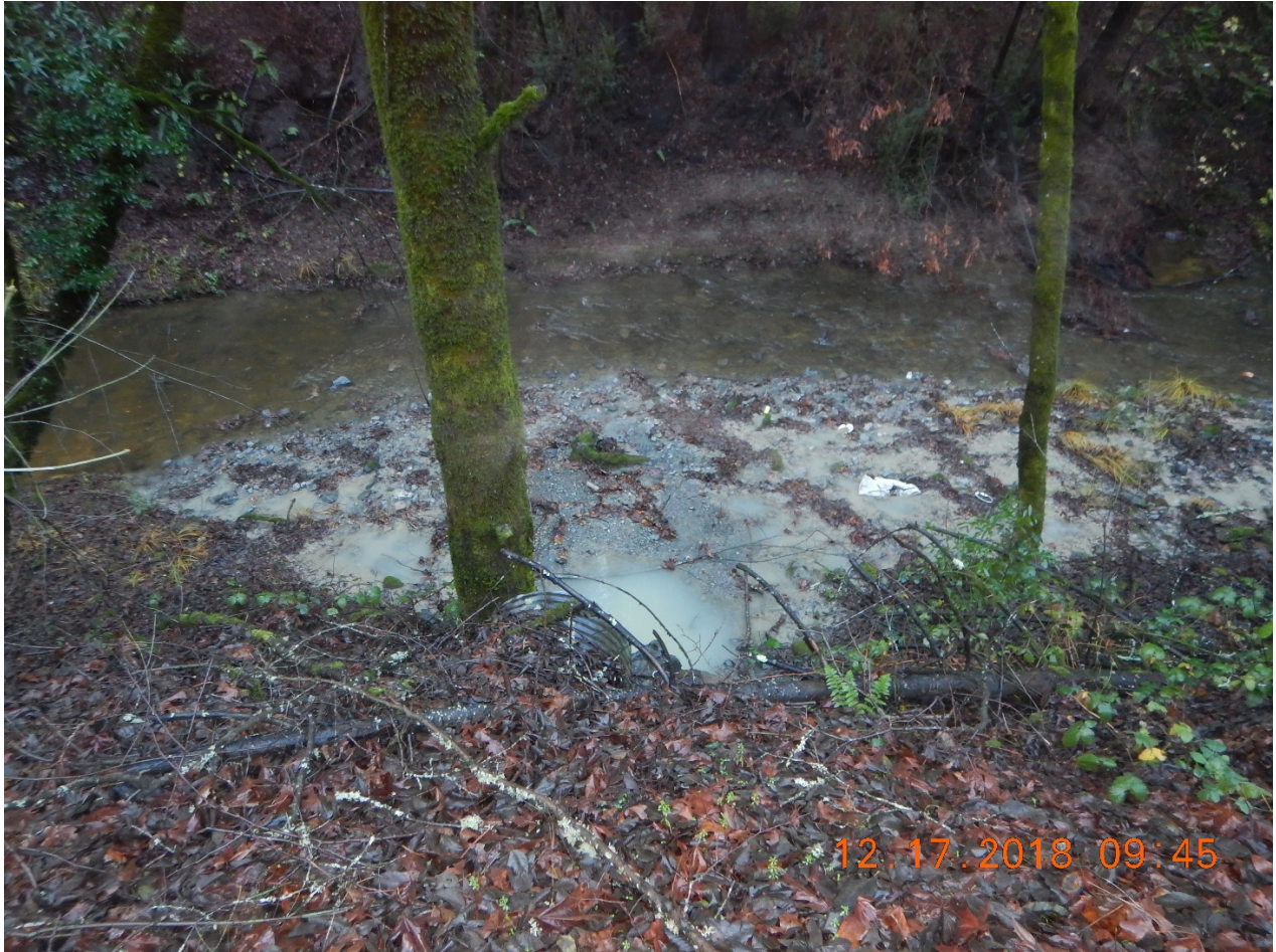
Photo 3: Eastern outfall from Mark West Quarry to Porter Creek showing turbid water in pool below pipe. Photograph taken by Paul Nelson.
