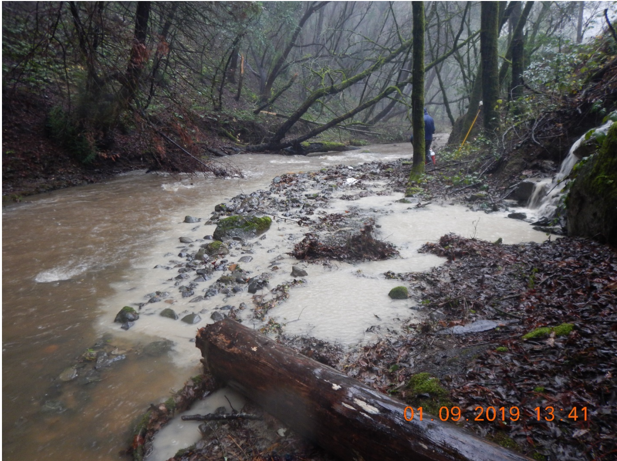
Photo 3: East culvert discharge to Porter Creek looking downstream (west). Note mixing zone at left side of photograph. Photographed by Josh Luders.
