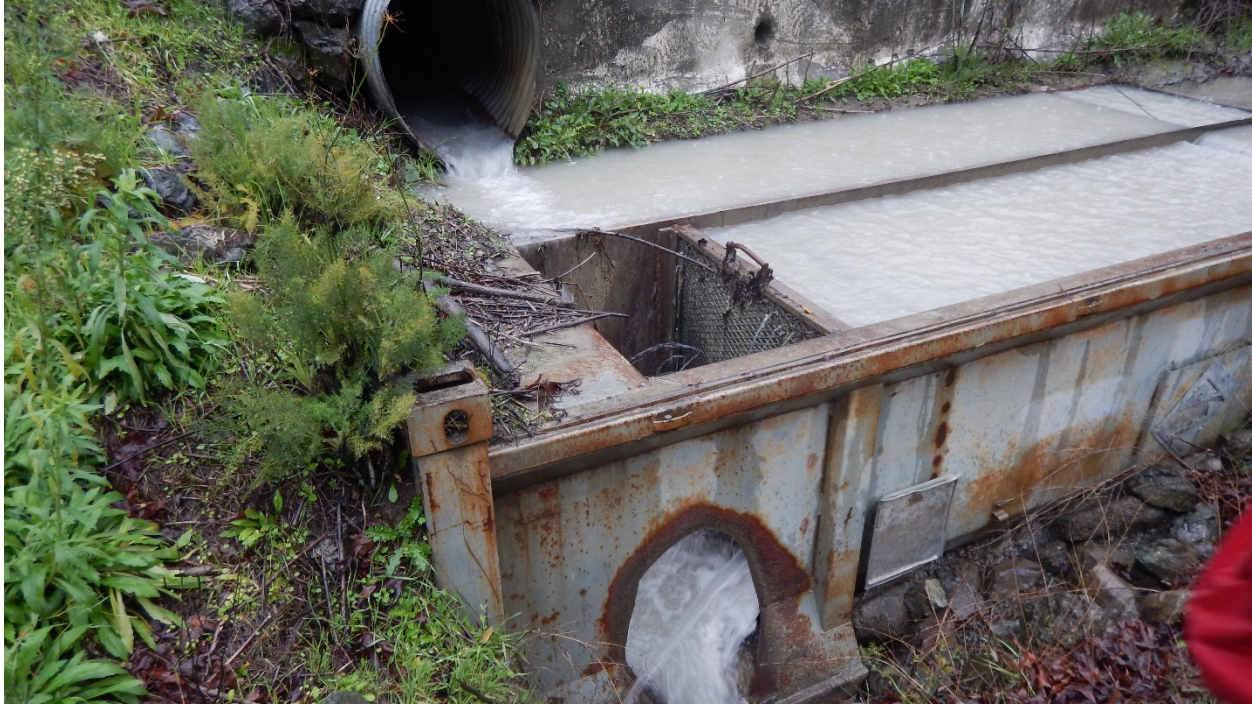
Photo 4: View of west culvert (CULVERT W) and settling structure. Turbid water evident in outfall and confirmed by turbidity results. Photographed by Paul Nelson.
