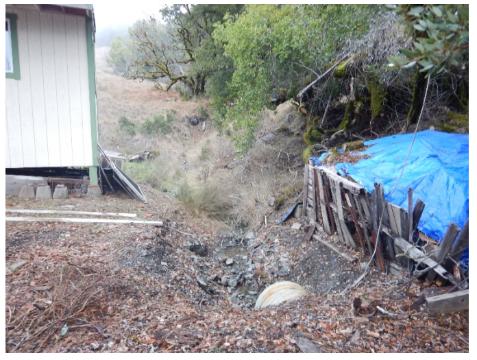
Photo 30: Stream crossing C5 located next to residence (DSCN4372)
