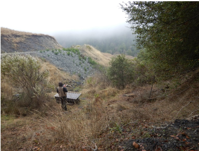
Photo 23: Fill from the road that had been sidecast into the pond's eastern Class III watercourse and adjacent to the well (DSCN4370)
