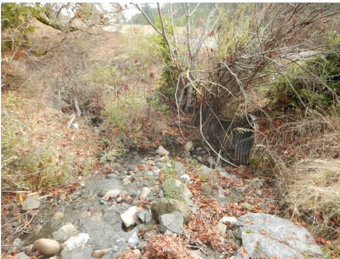
Photo 27: Stream crossing C1 at Briceland Thorne Road (DSCN4380)
