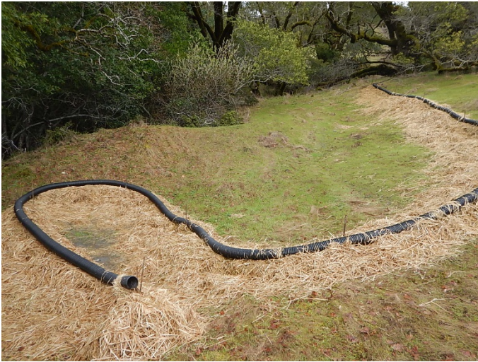
Photo 19: Siphon discharges to a bowl area that allows moderate pooling of water
