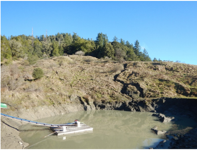
Photo 7: February 21, pond level after additional pumping (DSCN4430, photo taken February 21, 2019)
