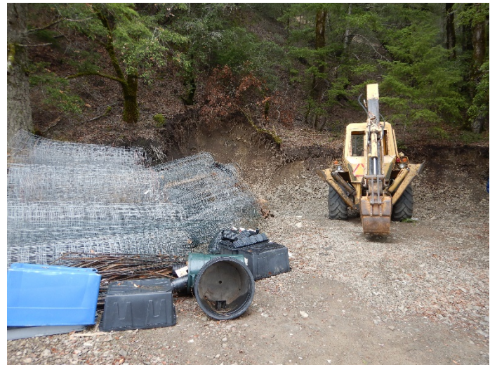
Photo 36: Backhoe located at the shop area (DSCN0150 photo taken by Sean Stout)
