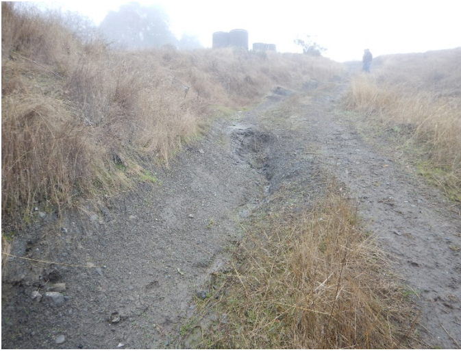
Photo 19: Ruts and rills in the road to CA2 (DSCN4289)
