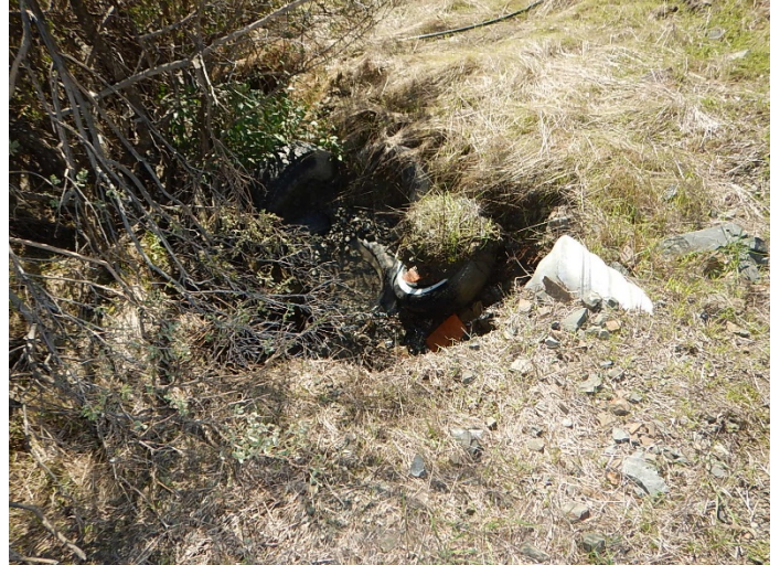
Photo 24: Stream crossing C4 with tires placed in the channel below the outlet (DSCN9382 photo taken by Adona White, February 18, 2019)
