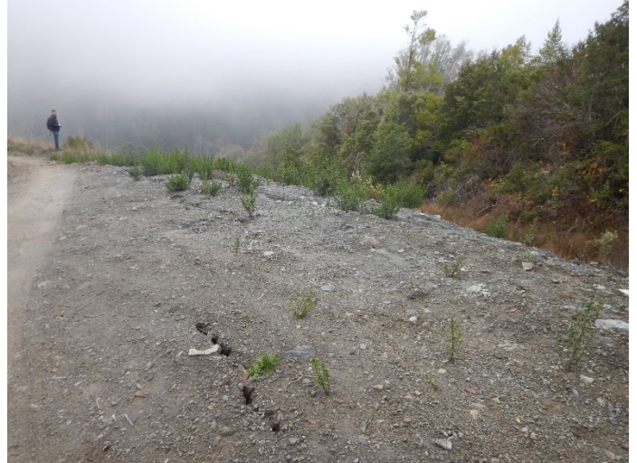
Photo 24: Cracks in fill above the eastern Class III watercourse (DSCN4364)
