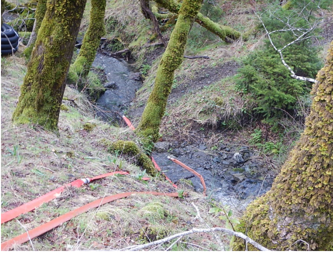
Photo 17: Discharge location of pumps in western Class II watercourse
