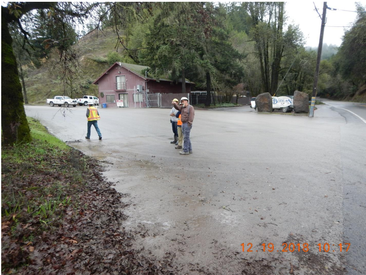
Photo 1 - View of quarry entrance at Highway 116. Note sediment on roadway (center right of photo) and drop inlet to stream at center left of photo. Photographed by Josh Luders.
