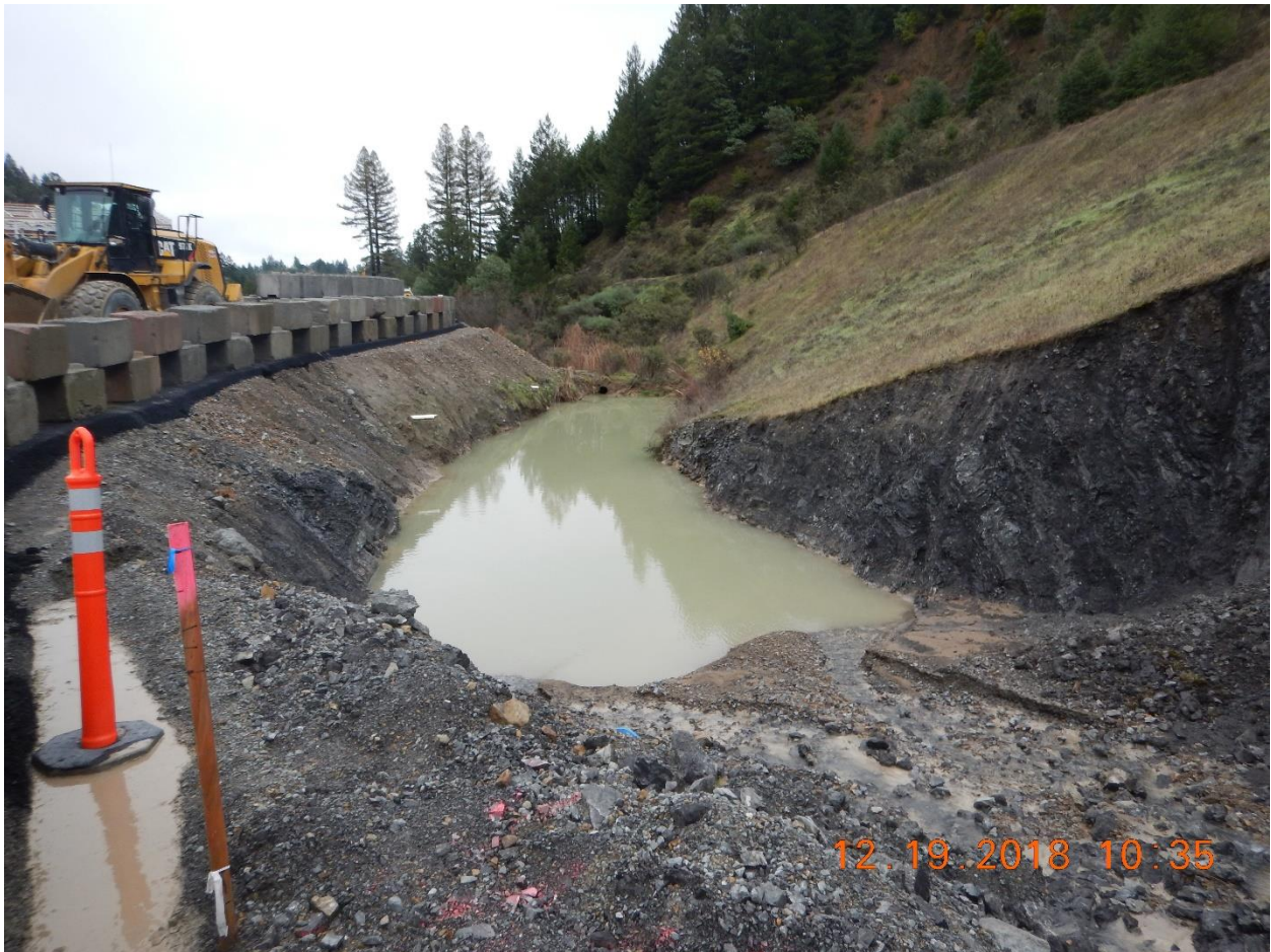
Photo 3 – View of eastern settling pond. Photographed by Josh Luders.
