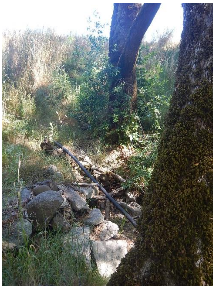
Figure 13. Embankment and dewatered section of watercourse at road crossing.
