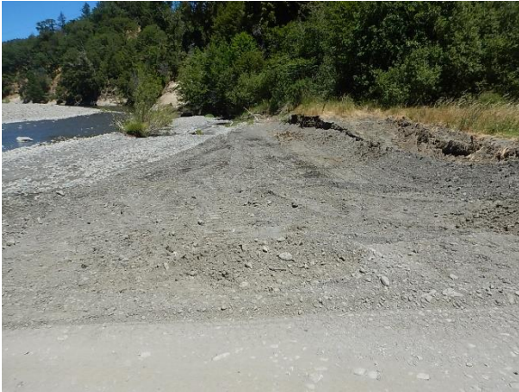
Figure 23. Terrace mined for embankment material.
