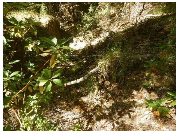
Figure 16. Bank erosion voids at spillway discharge point on Class II bank.
