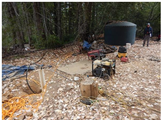
Photo 8: Well, W1, generators adjacent with no containment and refuse strewn about
