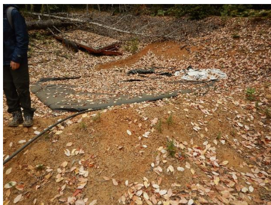
Photo 7: Bladder, B1, no secondary containment
