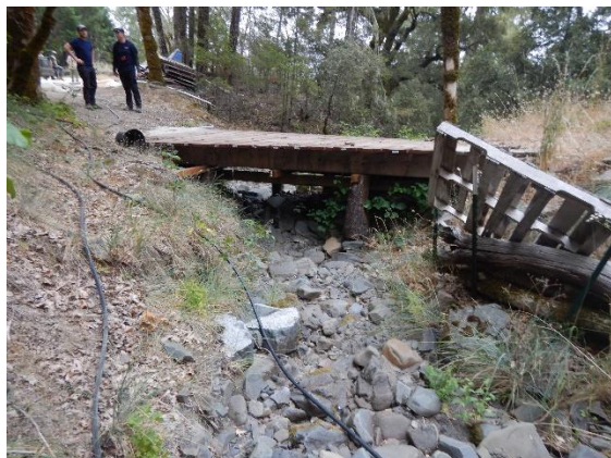
Photo 9: Bridge crossing, C1
