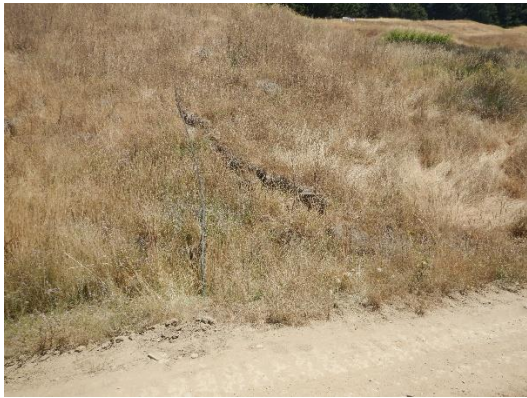
Photo 10: Hillside above DRC1, plastic polypipe leads into and through the crossing.
