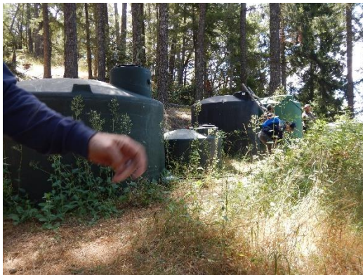
Photo 5: Water Storage tanks on a hillside, adjacent to MT1
