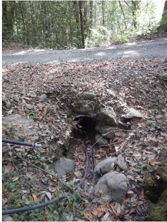
Photo 10: Inlet of C2
