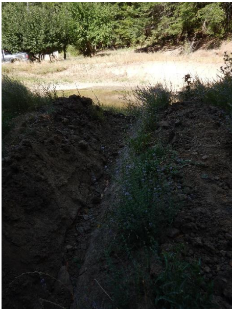
Photo 6: Spillway of P1
