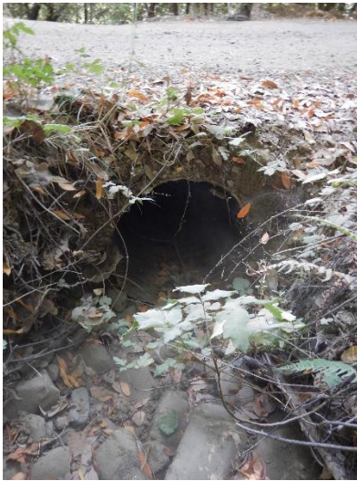
Photo 12: Inlet of C3
