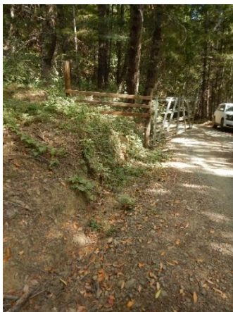
Photo 9: Inboard ditch carrying CIII channel conveyance from C1 diversion point
