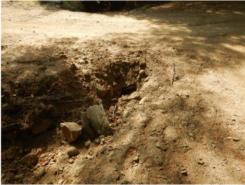
Photo 18: Buried inlet of C4
