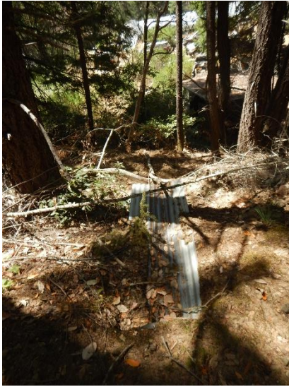
Photo 7: Outlet of DRC1
