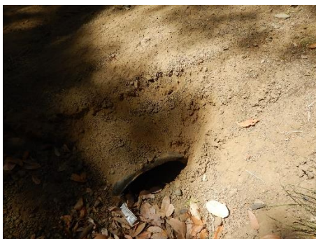
Photo 6: partially filled inlet of DRC1
