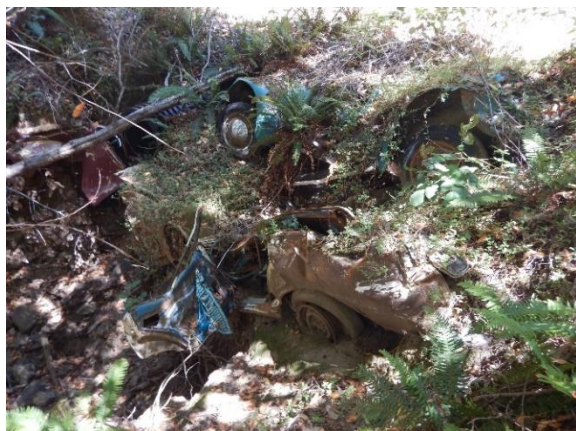
Picture 12: Outlet of C1, cars used to stabilize the fill
