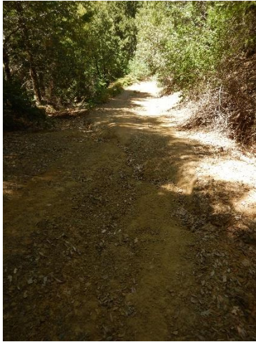
Photo 4: Rutting from inboard ditch crossing road, delivering to a class III watercourse.
