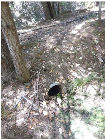
Picture 9: Inlet of outlet of P1
