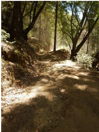
Photo 5: Rutting from poorly drained road
