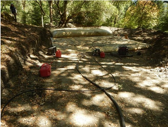
Figure 13. Cut made for the pad constructed for bladders.
