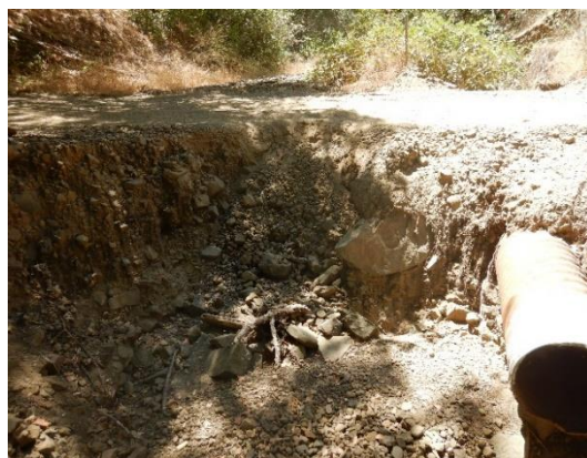
Photo 8 – Watercourse crossing and discharging sediment into the watercourse.
