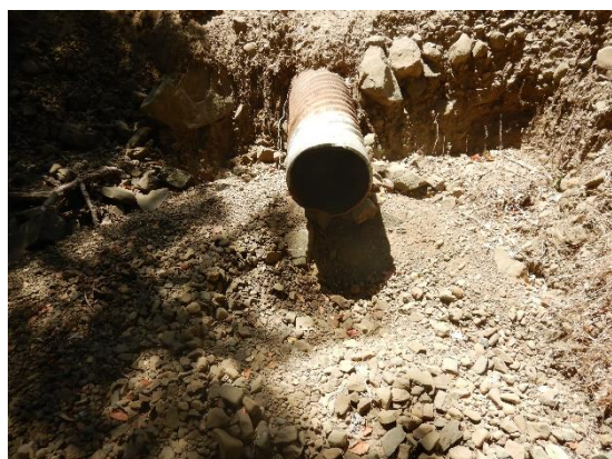
Photo 9 – Undersized shotgun culvert with road fill discharged into the watercourse.
