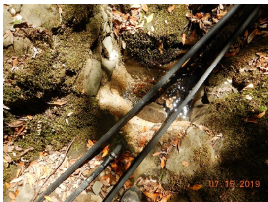
Photo 14 – Point of diversion from a watercourse providing water for cultivation on the parcel.
