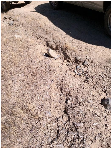
Photo 1 – Rill erosion on access road to property.
