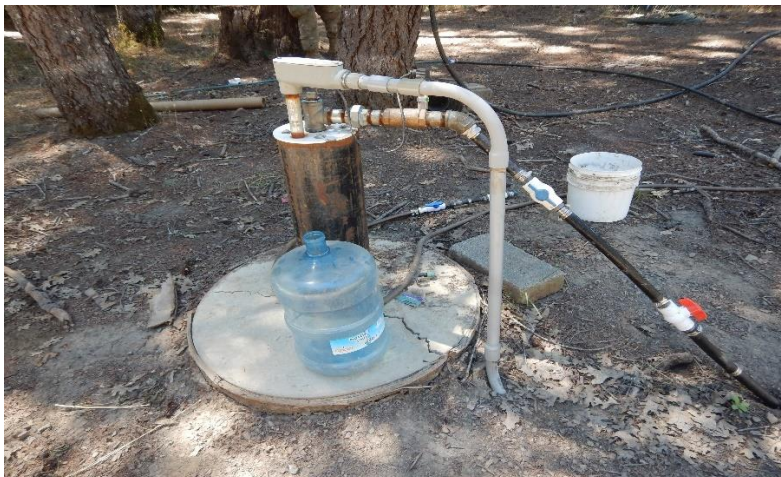
Photo 14: Groundwater well at inspection point W1
