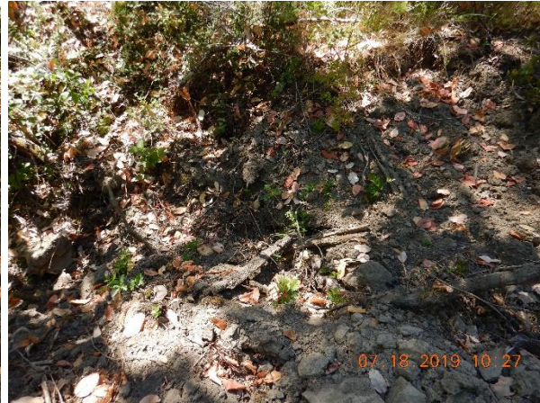
Photo 17 – Sediment in Class 3 (Crossing 2)
