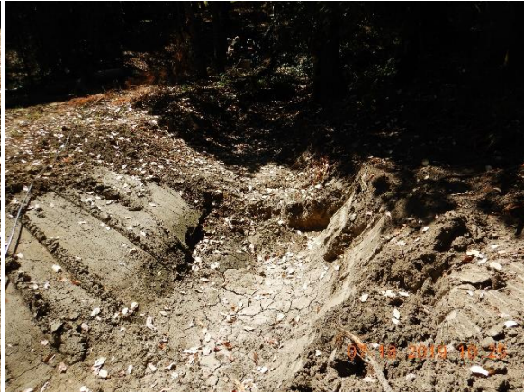
Photo 11 – Fill in crossing (Crossing 2)
