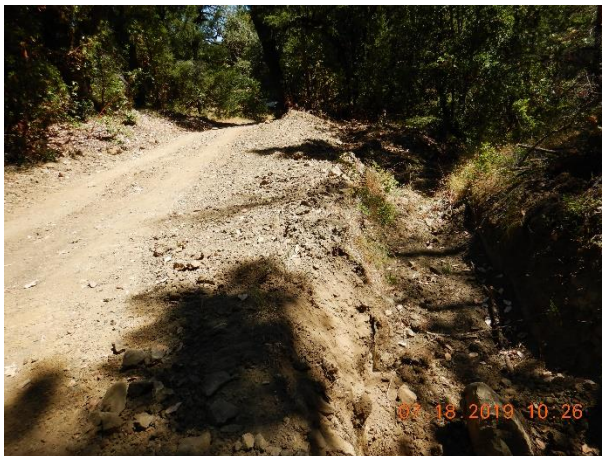
Photo 12 – Sediment from road work in ditch
