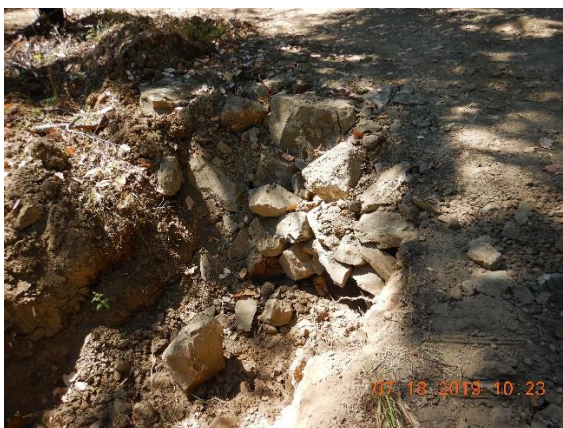
Photo 8 – road fill in crossing (Crossing 2)
