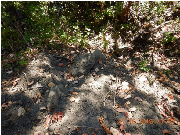
Photo 16 – Sediment in Class 3 (Crossing 2)
