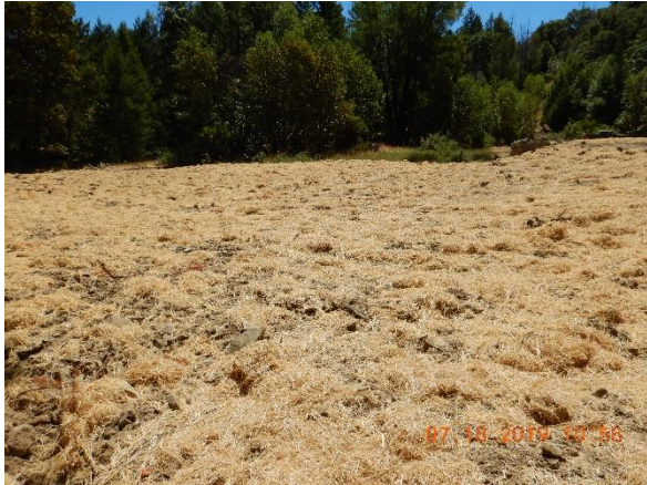
Photo 40 –Disturbed area with straw BMP
