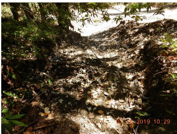
Photo 20 – Sediment in Class 3 (Crossing 2)
