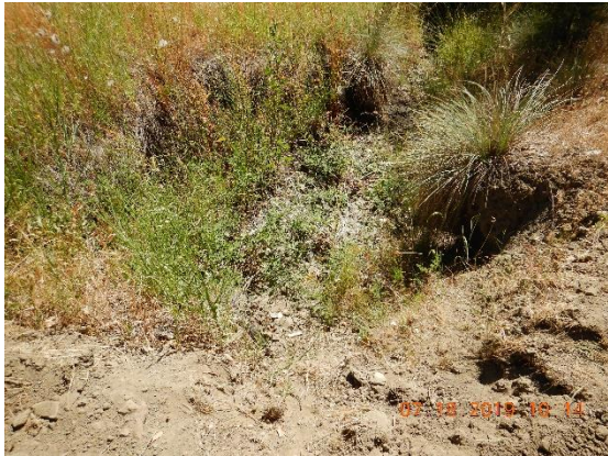
Photo 6 – Sediment in Crossing 1
