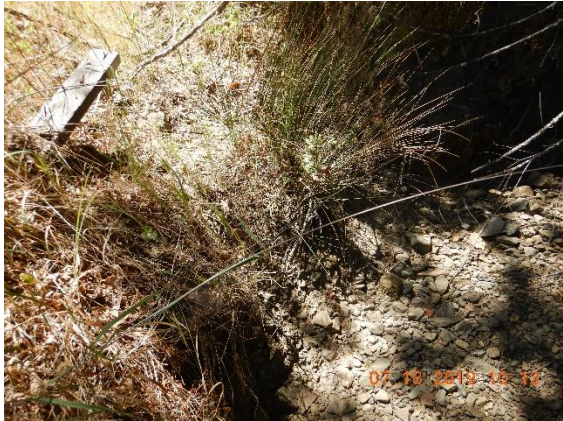
Photo 4 –Sediment in Crossing 1
