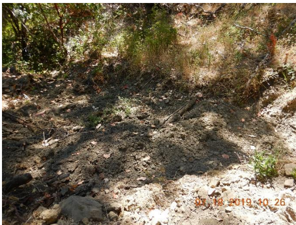
Photo 14 – Sediment in Class 3 (Crossing 2)
