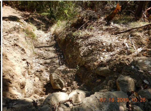
Photo 13 – Fill in crossing (Crossing 2)
