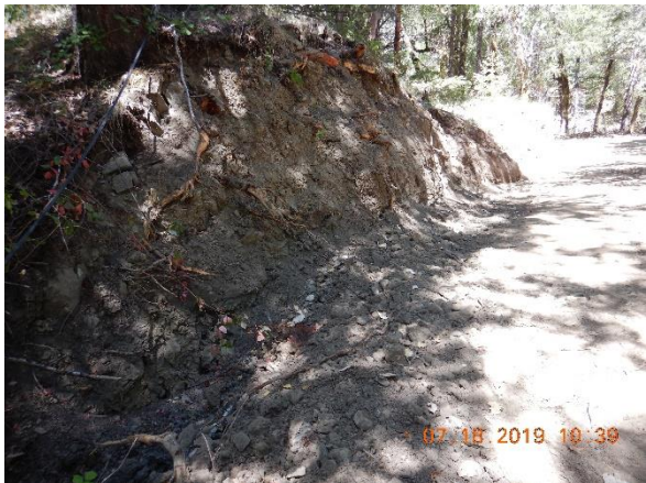
Photo 30 –Erosion from steep unstable cuts Photo 31 – Class 3 watercourse (Crossing 5)
