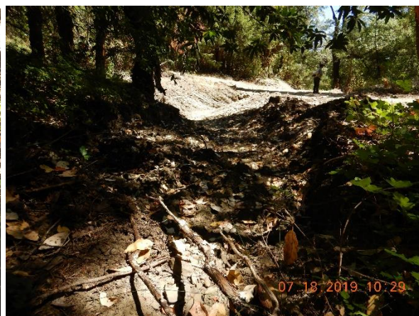
Photo 21 – Sediment in Class 3 (Crossing 2)
