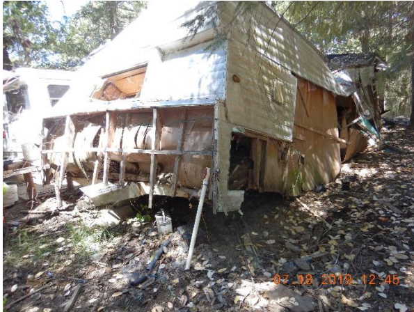
Photo 72 –Refuse and trailer falling apart adjacent to Class 2 watercourse (Figure 5)
