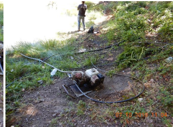
Photo 45- Pump and diversion pipes (pond edge)
