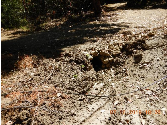
Photo 10 – Filled in crossing (Crossing 2)
