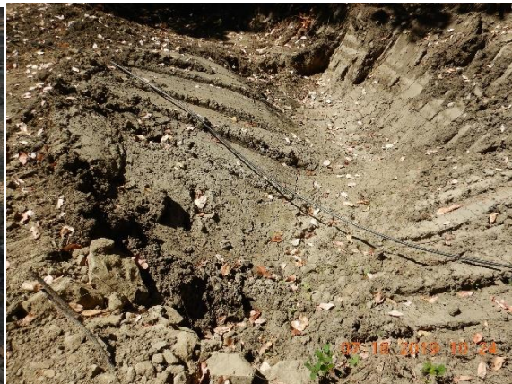
Photo 9 – Fill in crossing (Crossing 2)
