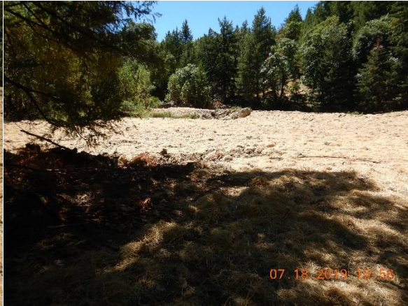
Photo 41 – Disturbed area with straw BMP
