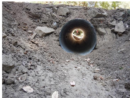
Photo – 13 Inlet view of culvert.
