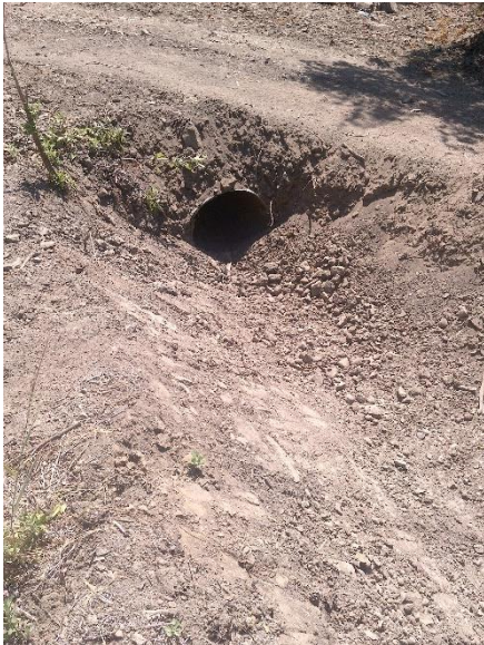
Photo – 20 Outlet of 3-foot culvert at inspection point 17.
