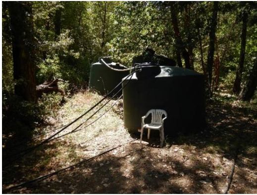
Photo – 5 Water storage tanks.
