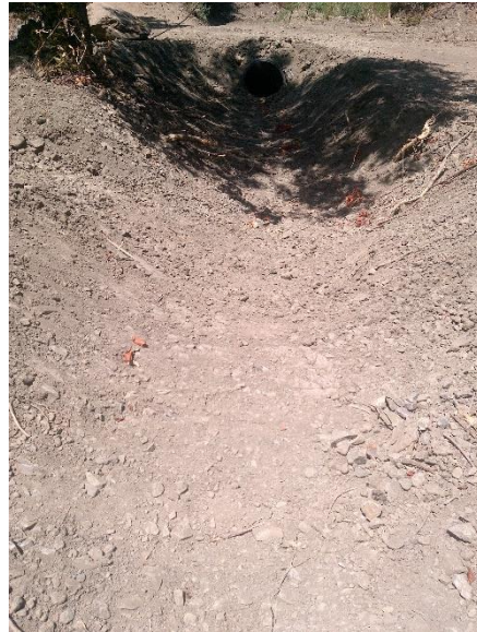
Photo – 21 Inlet of 3-foot culvert at inspection point 17.
