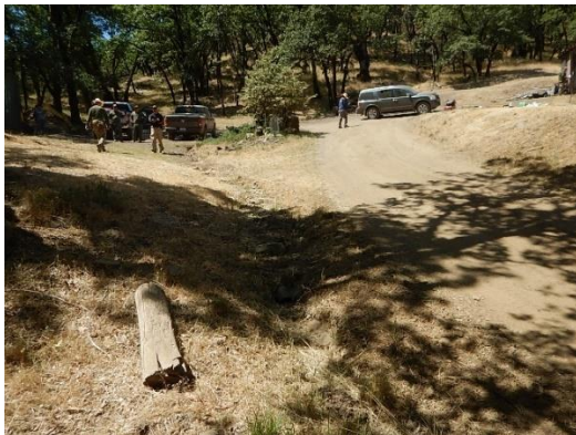
Figure 14. Class III, looking upstream to culvert outlet.
