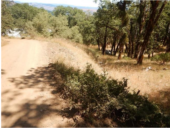
Figure 19. Road continues to impact Class III with side cast and surface erosion sediment delivery.
