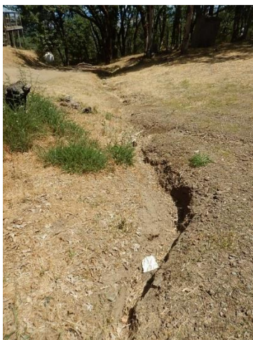
Figure 15. Looking downstream, gullied flow path on road surface from diverted Class III watercourse.
