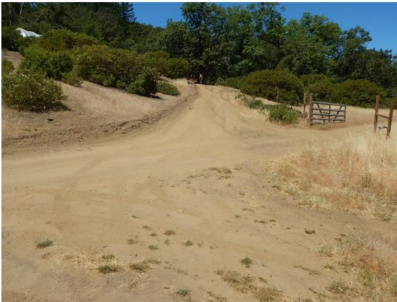
Figure 43. The road to CA4 intersects the main access road; runoff from the greenhouse has a flow path of approximately 230 feet to a channel head.
