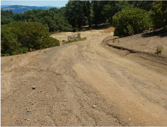
Figure 42. The road to CA4 intersects the main access road.
