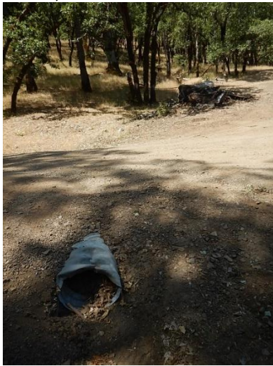
Figure 13. 20' long 12"-CUMP outlet for Class III watercourse.
