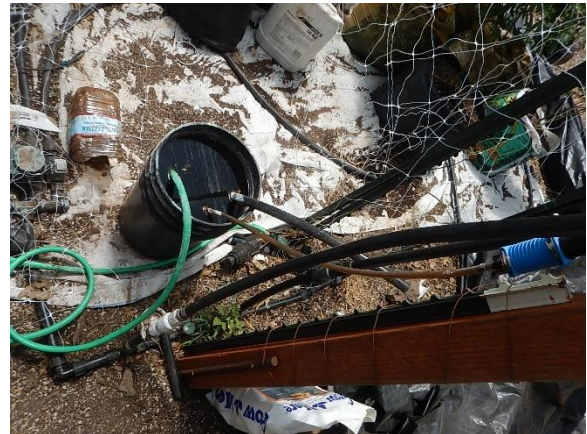
Figure 39. Fertilizers and mixing containers are on ground and the setup appears to readily allow for spills and overfills.
