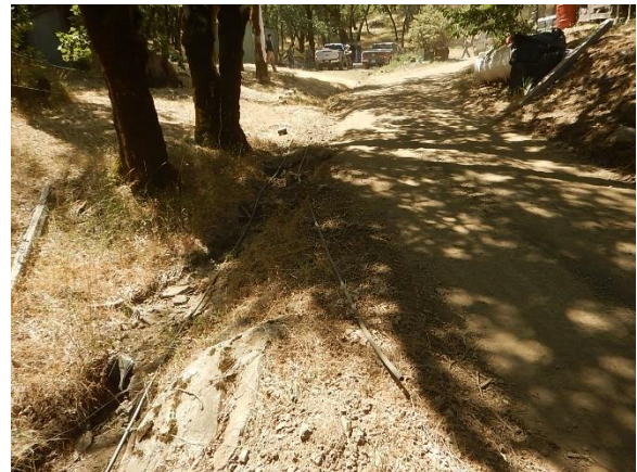
Figure 17. Class III runs along outboard ditch
