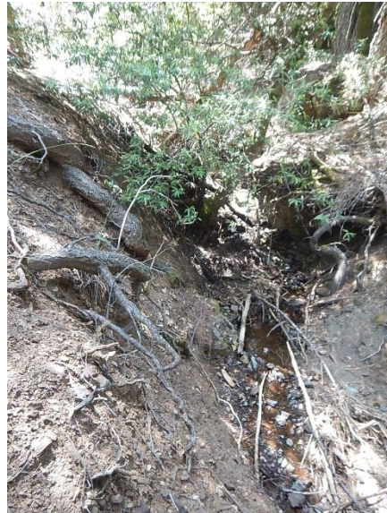
Figure 50. Watercourse below overflow pipe.
