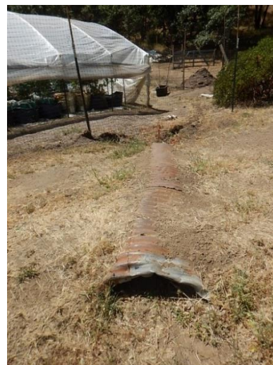
Figure 30. A 12" CMP is buried
