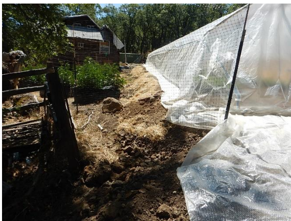
Figure 27. Grading of CA2 greenhouse pad.
