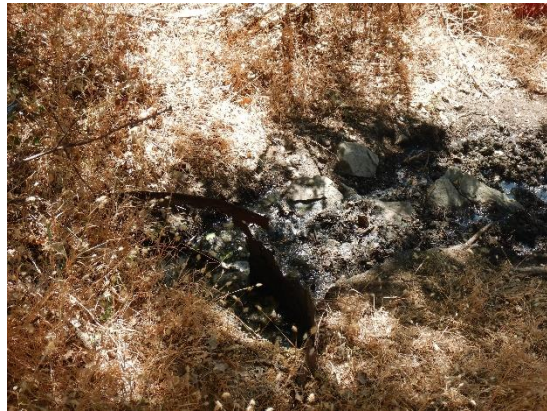
Photo – 9 Sewage outfall.
