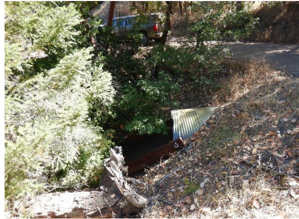
Photo 16 – Culvert outlet.
