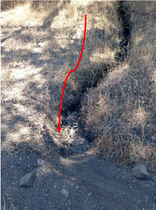
Photo 25 – Hillside erosion which produced channelization.
