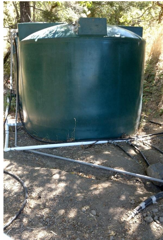
Photo 24 – Water storage tank area.
