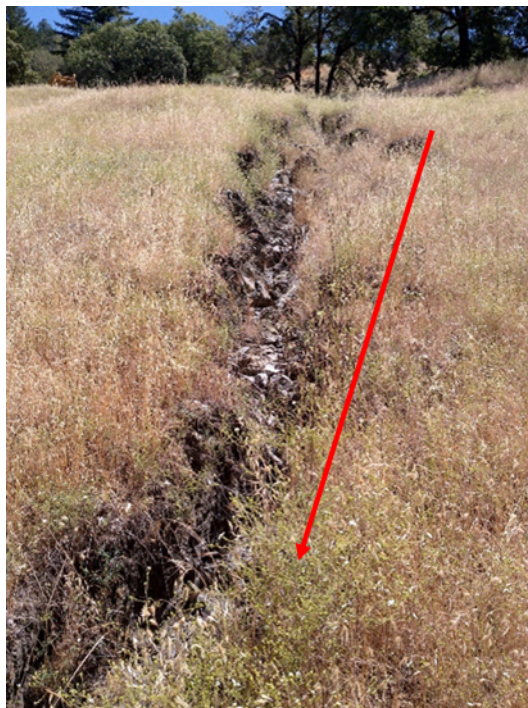
Photo 27 – Upstream view of erosion and channelization.
