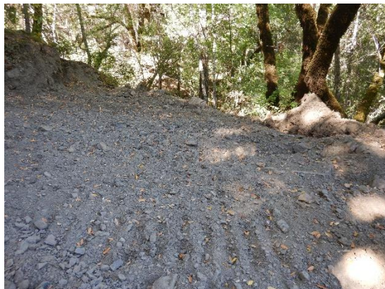
Photo 10 – Graded flat area along access road.
