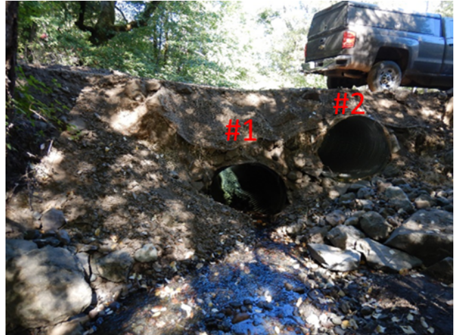
Photo 12 – Inlet view of double culverts and water crossing.
