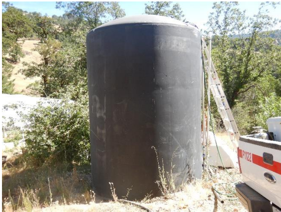
Photo 17 – Water storage tank.
