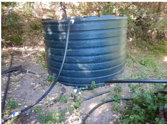
Photo 13 – Large water storage tank.
