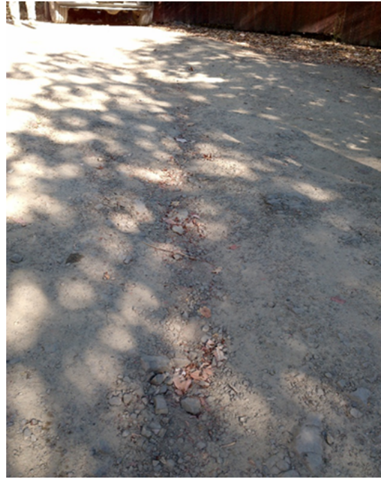
Photo 2 – Rilling on road behind entry gate.
