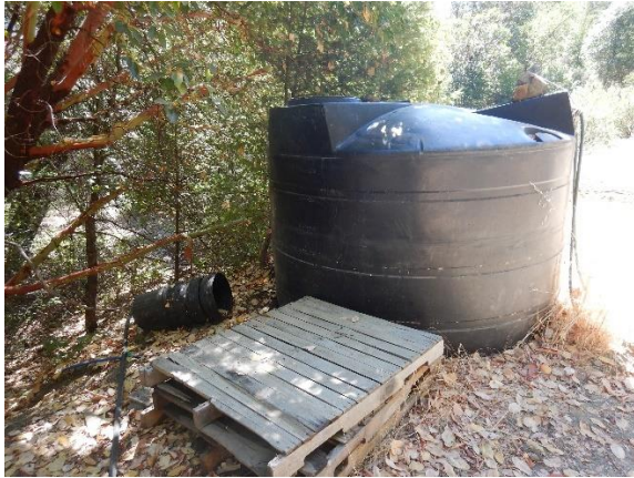
Photo 15 – Water storage tank.
