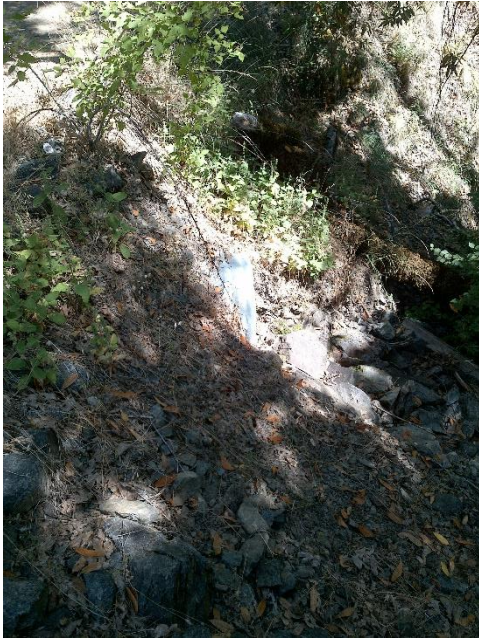
Photo – 17 Culvert outlet.
