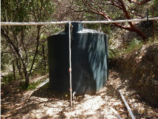
Photo 1 – Water tank storage.
