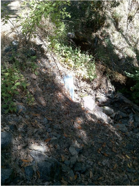
Photo – 17 Culvert outlet.
