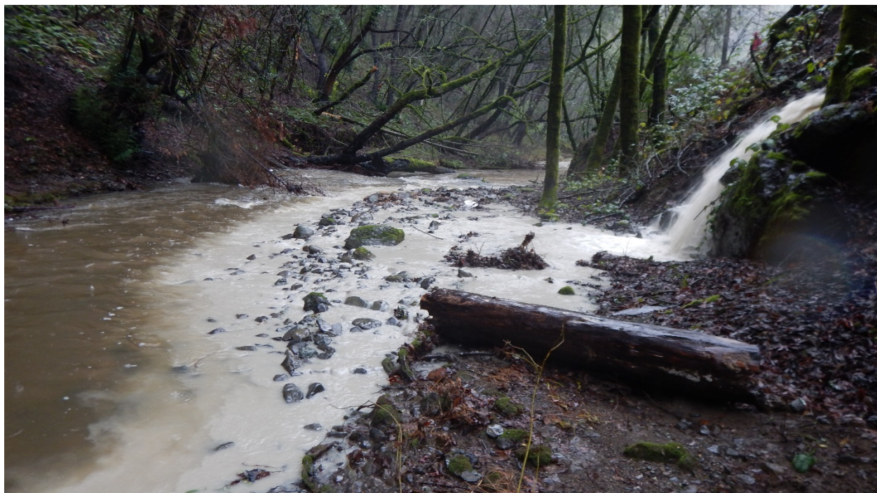
Photo 1: East culvert discharge to Porter Creek looking downstream (west). Note mixing zone at left side of photograph. Photographed by Paul Nelson.
