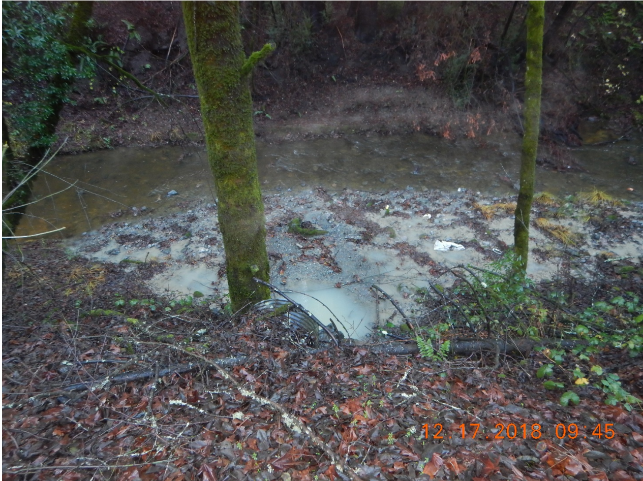
Photo 3: Eastern outfall from Mark West Quarry to Porter Creek showing turbid water in pool below pipe. Photograph taken by Paul Nelson.
