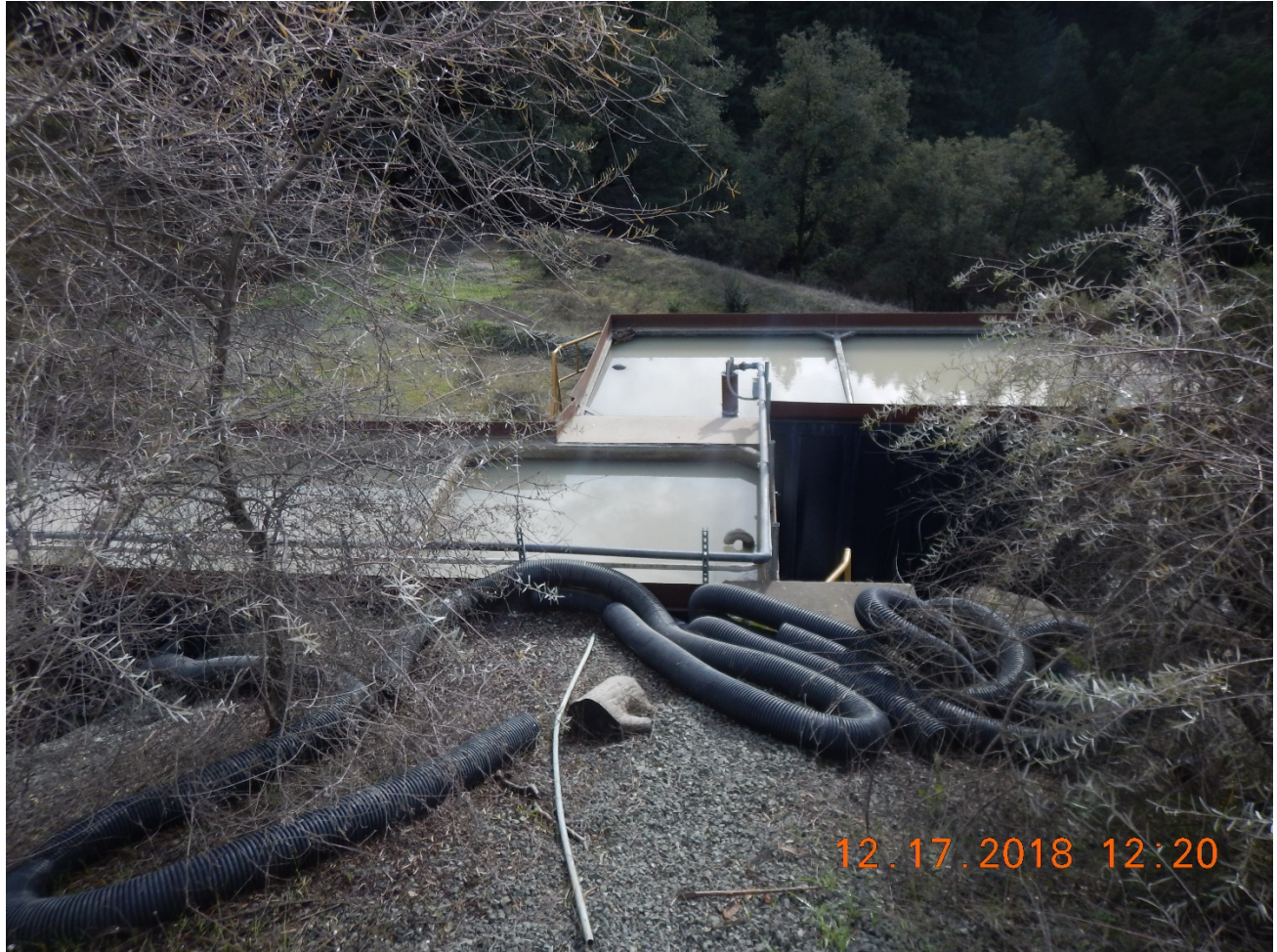
Photo 5: Photograph of settling tanks. Tank at upper right discharges to eastern outfall. Photograph taken by Paul Nelson.
