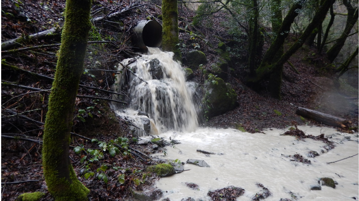
Photo 2: East culvert discharge to Porter Creek looking south from Porter Creek Road. Elevated sediment content is evident in the discharging water and confirmed by the analytical results. Photographed by Paul Nelson.
