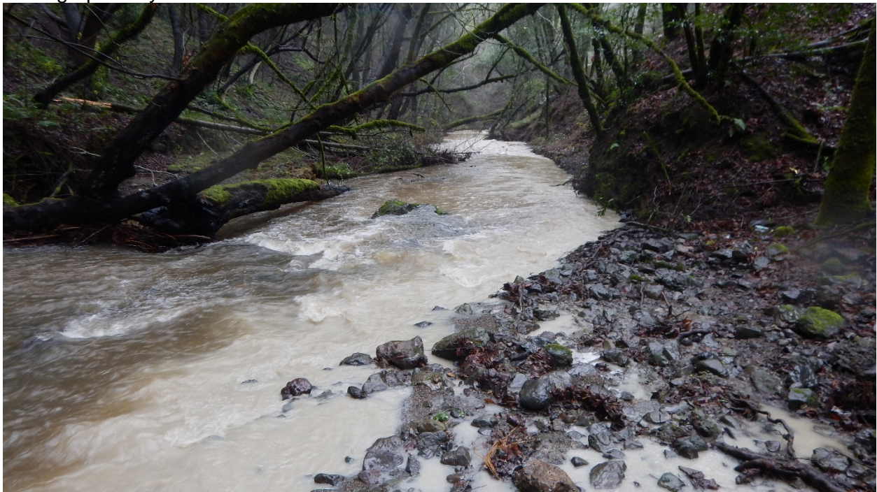
Photo 3: View downstream from east culvert (west). Turbid water mixing with streamflow. Photographed by Paul Nelson.
