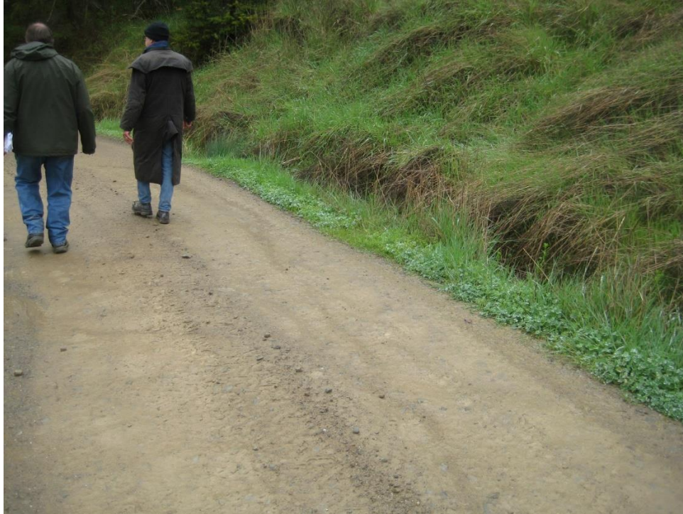
Photo 23. Road south of Site 2, spring flow runs into ditch.
