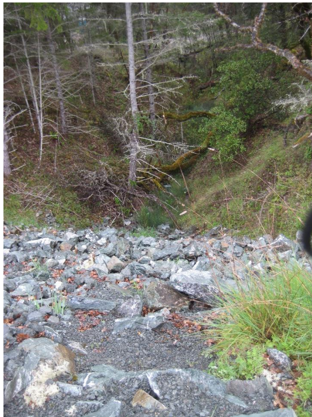
Photo 4. Looking northwest from top of spillway.
