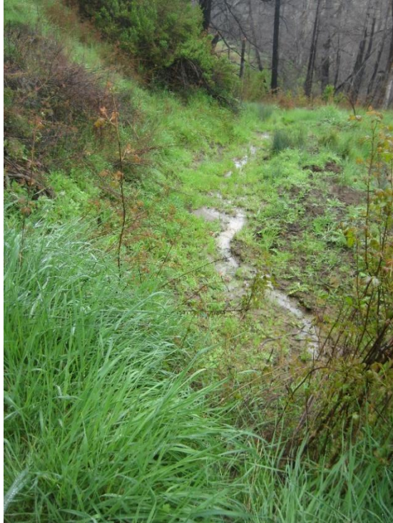
Photo 17. Site 2 downstream of plugged road crossing.
