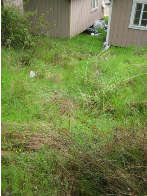
Photo 31. Site 4, water flowing past and underneath sheds.
