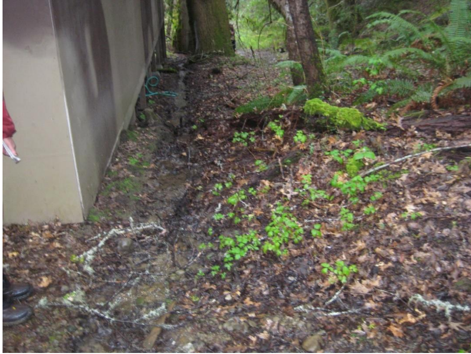
Photo 27. Water course directed along the side of building.
