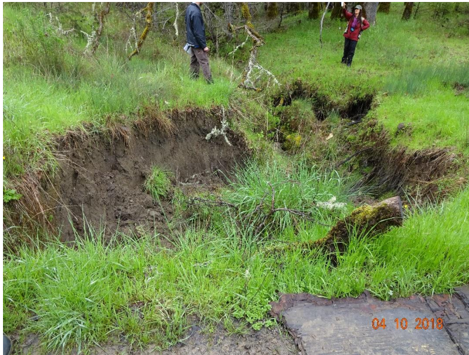
Photo 25. Road runoff and spring water is concentrated in incised gully.
