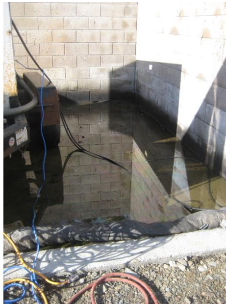
Photo 12. Generator building with no roof. Rainwater covered the floor of the building and is able to transport spilled hydrocarbons, identified by colorful sheen on water surface, outside of building.
