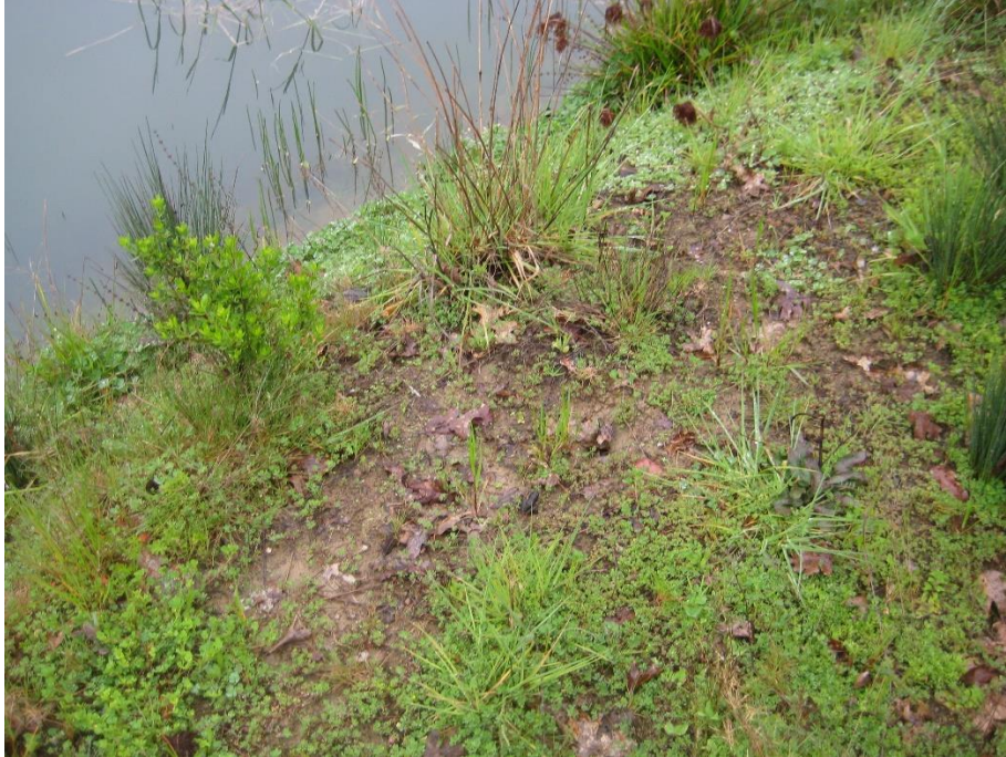
Photo 3. Picture showing water level in pond near dam crest.
