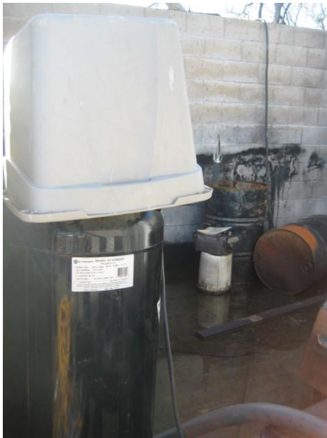
Photo 12. Generator building with no roof. Rainwater covered the floor of the building and is able to transport spilled hydrocarbons, identified by colorful sheen on water surface, outside of building.
