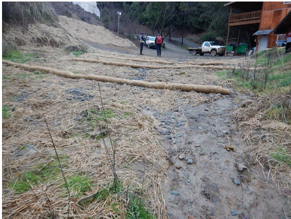
Figure 42. The residence is located in a bowl landform and road drainage from both north and south concentrate water between the cultivation area CAI, and fuels storage and the residence (WRPP site 42). The concentrated water extends downslope and has delivery to a Class III watercourse. Wattles were recently installed and have certainly improved the conditions by slowing the water flow and reducing the resulting ongoing scour.
