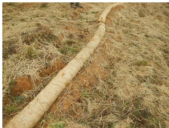
Figure 124. A single wattle is laid around the perimeter of the landing at CAA. Slumps.
