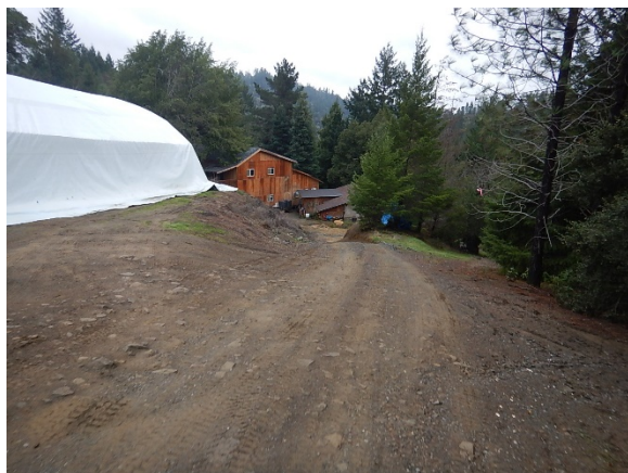
Figure 54. The western road enters the residence area from the north, downslope of CAI and the fuels storage, at the head of the gully.
