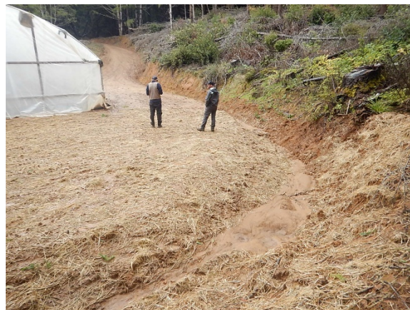
Figure 135. CAC, road drainage comes into area and is transporting sediment in a ditch at edge of cultivation area.
