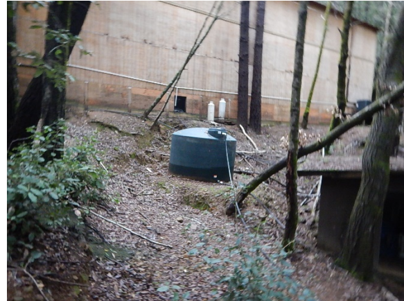
Figure 70. Tank immediately upslope of small building in swale.
