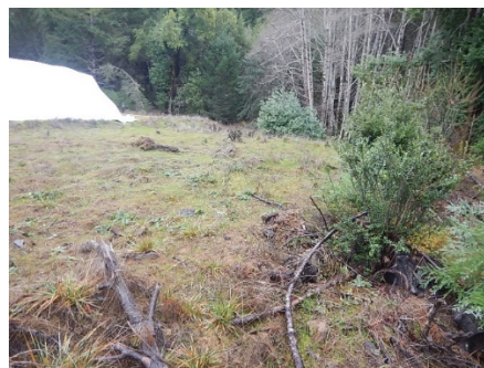
Figure 102. The landing at CAD appears to remain oversteepened in portions.
