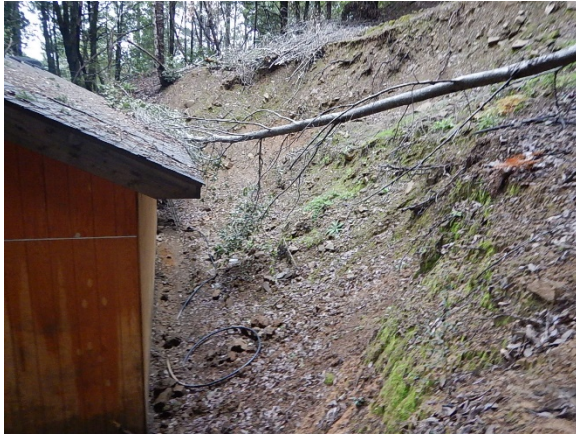
Figure 58. The upper most building at CAH is a generator shed and is built against a cut bank.
