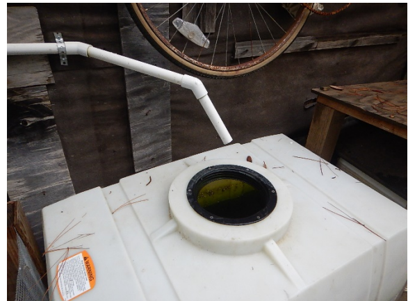
Figure 39. Feed tank at residence.
