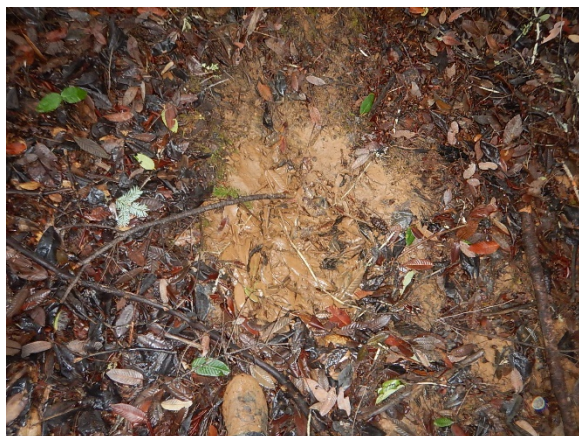
Figure 139. Transported sediment from CAC continues to be fine and mucky well below the source area, where it threatens delivery to the watercourse associated with Site 19.
