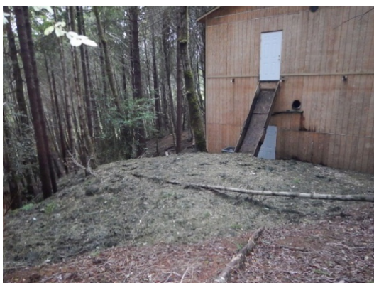
Figure 74. Each of the indoor cultivation buildings has an upstairs door and "chute" that appears to be used to dispose of cultivation waste outside the indoor cultivation buildings.
