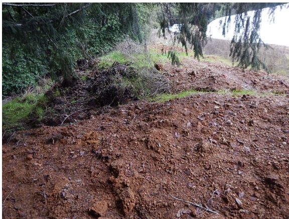
Figure 11. At the south end of the outboard edge of the landing at CAJ, I observed potting soil spoils placed over the edge of the landing, with native earthen material placed on top.
