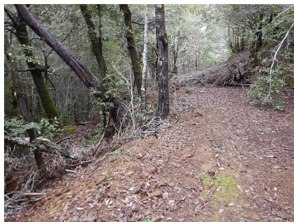
Figure 145. Below CAC, drainage had been diverted down skid road at one point.
