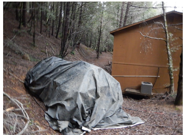
Figure 66. Covered empty fuel storage tank.
