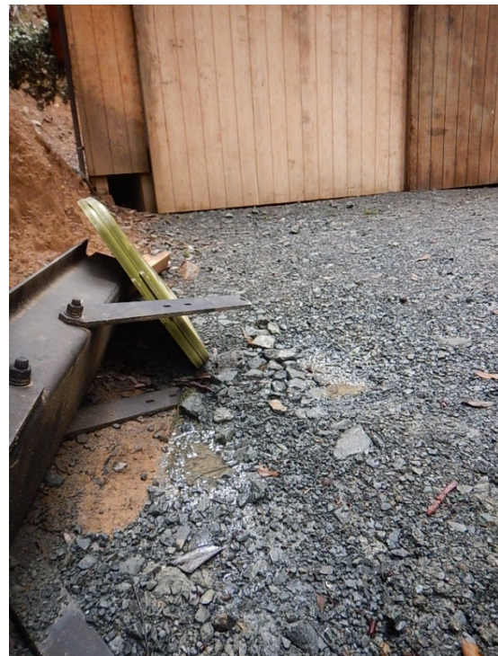
Figure 61. The front of the generator shed has sliding doors that open to an access driveway. This portion of the
