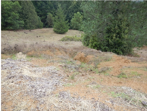
Figure 86. Perlite is transporting through the gully formed in the fill failure at CAH.
