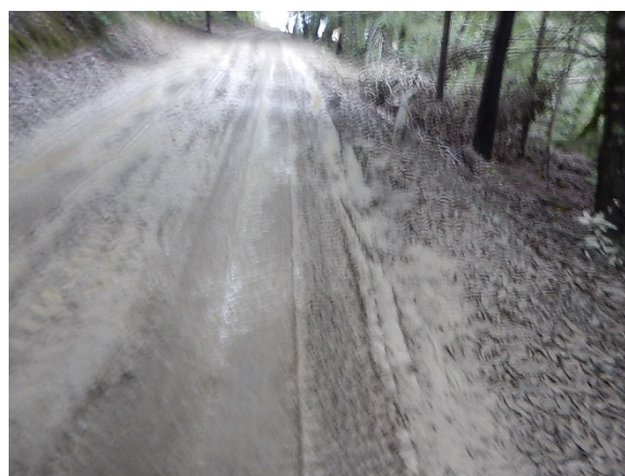
Figure 57. Surface erosion transport.
