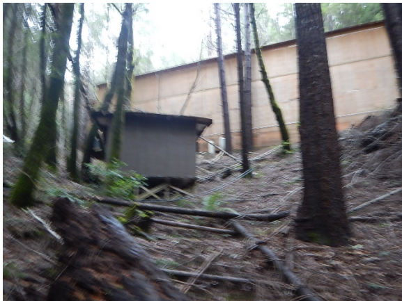
Figure 68. The small building built in the swale of the class III.
