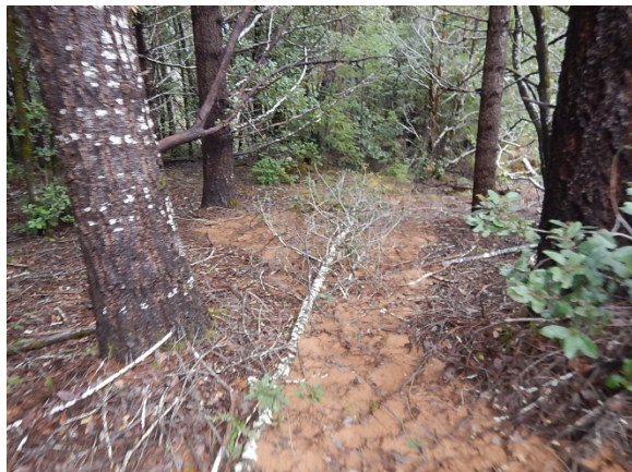
Figure 138. Sediment track from CAC transported from eroded fill slope.
