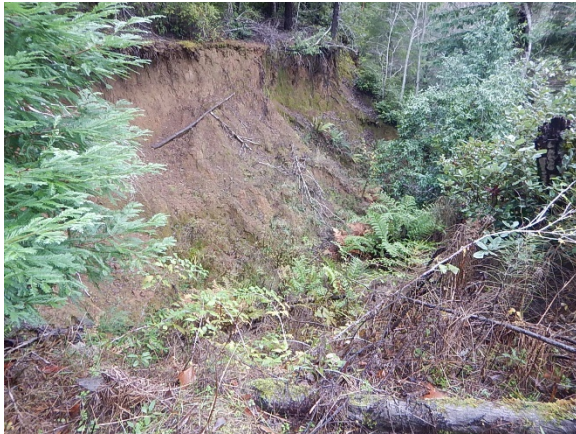
Figure 96. Eroded bank on watercourse adjacent to the landing associated with CAD.
