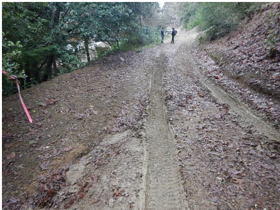
Figure 28. Concentrated road drainage is directed off the road surface via a
