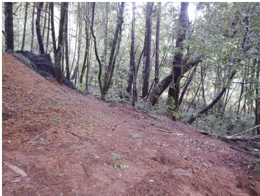
Figure 23 South of CAJ, upslope of the road, cultivation waste is placed on the hillside along with earthen spoils. The spoils are not stabilized. The riparian area along a class III watercourse is comprised of native forest.
