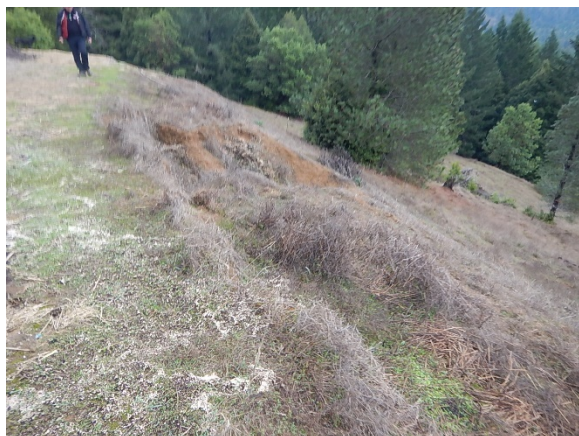
Figure 83. The fill slope at CAG has slumped and eroded. There appears to be no delivery to surface water. Cultivation at CAH has been ceased.
