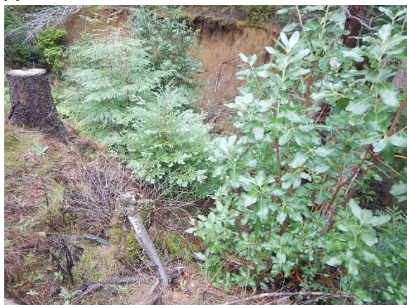
Figure 100. Landing is constructed along a stretch of gullied watercourse.
