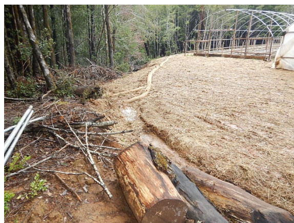
Figure 136. CAC. Straw mulch and a perimeter waddle have been installed.
