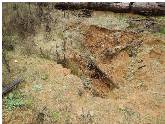
Figure 142. Gully erosion at CAC
