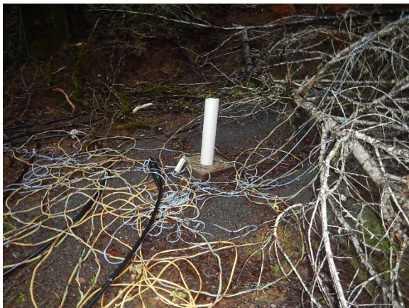
Figure 79. Well head near crossing at site 19.
