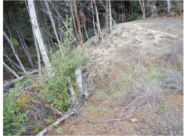
Figure 97. Landing constructed adjacent to watercourse.
