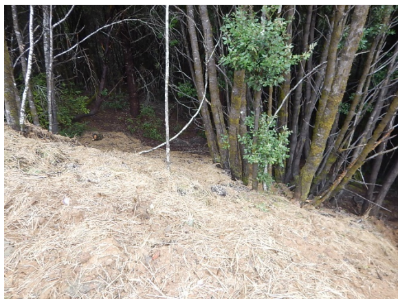
Figure 134. CAB fill pushed into forest.
