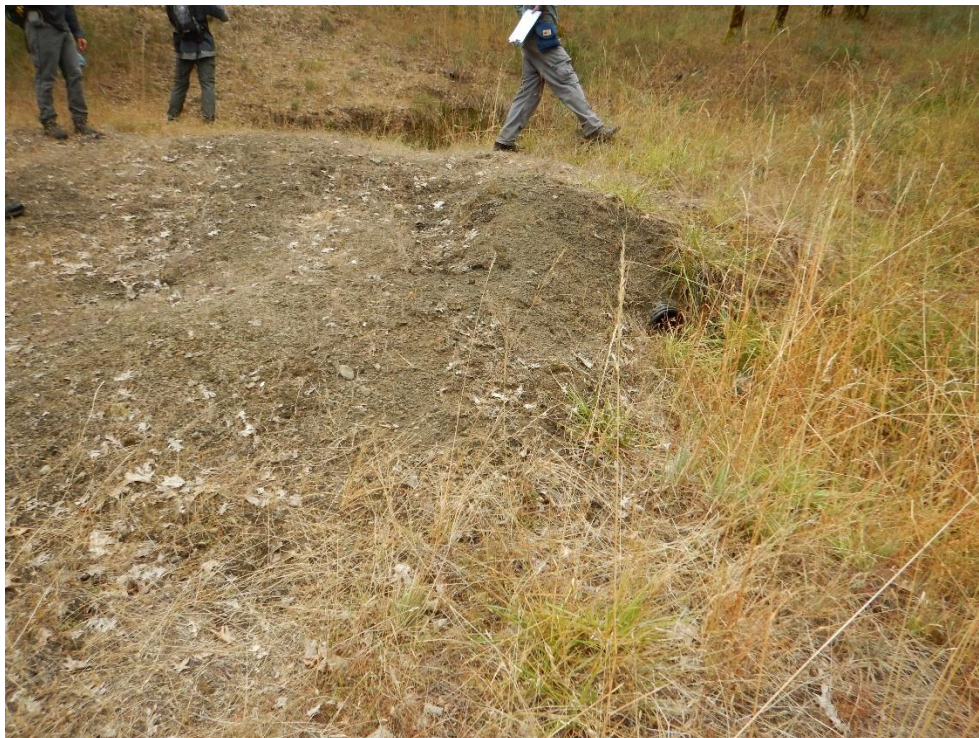
Photo 6— Berm with buried plastic outflow pipe at WQ 3.
