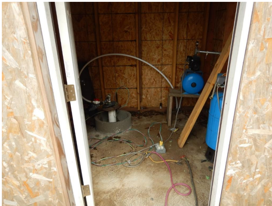
Photo 13—Well house located southeast of WQ 1.
