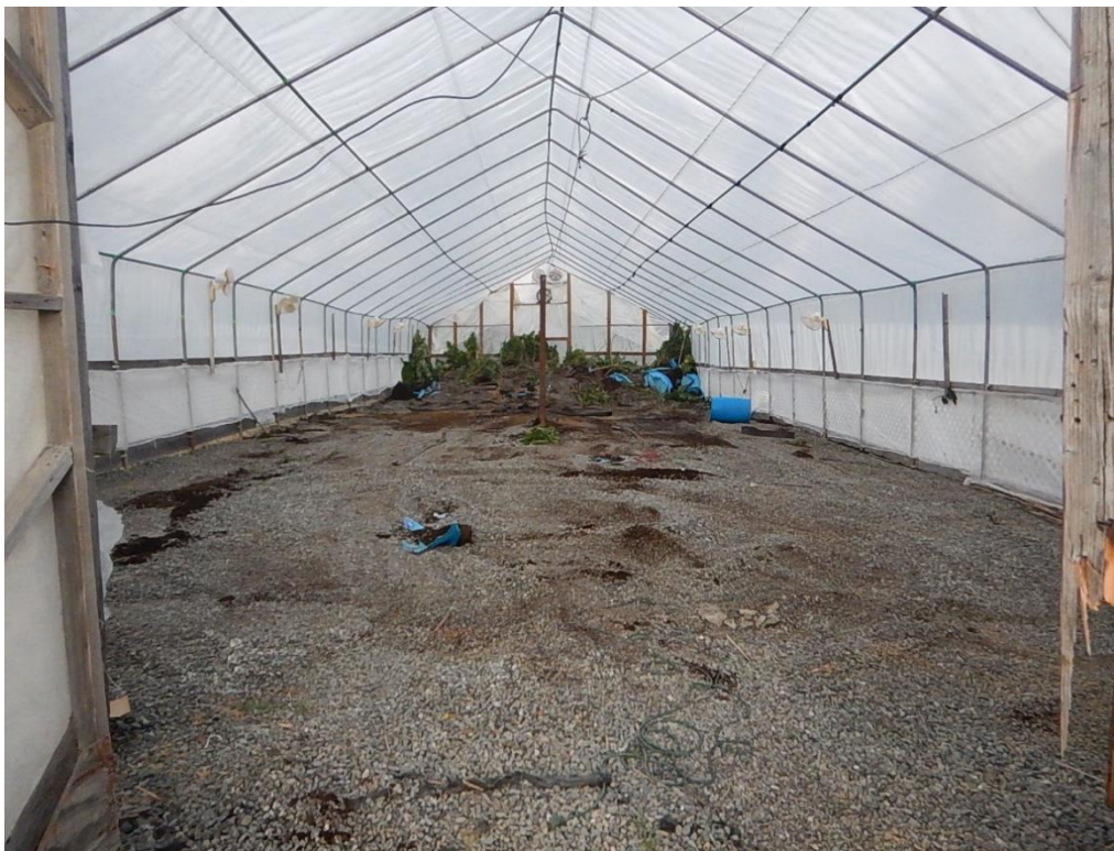
Photo 8, Green house at inspection point GH2
