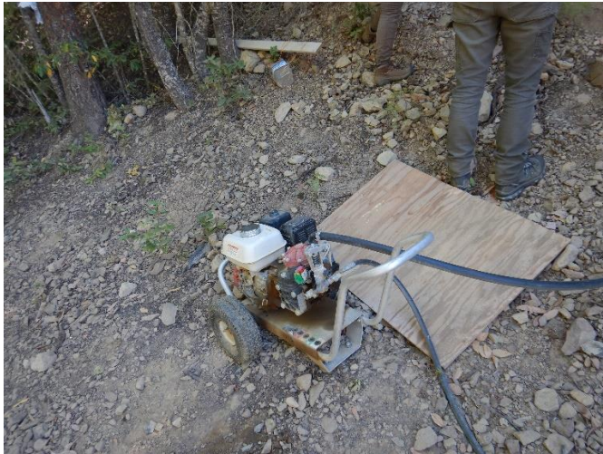
Photo 12, Uncontained pump near inspection point WSTG2
