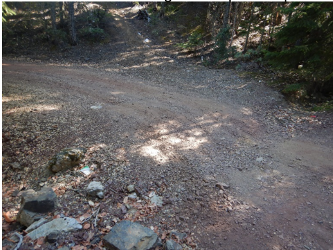
Photo 2 stream crossing 2 at inspection point SC2
