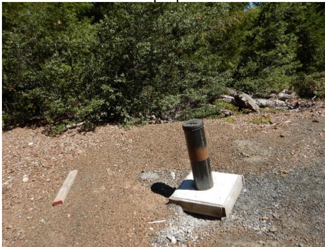
Photo 7, well head at inspection point Well
