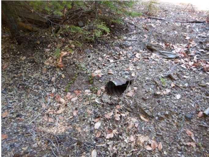
Photo 1 stream crossing 1 at inspection point SC1
