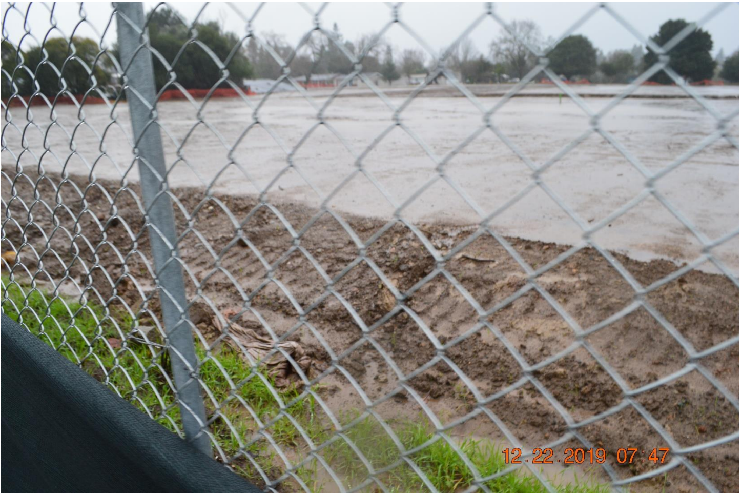
Photo 1: Pad adjacent to Marlow road still has no evidence of effective soil cover. Photo taken by Joshua Luders from public sidewalk.
