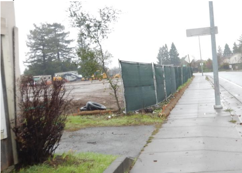
Photo 1: Uncovered disturbed soils sloping towards Marlow Road. Photo taken and edited by Joshua Luders.
