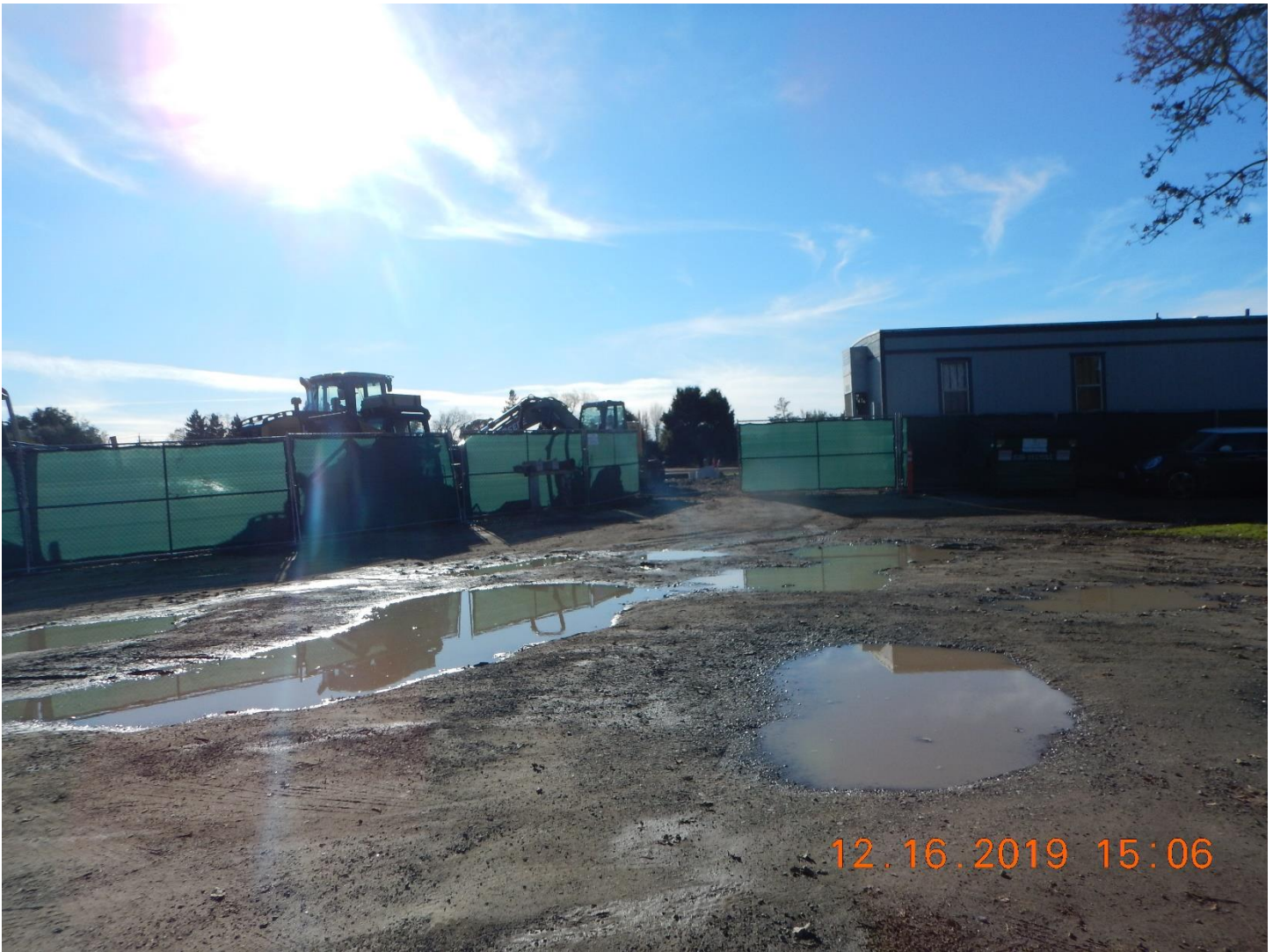
Photo 1: Construction entrance off Marlow Road.
