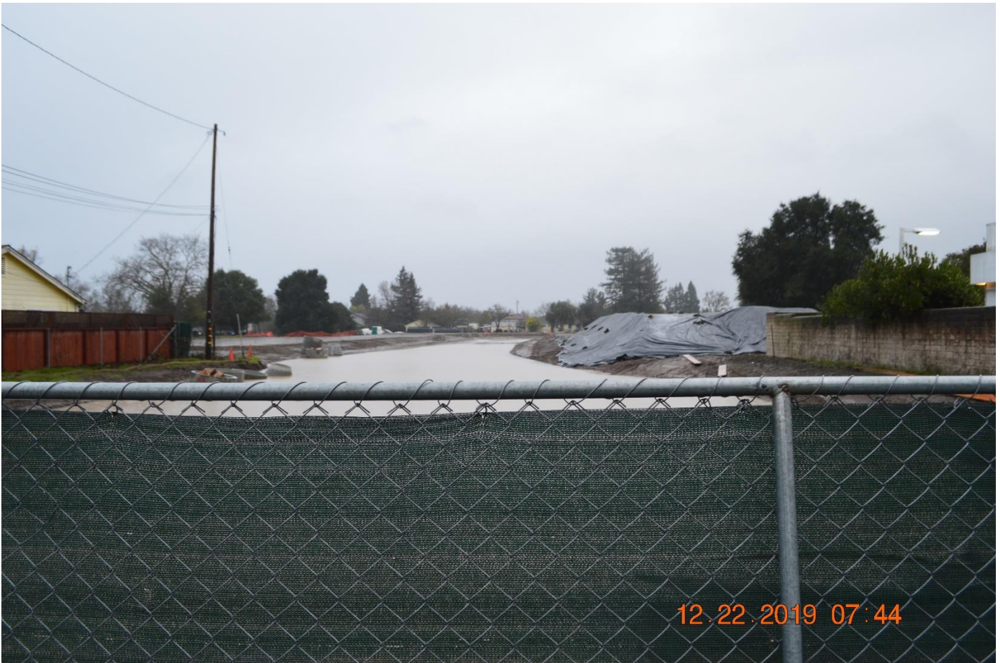
Photo 4: Ponding water extends in the background from Guerneville Road. Exposed soils are on the left and a pile of material is covered on the right. For perspective, a section of the covered pile can be seen from Marlow Road, near the left center of Photo 1. Photo taken by Joshua Luders
