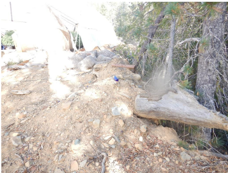
Photo 3—Edge of cut and fill pad in the vicinity of WQ 3.
